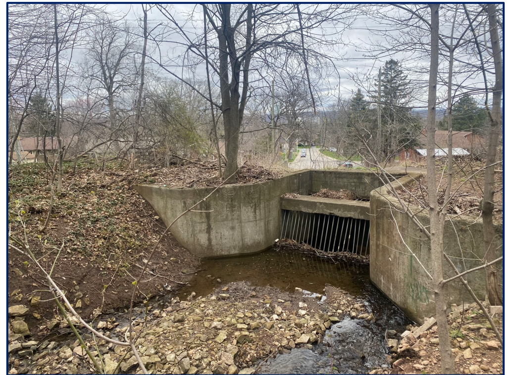
Input 2 Inlet Grate (April 2022)
