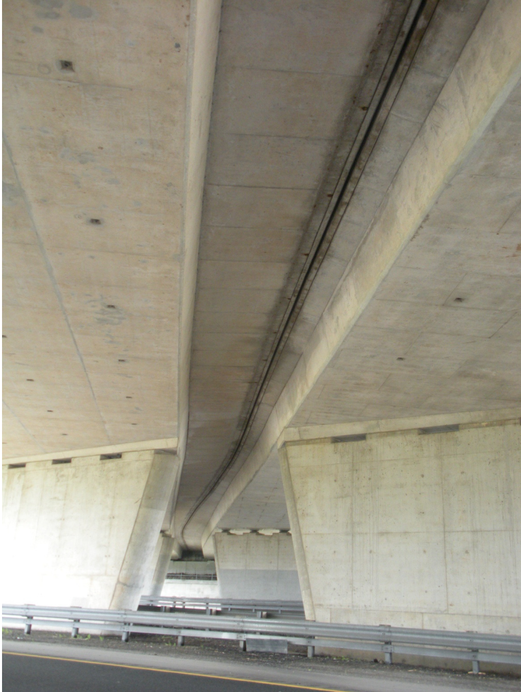
Figure 4 Underside of the Superstructure
