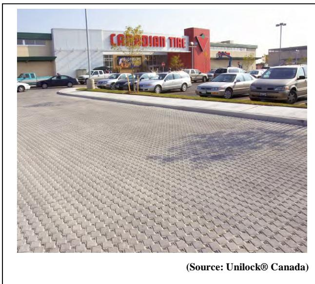
stormwater flows compared to traditional impervious paving surfaces like concrete and asphalt. Assuming the permeable paver is designed with adequate pretreatment and soil infiltration testing, a conservative runoff reduction rate of 90% is assigned to designs that rely upon full infiltration. Other benefits include reduce snow removal costs due to rapid ice melting and drainage, reductions in urban heat island effect (pavers have less thermal conductivity and thermal capacity
