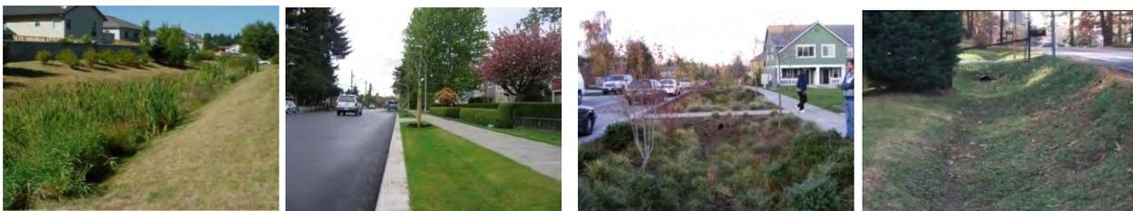
(From L to R: Vegetated Channel, Subsurface Perforated Pipe, Bio-swale & Grass Channel)
