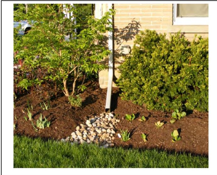
Rooftop disconnection with treatment is possible on lots with any size and configuration; however functional downspout disconnection requires a minimum length of pervious flow path and appropriate soil conditions.
