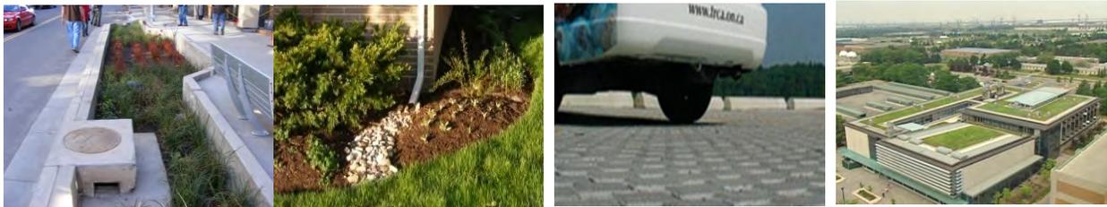
(From L to R: Special Bioretention, Downspout Disconnection, Permeable Pavement & Green Roofs)
