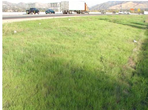
With proper design and maintenance, filter strips can provide relatively high pollutant removal. Research suggests that pollutant concentration levels decrease and that steady state levels can be achieved within five metres of the pavement edge (Lantin and Barrett, 2005). However, maintaining sheet flow is a challenge. Consequently, urban filter strips are often "short circuited" by concentrated flows, which result in little or no treatment of stormwater runoff.
