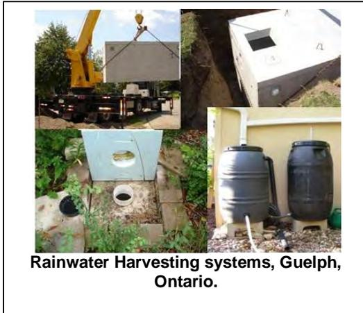
Harvested rainwater that is used for watering landscaping meets the objectives of the water balance requirement, as these flows are infiltrated or evapotranspired after storage. On a larger scale, the reduced demand on the water resources (such as groundwater aquifers and reservoirs) from which municipal water supplies are drawn will add to the water balance benefits of rainwater harvesting. It is estimated that these applications alone can reduce
