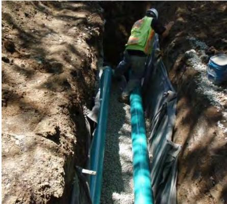
Subsurface perforated pipe systems are essentially a variant/combination of a French drain type Soakaway pit and a conventional storm sewer system. These systems provide efficient conveyance, while encouraging infiltration and groundwater recharge. Perforated pipe systems are linear perforated pipes surrounded by gravel and wrapped in filter cloth, designed to encourage infiltration, thereby reducing runoff volumes, improving water quality and
