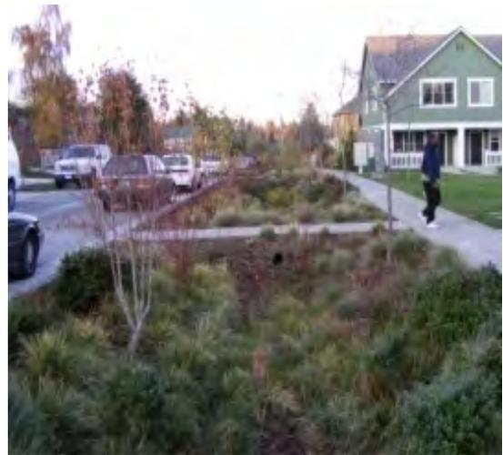
If properly designed and maintained, dry swales can provide stormwater treatment while accenting the natural landscape and providing improved site aesthetics. Dry swales can be implemented on a variety of development sites where density and topography permit their application. The linear nature of swales makes them well-suited to treat roadway or commercial/industrial runoff. Dry swales can also be used in or alongside parking lots in various configurations.
