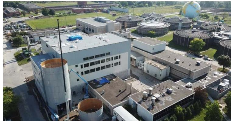
Interior architectural finishing's are progressing quickly, with flooring placed and ceilings finished. The odour control system is being installed, ductwork is being constructed, and remaining exterior works such as paving have started.
