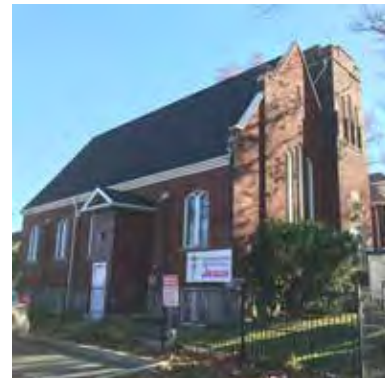
North and West elevation - 15 Wexford Avenue (ERA, 2022)
