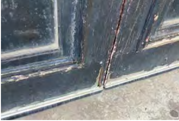
Fig. 89. Paint deterioration.
