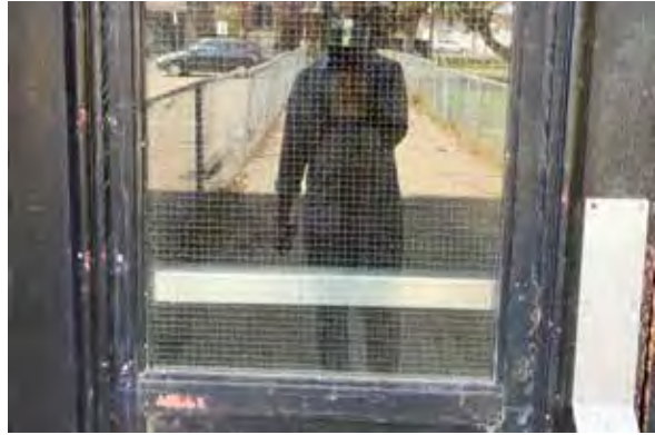
Fig. 87. Wired safety glass panel infill.
