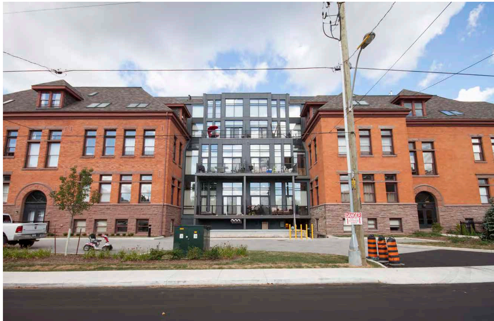
Precedent - Existing masonry building with contemporary infill - Stinson School Lofts (ICON Architects)
