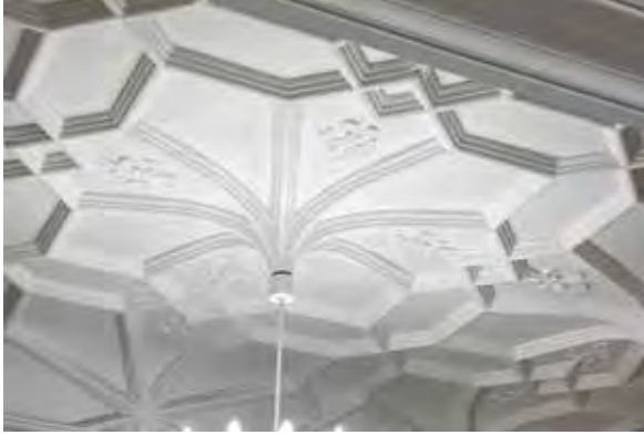
Fig. 94. Main lobby plaster ceiling.
