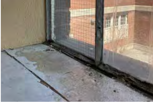
Fig. 57. Overpainting of steel frames.
