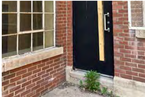
Fig. 43. Cast in place concrete base wall.
