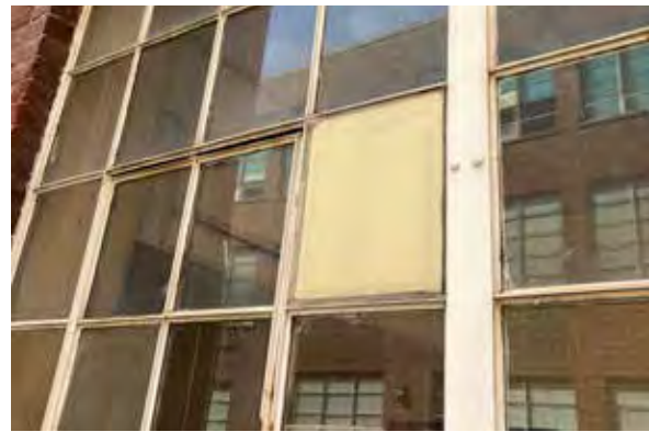
Fig. 55. Infilled window lite.
