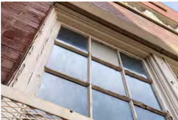
Fig. 54. Large cracks at base of pilasters.
