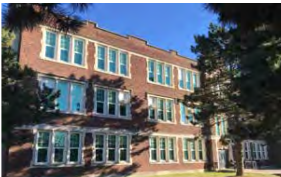
1924 School Building, west elevation.
