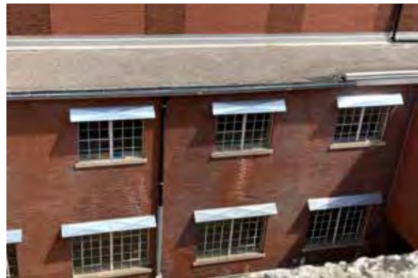
Fig. 50. Added flashings over first floor windows.
