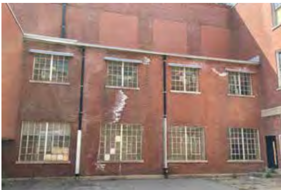
Fig. 46. Brick infill of pre-existing clerestory.
