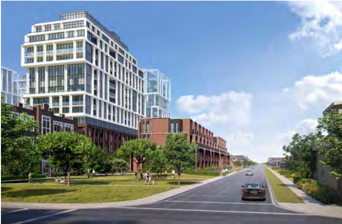
Looking south along Graham Avenue South from Main Street East (Graziani & Corazza Architects Inc., 2022).
