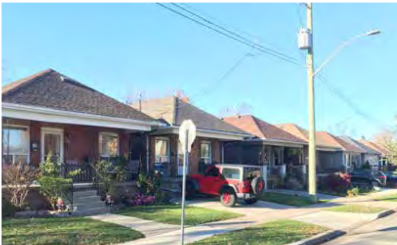
Looking northwest from the corner of Graham Avenue and Maple Avenue (ERA, 2022).
