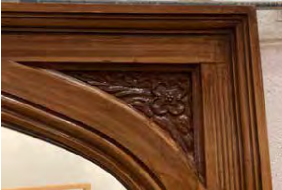
Fig. 101. Auditorium door surround detail.
