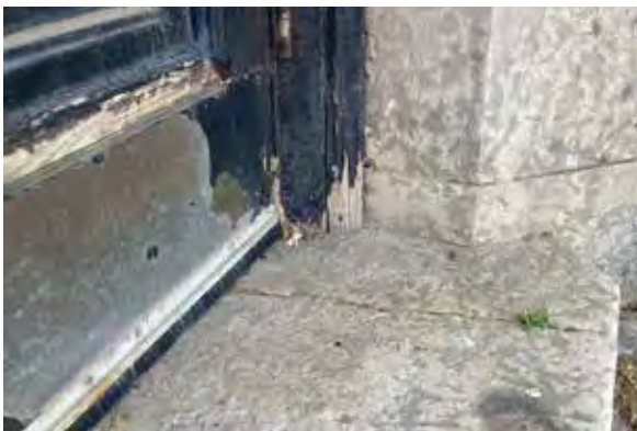
Fig. 91. Paint deterioration.
