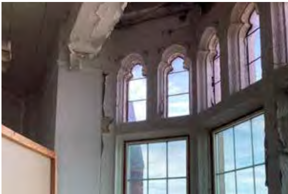
Fig. 41. Trefoil arched openings with original glazing.
