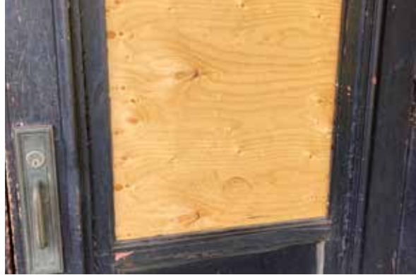
Fig. 86. Plywood pane infill.
