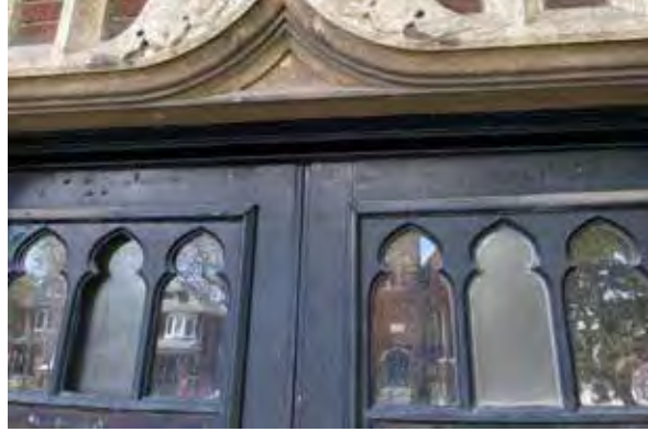
Fig. 85. Replaced transom lites.
