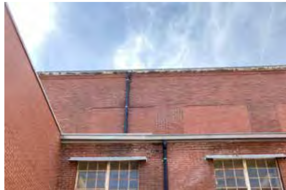
Fig. 49. Added flashings over first floor windows.
