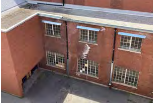
Fig. 51. Added flashings and PVC downspout.
