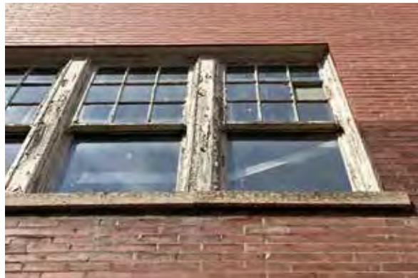
Fig. 44. Cast stone window sills.
