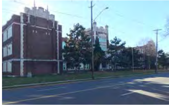
1924 School Building, north elevation.
