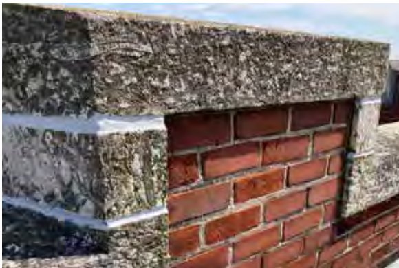
Fig. 64. Replaced mortar joint.
