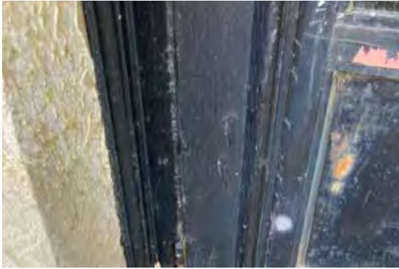
Fig. 90. Paint deterioration.
