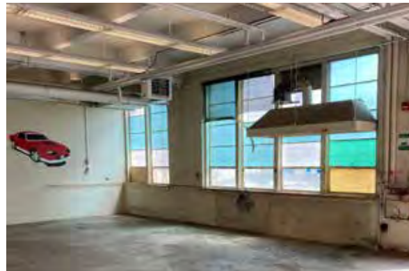
Fig. 115. Infilled window panes.
