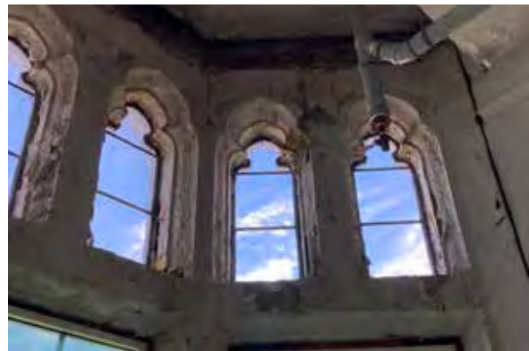
Fig. 113. Original trefoil glazed openings.
