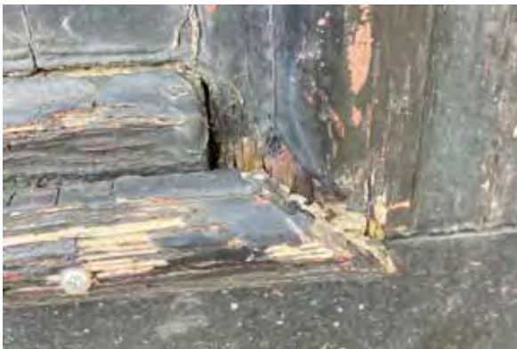
Fig. 92. Separated moulding attached via screw.
