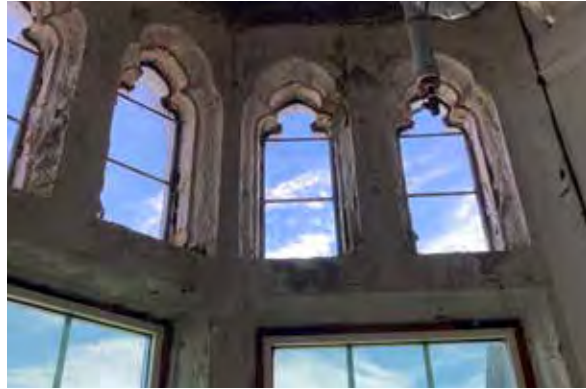
Fig. 42. Trefoil arched openings with original glazing.
