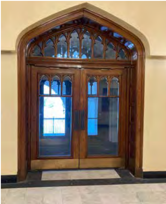
Interior front entrance vestibule doorway.
