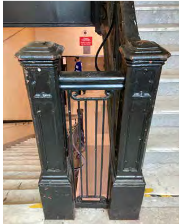
Stairway landing newel posts.
