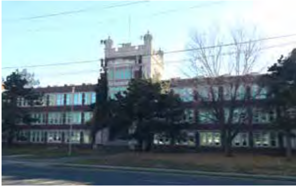
North elevation, 1924 School Building.
