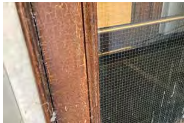
Fig. 80. Crazing of wood coating.
