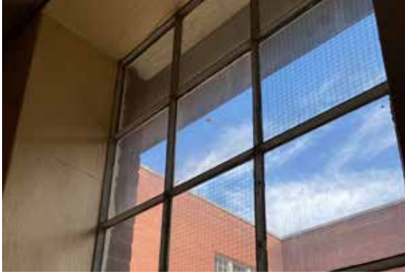
Fig. 56. Replaced window lites.
