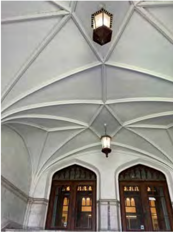
Front entrance and doorways.
