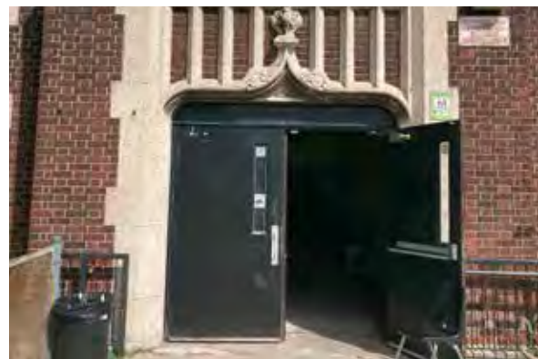
Fig. 93. Replaced double doors.
