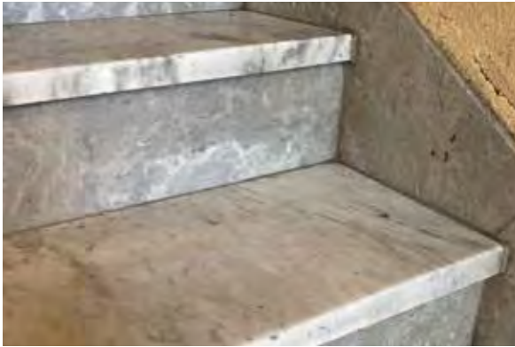
Fig. 107. Original marble stairs in good condition.
