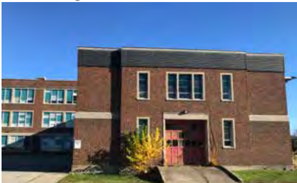
West elevation - 1948-50 Southwest Wing (left) and 1948-50 South Centre Wing (right).
