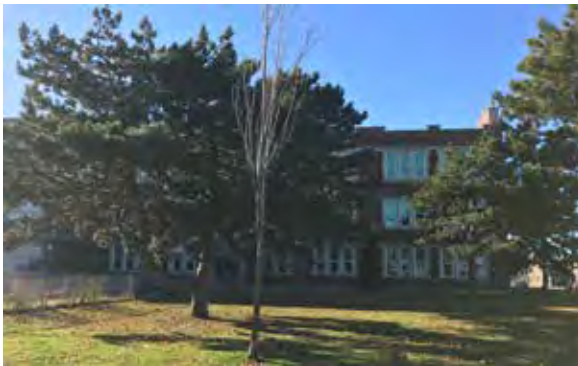
1924 School Building, east elevation.
