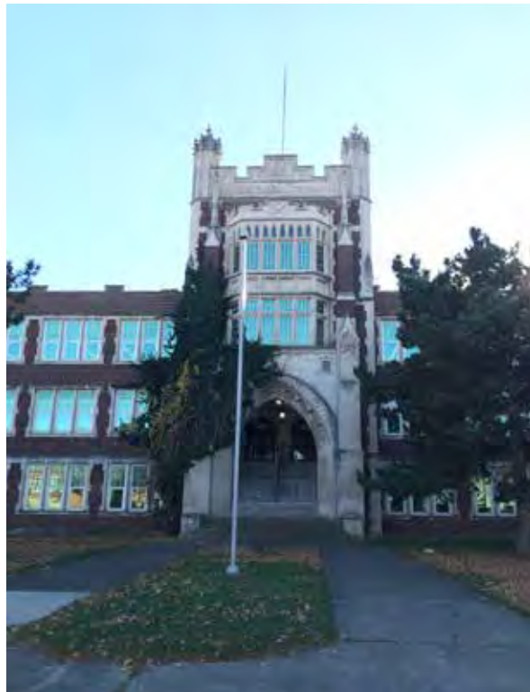
1924 School Building, north elevation tower.
