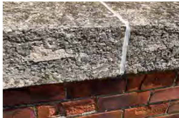
Fig. 62. Replaced mortar joint.
