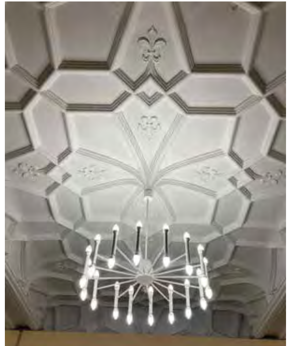
Front entrance lobby plaster ceiling.
