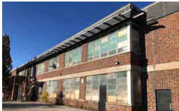
South elevation - 1948-50 South Wing.
