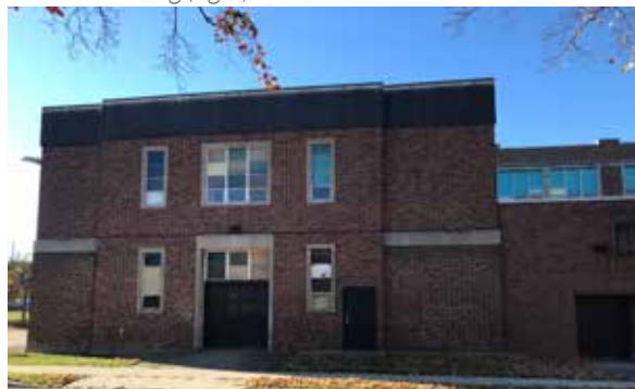
East elevation - 1948-50 South Centre Wing (left) and 1970 plumbing shop addition (right).
