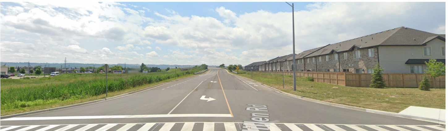
View towards the South on Millen Road
