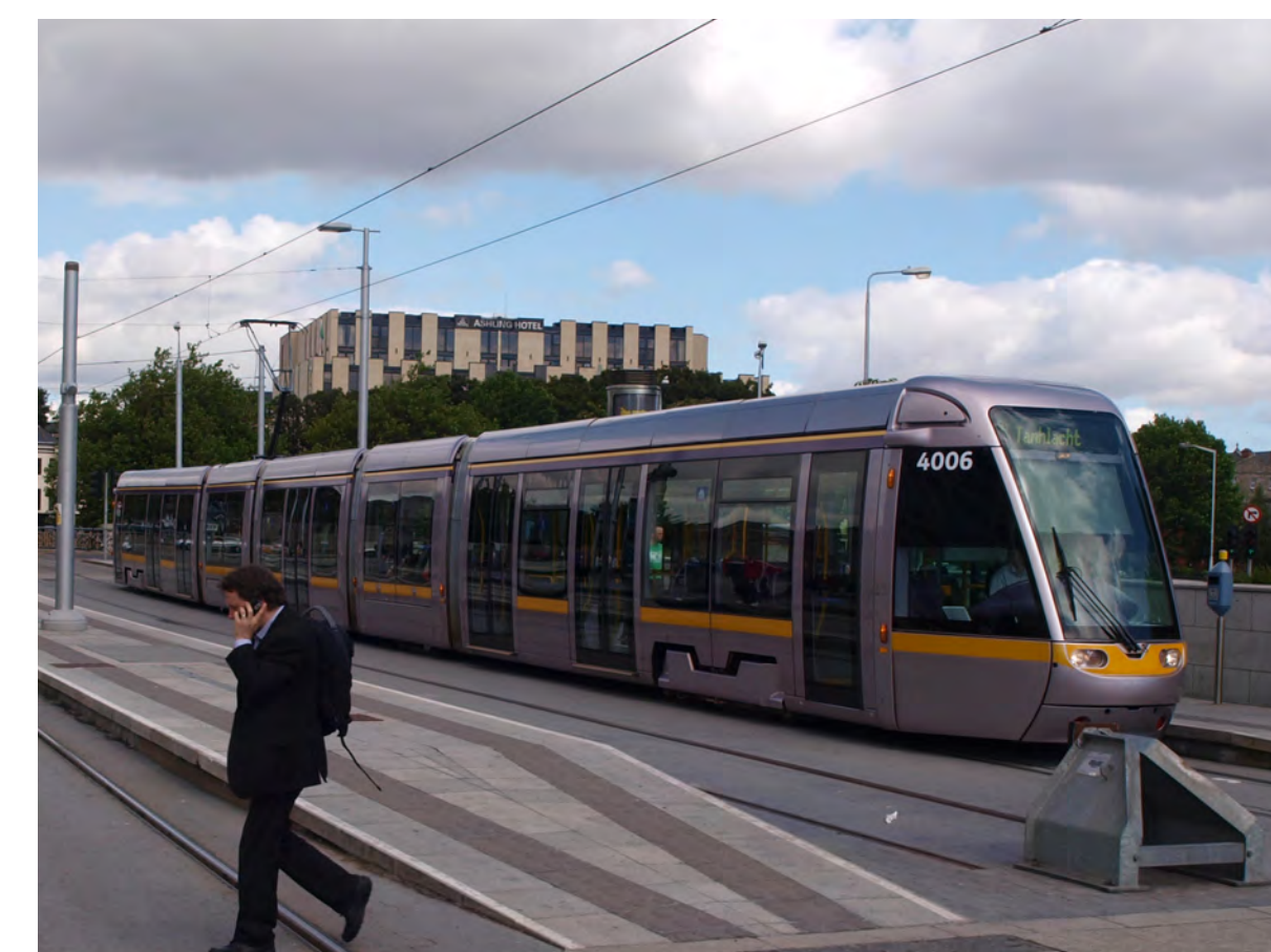
↑ Side-pole system at off-street stop in Dublin with platform lighting combined on OCS poles
