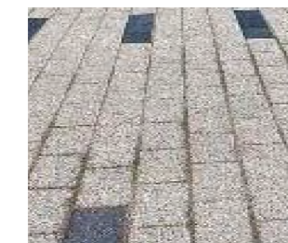
↑ Concrete unit paving
