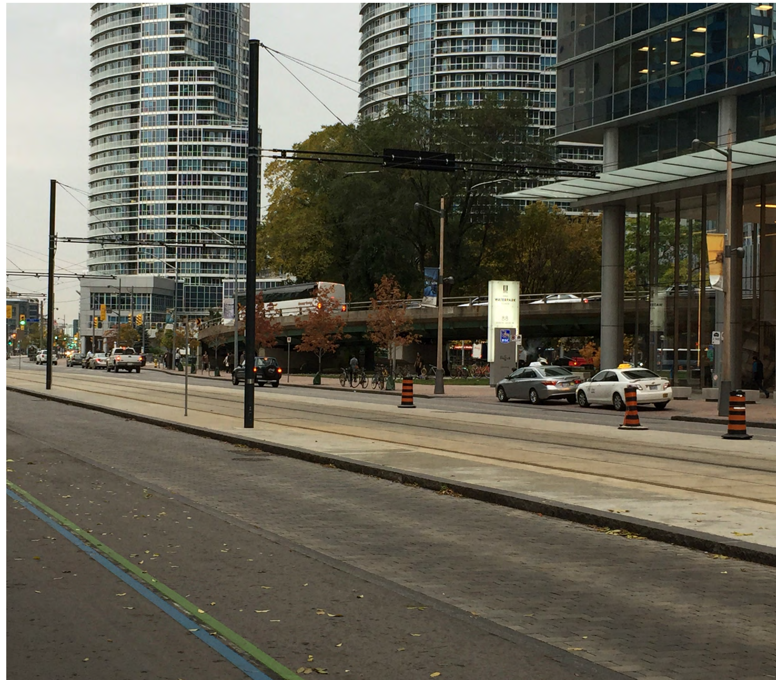
↑ OCS poles on Queen's Quay in Toronto
