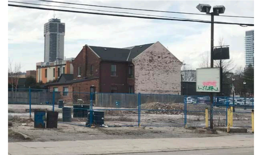
North elevation of 136 Ferguson Avenue North (ERA, 2024).
