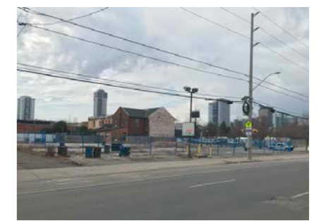
View southwest along Cannon St. East towards the Site (ERA, 2024).
