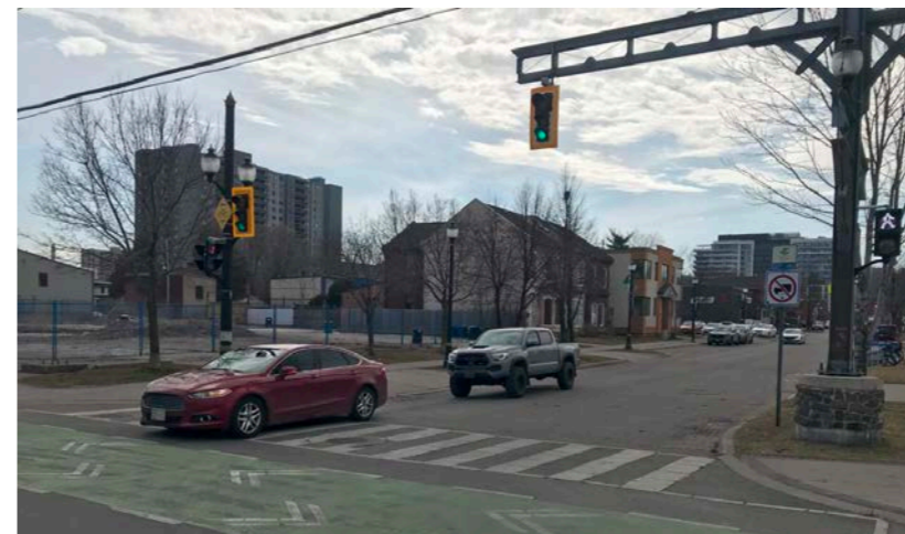
View southeast towards the Site on Ferguson Avenue North at Cannon Street East (ERA, 2024).
