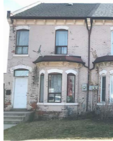
From left to right: 136 Ferguson Avenue North (ERA, 2024).
