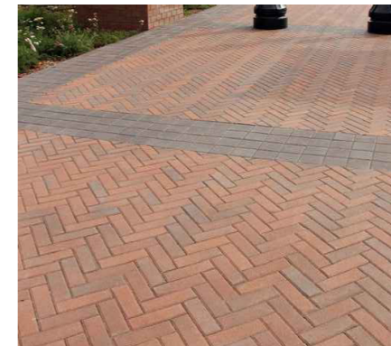
Heritage paving pattern and colour
