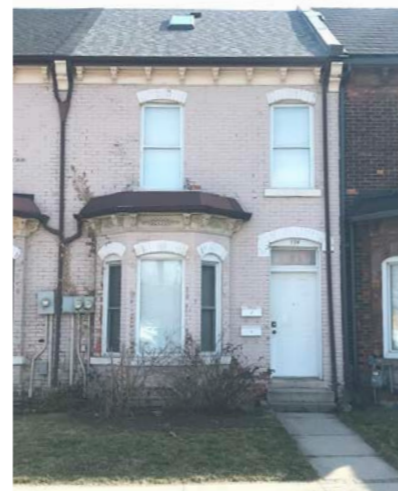
From left to right: 134 Ferguson Avenue North (ERA, 2024).
