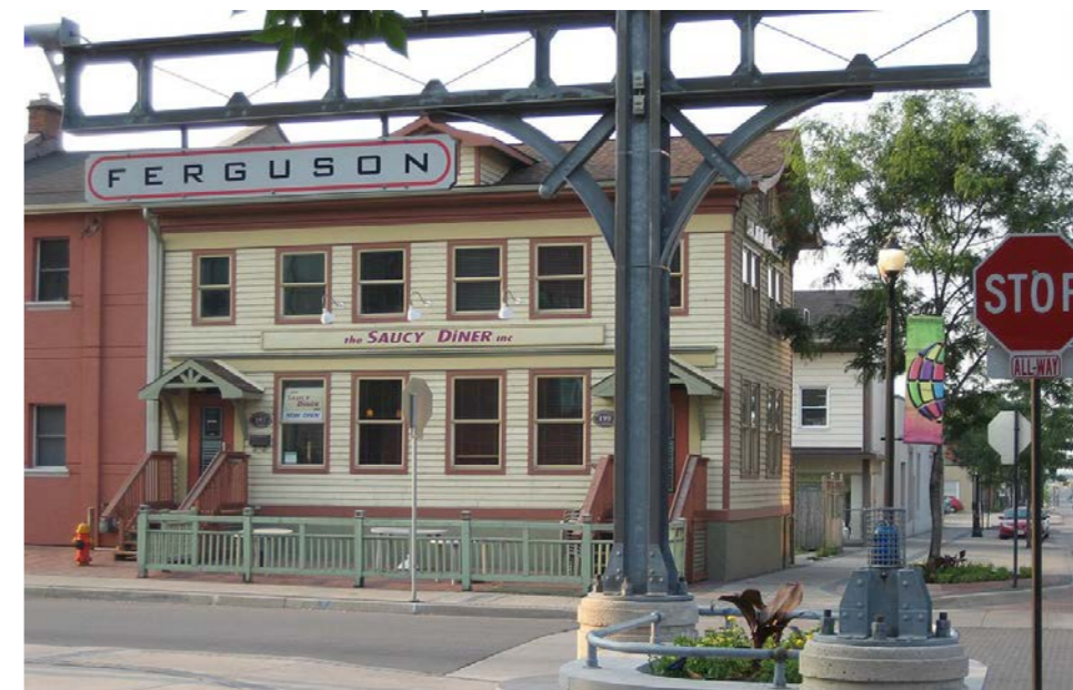
Fig 10. Ferguson Avenue Crossing Gates
