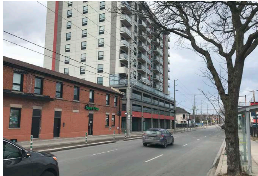
View west on Cannon Street East near the tower development at 220 Cannon Street East (ERA, 2024).
