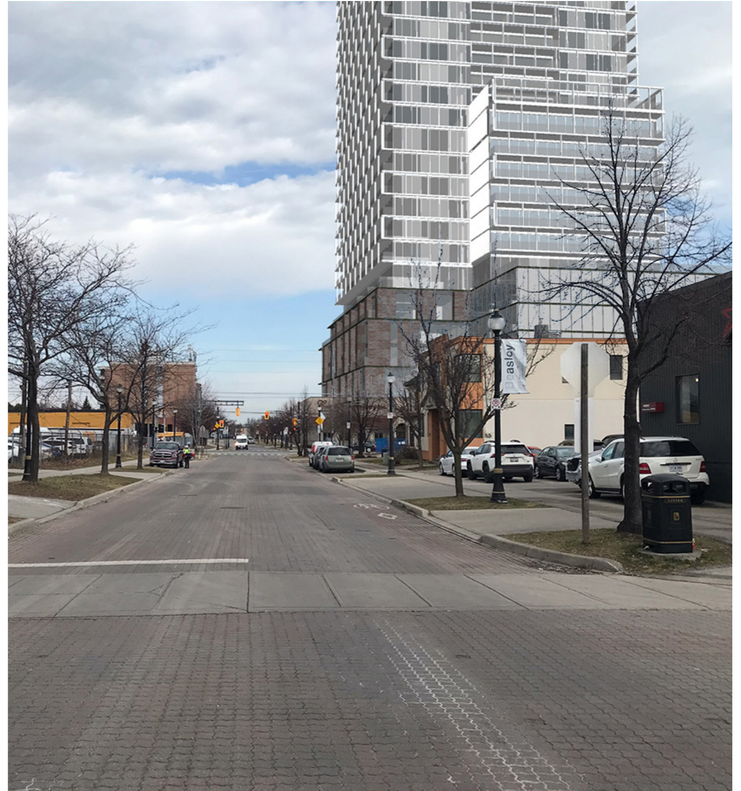
After: Looking North on Ferguson Avenue North
