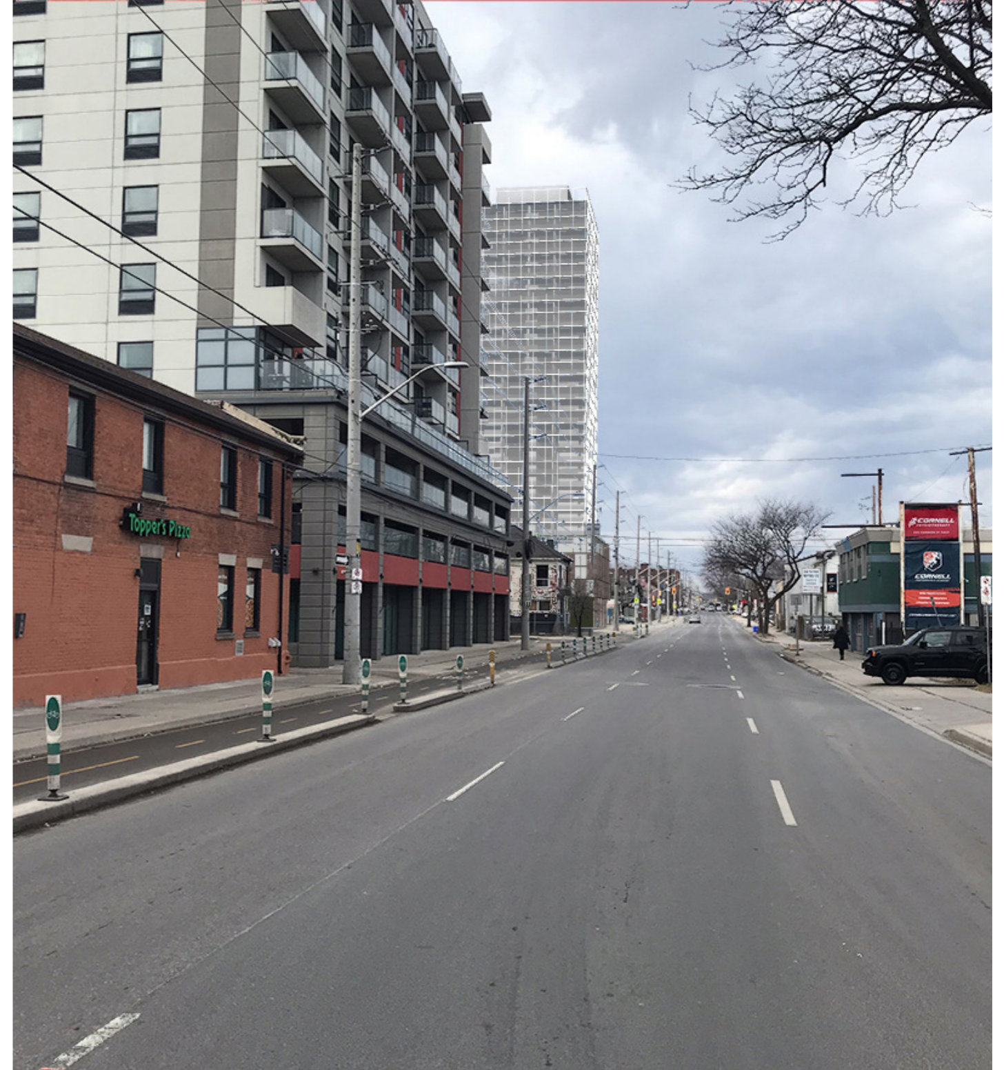
After: Looking West on Cannon Street East
