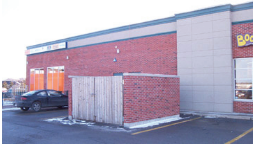
Waste storage enclosure of brick and wood similar to adjacent commercial building
