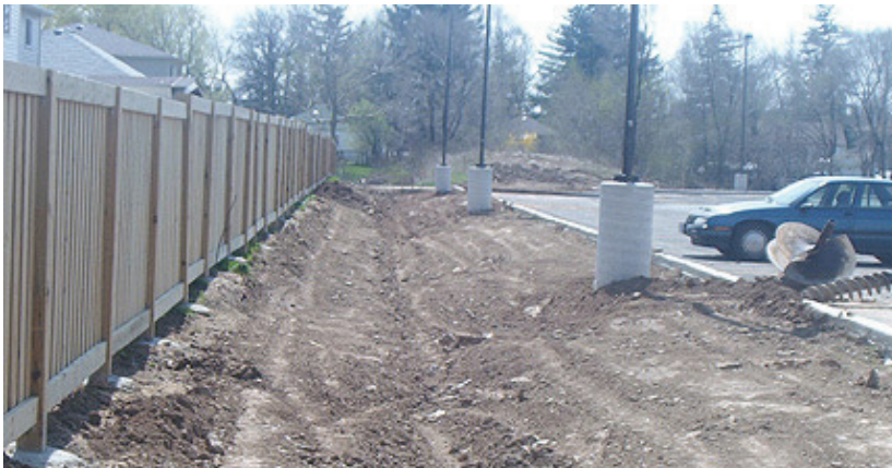
Commercial property graded to drain away from adjacent development, shown during construction (above) and with landscaping installed (below)
