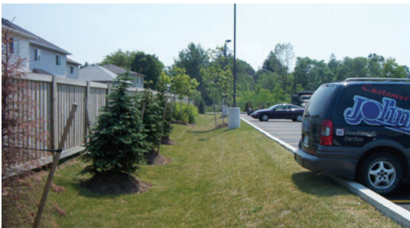
Commercial property graded to drain away from adjacent development, shown during construction (above) and with landscaping installed (below)
