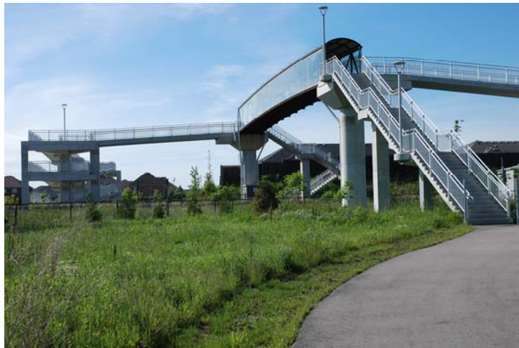
Figure B -View of track crossing – glass panels. Remaining pedestrian circulation areas indicate railings, OMC Photo
