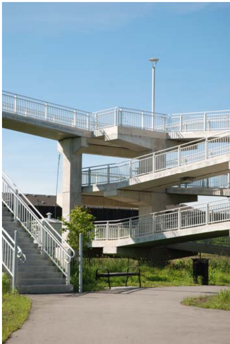
Figure A - View of bridge entrance with accessible ramps and rest stop at base, OMC Photo
