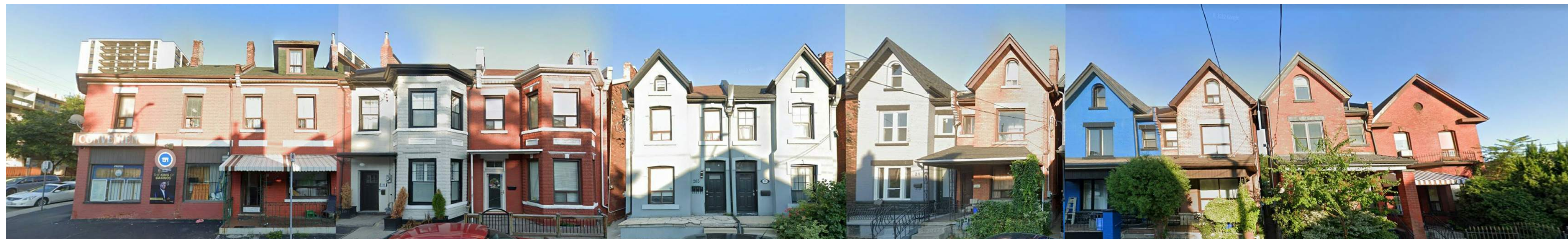
STREETSCAPE VIEW ALONG JOHN STREET TO THE NORTH OF 75 JOHN
