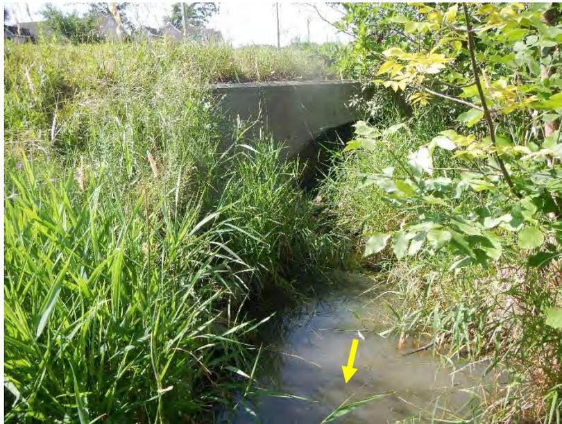
The crossing at Barton Street was a circular concrete culvert which had been partially blocked by riparian vegetation which had colonized the channel.
