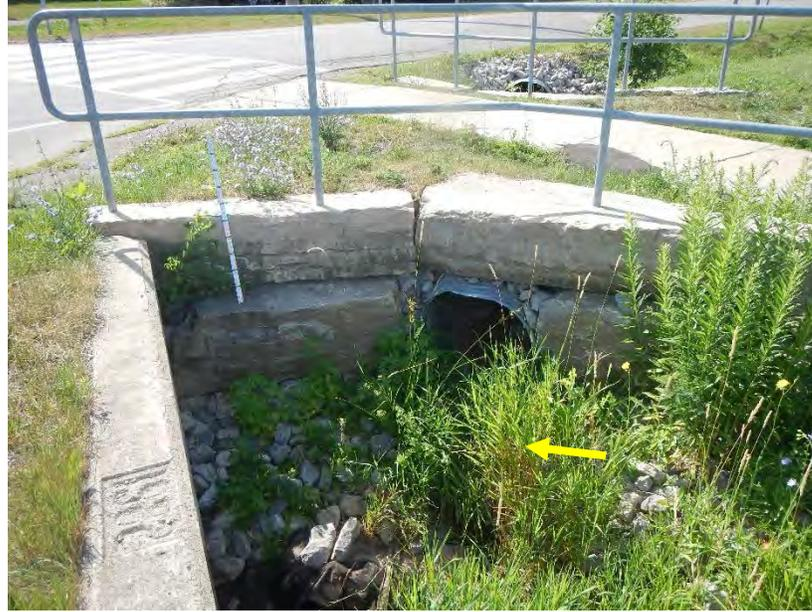
At the downstream extent of Reach 3, a culvert conveying flow from the west side of Lewis Road and a small ditch from the north formed a confluence.
