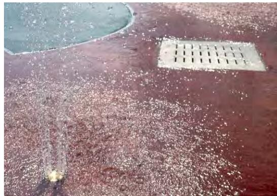
Provide min. 1.0m concrete apron with 50mm rise on down slope side to contain and direct water to drain. Sheet drain to catch basin with slotted cover.
