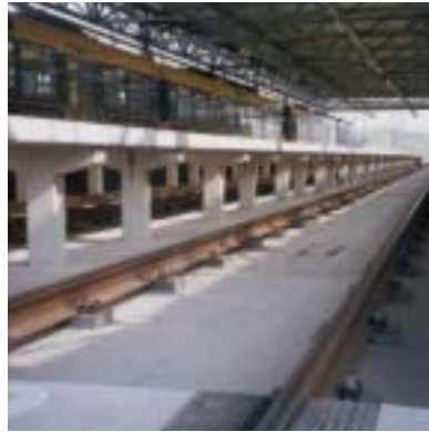
Remseck/Germany; LRV depot of SSB. Steel baseplates (360 x 210 mm) fixed with Icosit® KC 340 adhesive without anchor bolts – an extremely cost-efficient design.
