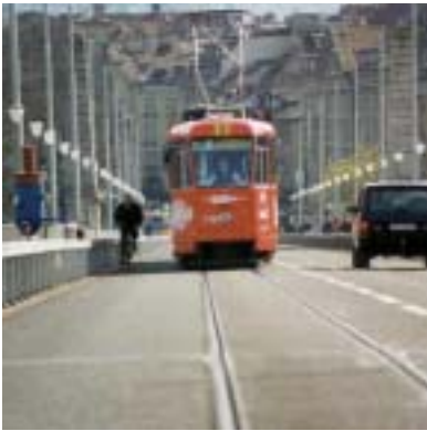
Bern/Switzerland; Kornhaus bridge. The embedded (Ri51) rail design with Icosit® KC 340 permitted lower construction height and a considerable reduction of the deadweight of this historic bridge
