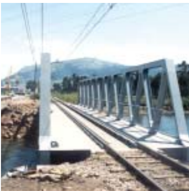
La Pereda/Spain; F.E.R.V.E. railway bridge. As the UIC 54 rail floats in Icosit® KC, noise emissions were drastically reduced.
