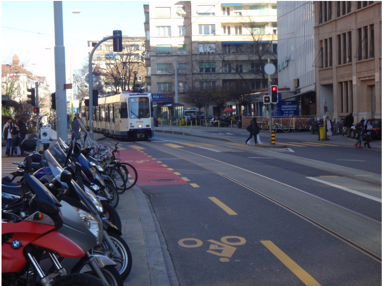
Figure 2-2 - Example of Embedded Track - Geneva Switzerland
