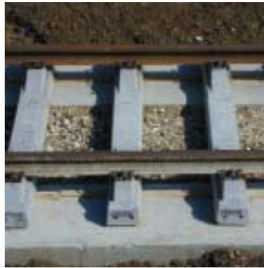
Stuttgart/Germany. Detail of "Bremen" type lawn track before undersealing of sleepers/ ties.
