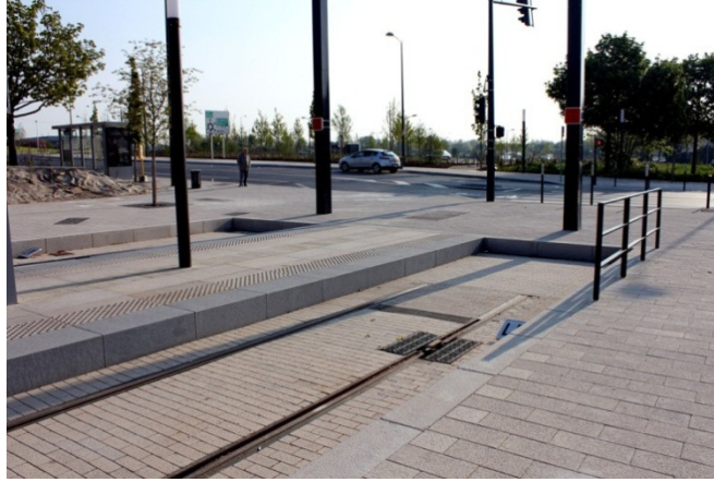
Figure 2-9 - Rail Arrestor System - Reims Tramway, France
