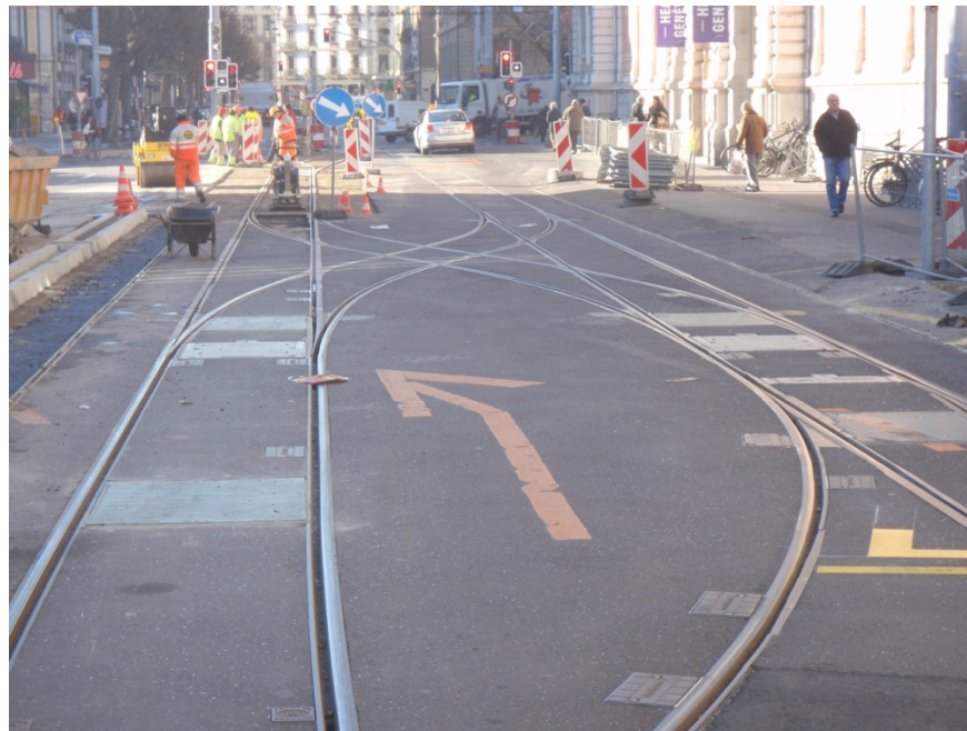
Figure 2-6 - Typical Embedded Special Trackwork - Geneva Tram – Switzerland
