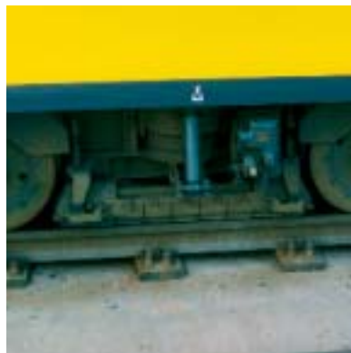
Berlin/Germany. Discrete fixation with baseplates 360 x 210 mm
