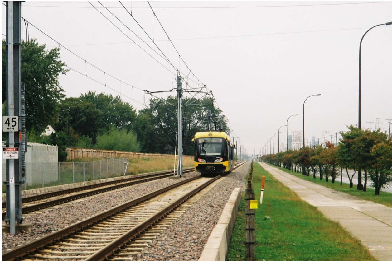
Figure 2-3 - Example of Ballasted Track - Minneapolis LRT, USA
