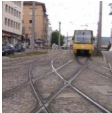
Stuttgart, Germany, Berliner Platz (rail junction, Ri60 continuously undersealed)
