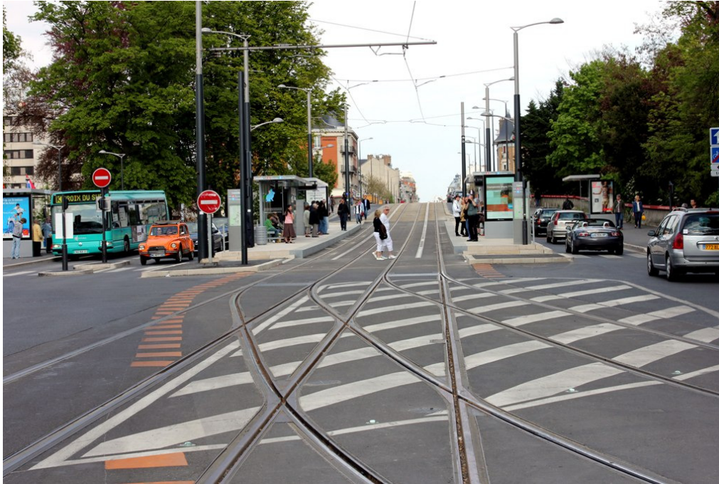
Figure 2-7 - Embedded Special Turnouts - Reims, France
