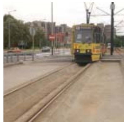
Cracow/Poland, Izidora-Stelli-Sawickiego bridge. Ri60 rail continuously embedded in Icosit® KC 340/45
