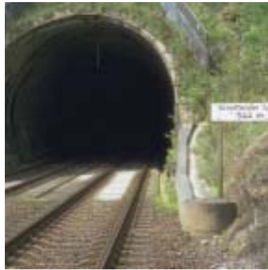
Mosbach/Germany; Schefflenzer railway tunnel. Discrete fixation (loarb 199) on slabtrack after removal of ballast to increase clearance.
