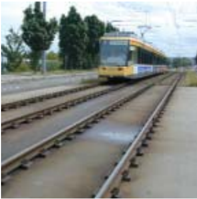
Karlsruhe/Germany, Siemens Allee bridge. Rph1 baseplates (345 x 210 mm) fixed with Icosit® KC adhesive grout without any anchor bolts.
