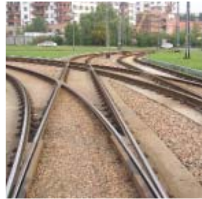
Cracow/Poland. Discrete fixation with Icosit® KC 340/4 Polyurethane grout on slabtrack.
