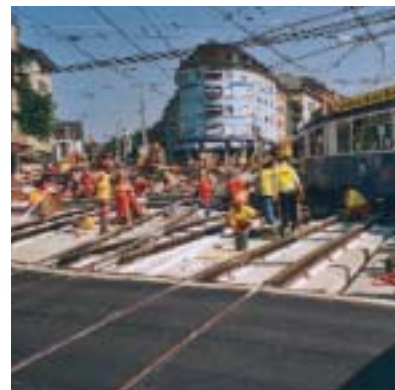
Zurich/Switzerland, Schaffhauser Platz, continuously undersealed Ri60 rail
