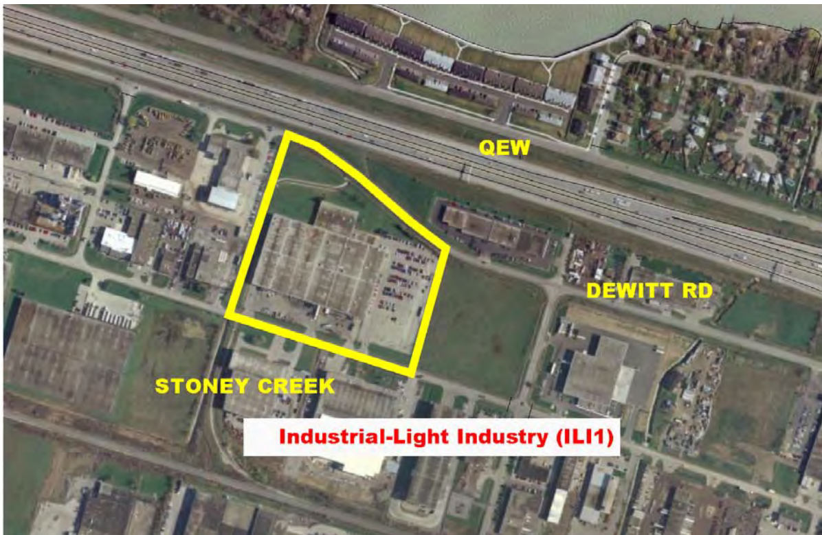
Figure 5.11: Standard Industrial Property – Stoney Creek (ILI1), indicates that the industrial building, parking lot and grass area are the main components for this sub-catchment area.
