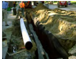
Perforated Pipe (during construction) used to promote infiltration
