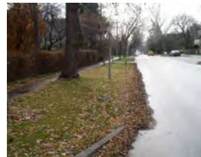
Perforated Pipe (underground)
