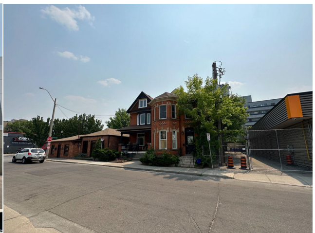
Figure 2.4: South view from southwest corner of subject lands.
