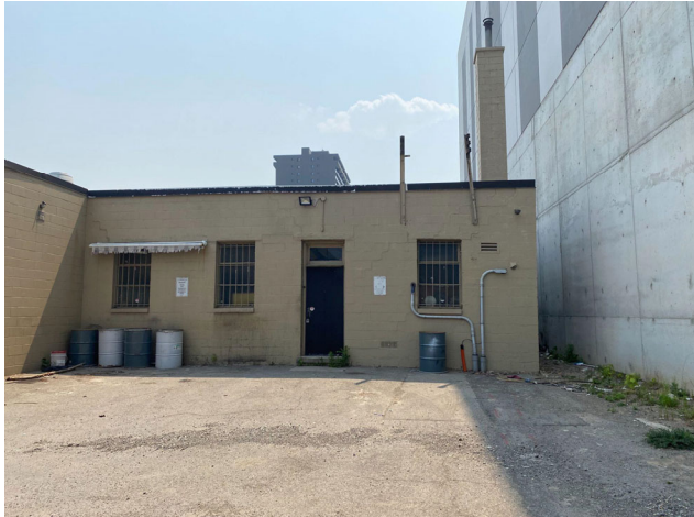
Figure 4.1: South View of northwest side of subject lands.
