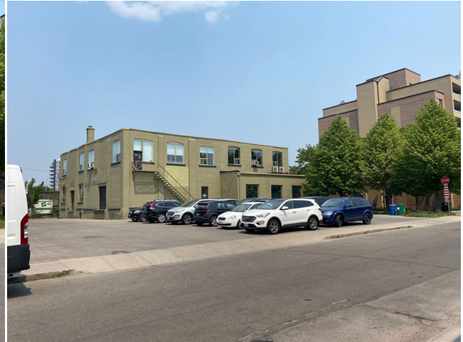
Figure 2.2: Northeast view of subject lands from Jackson St. E.
