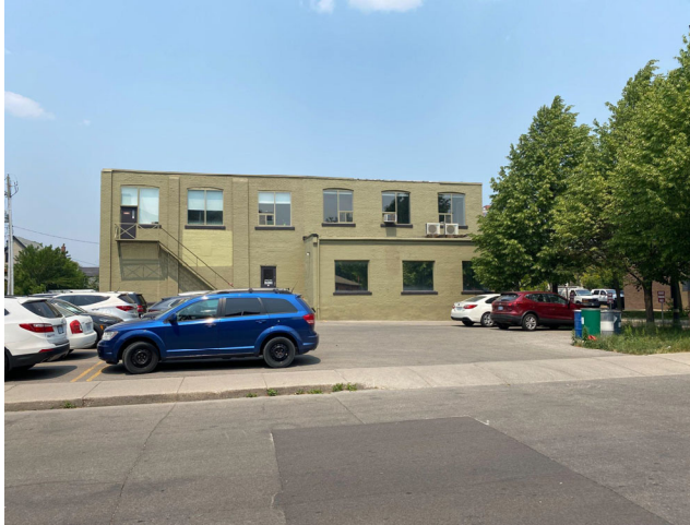
Figure 2.1: North view of subject lands from Jackson St. E.
