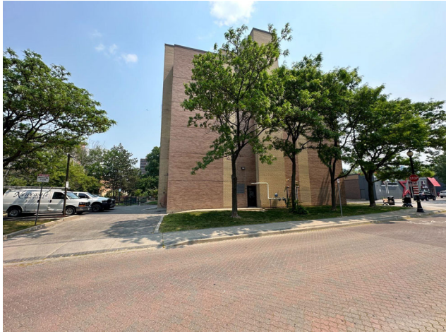
Figure 6.1: Southeast view from northeast corner of subject lands.
