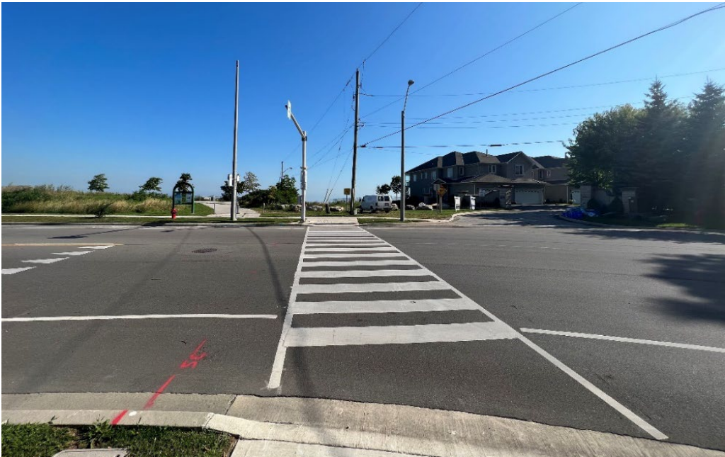
View of crosswalk connecting to the paved multi-use trail, looking north
