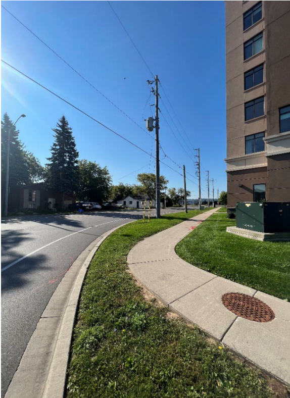
View of Subject Lands from intersection of Shoreview Place & Millen Road looking Southeast
