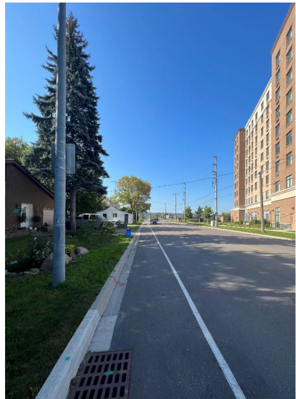
View along Subject Lands frontage along Millen Road looking southeast
