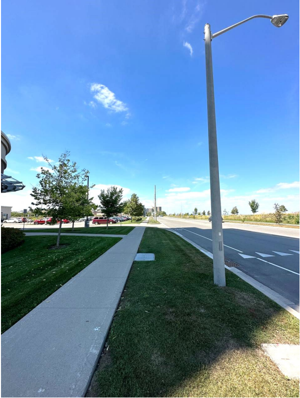
View of existing sidewalk and bike lane on Shoreview Place (right) looking Northwest
