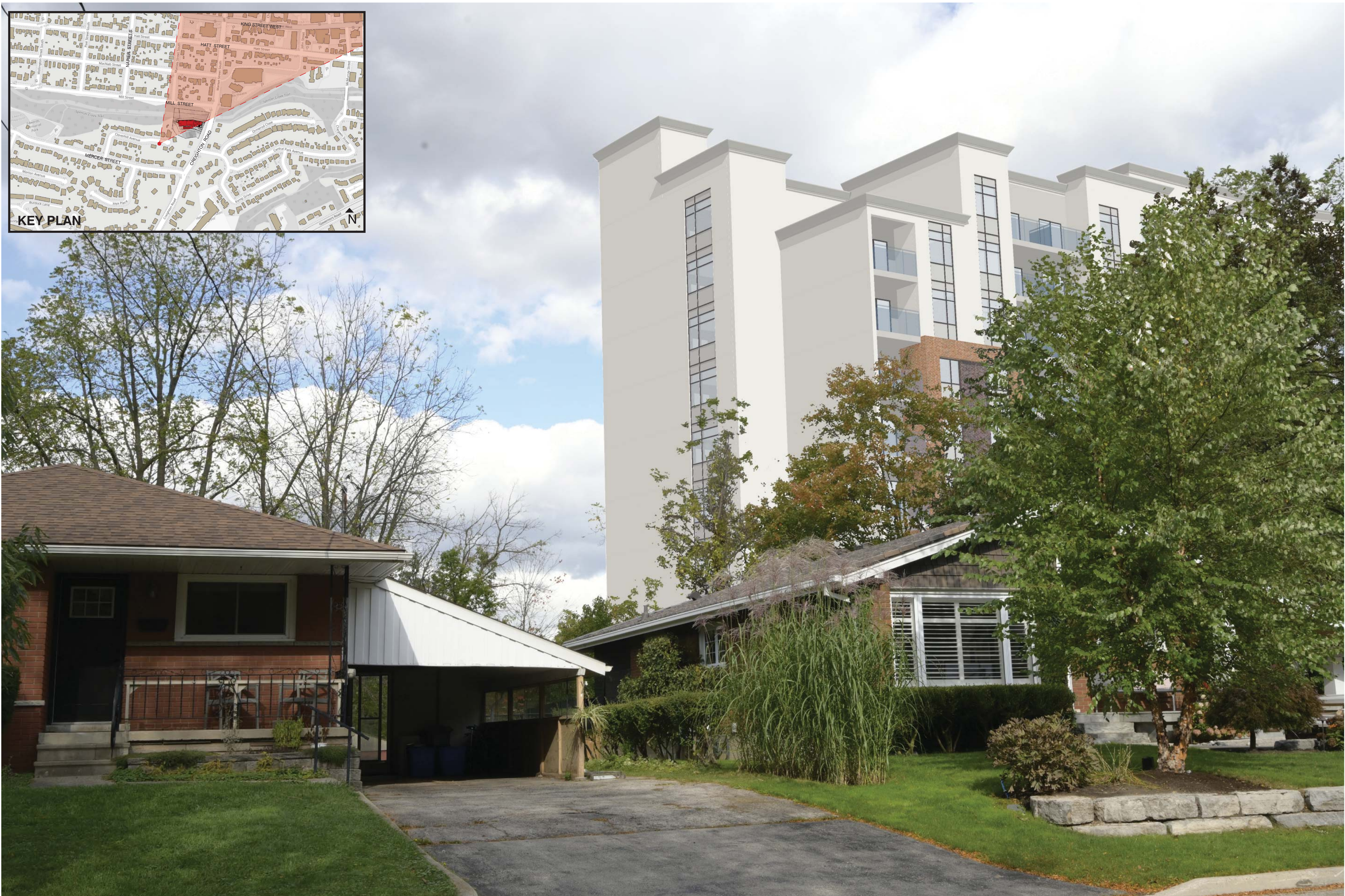
VIEW : CLOVERHILL AVENUE 80m FROM PROPOSED 12 STOREY DEVELOPMENT 50 CREIGHTON ROAD, DUNDAS, ON
