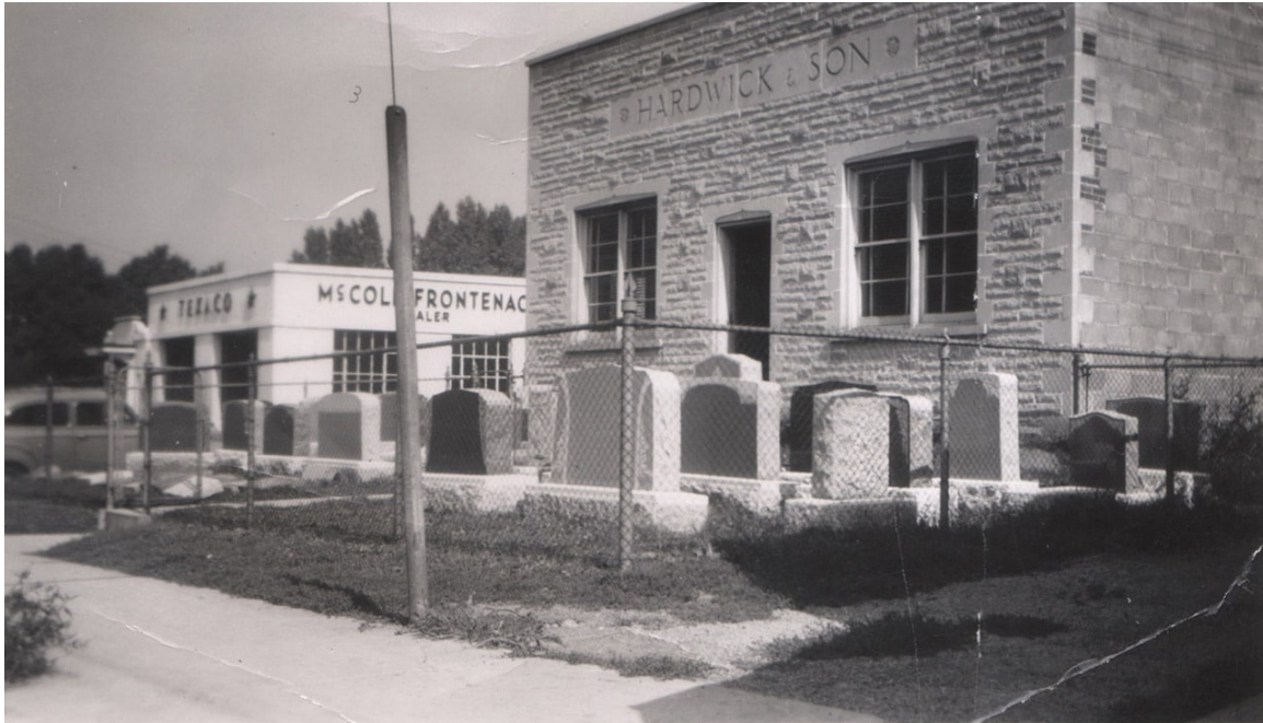
1947 HARDWICK & SON – memorials displayed in the front yard before King Street West was widened. This was their second location. H.G. Hardwick & Sons was founded in 1929 by Henry George Hardwick. His original facility on Ottawa Street was destroyed by fire in 1947. He then acquired the King Street West location and built a purpose-built showroom and workshop. The cut stone façade showcases the firm’s masonry skills.
