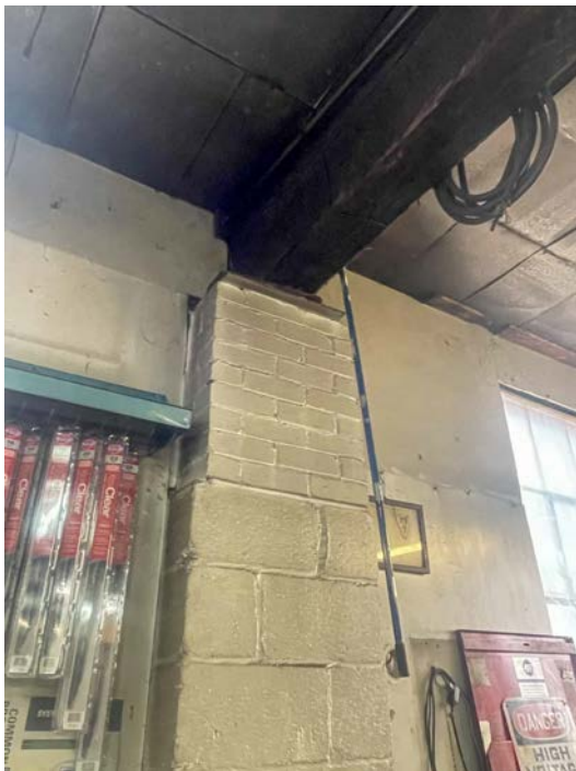
PATON MOTORS – INTERIOR – steel beam added when the eastward extension was built – two-piece bathroom with porcelain utility sink and wood panelled door
