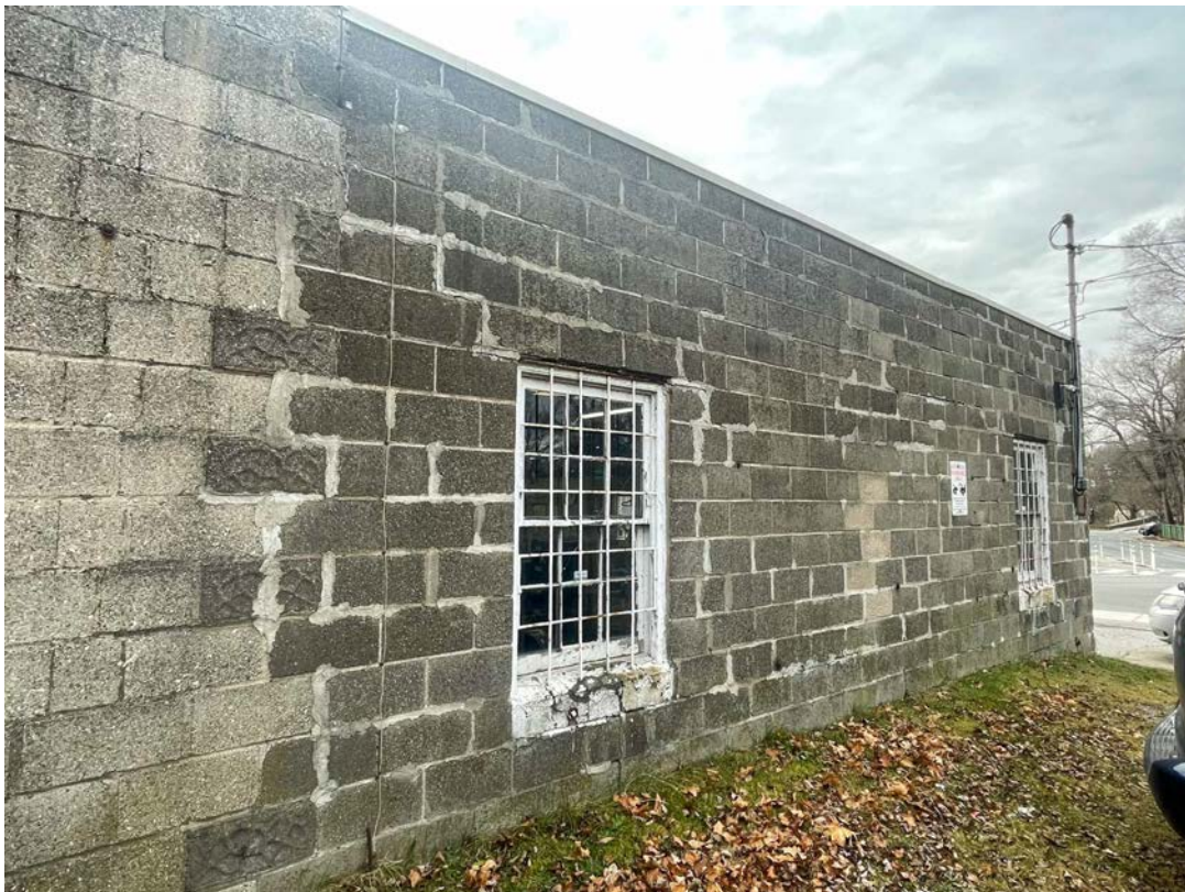
PATON MOTORS – EXTERIOR – north side elevation – 2 westerly bays with wood windows
