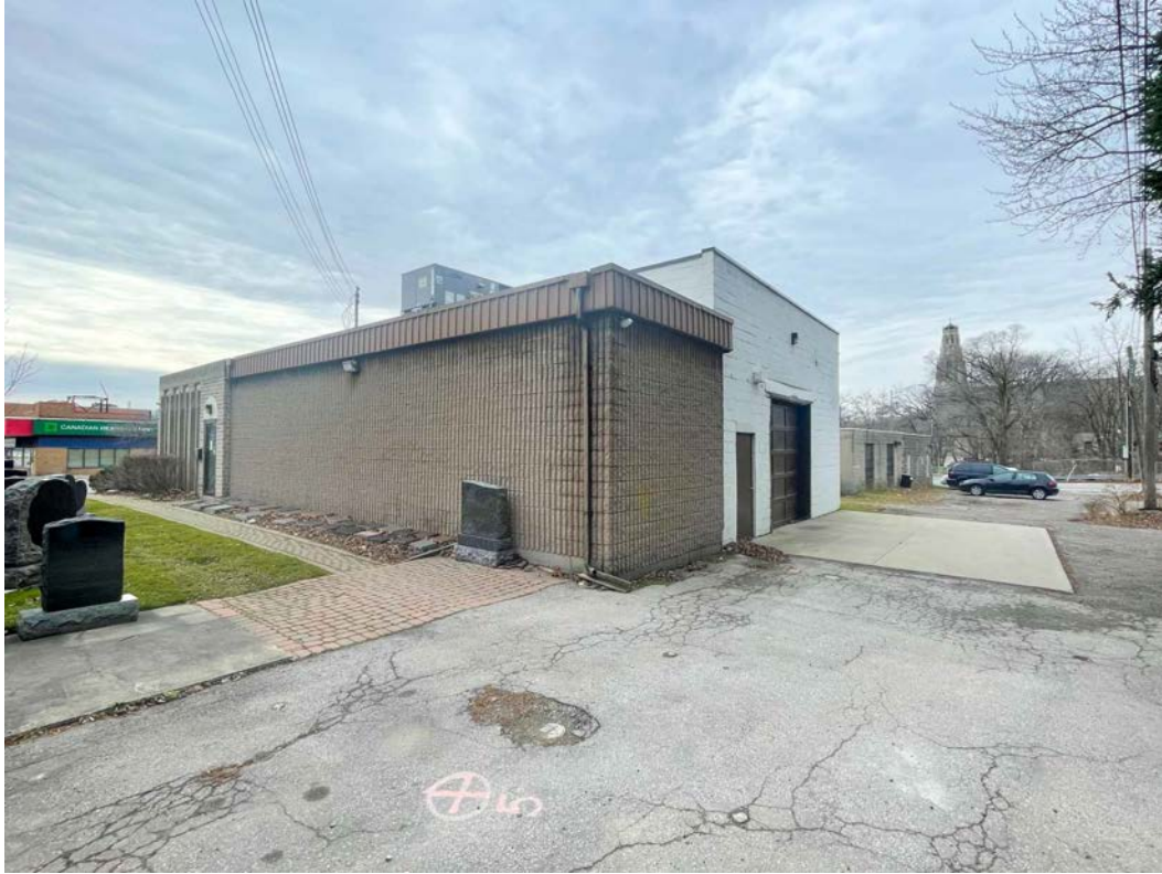
HARDWICK & SON – EXTERIOR – east side and rear elevation – cinder block addition and original concrete block workshop & warehouse – rear alley from Breadalbane – view to the Cathedral
