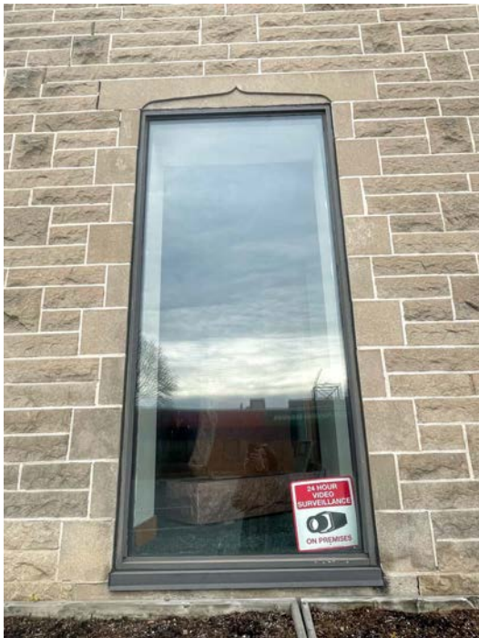
HARDWICK & SON – EXTERIOR – stone engraved with “Hardwick & Son” and two rosettes – carved stone lintels with stylized ogee arches – the central doorway has been converted to a window
