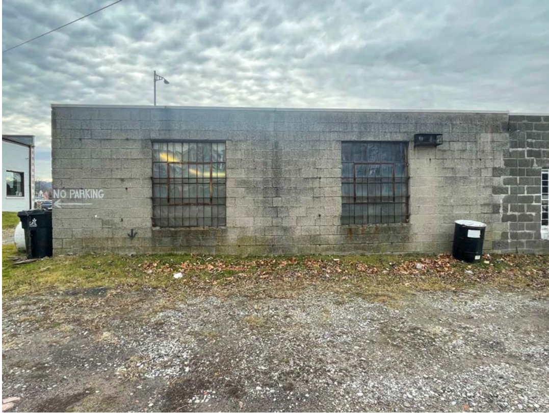
PATON MOTORS – EXTERIOR – north side elevation – 2 easterly bays with steel windows
