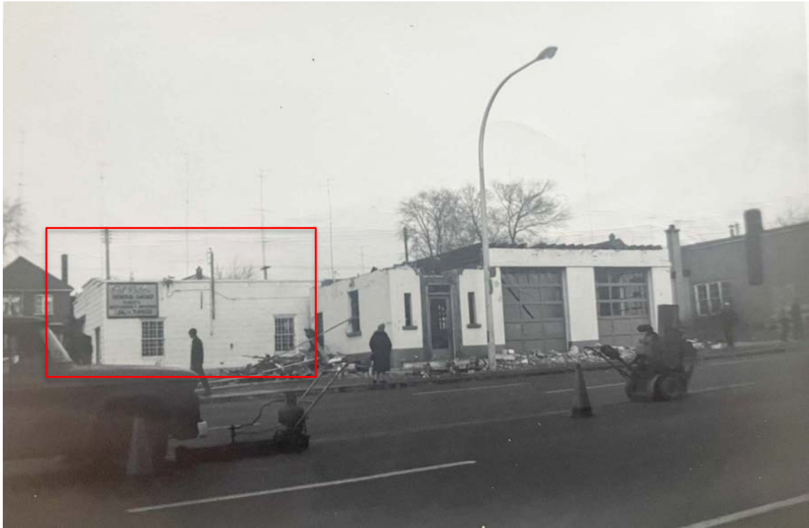
PATON MOTORS - the Texaco Service Station demolition underway in 1963
