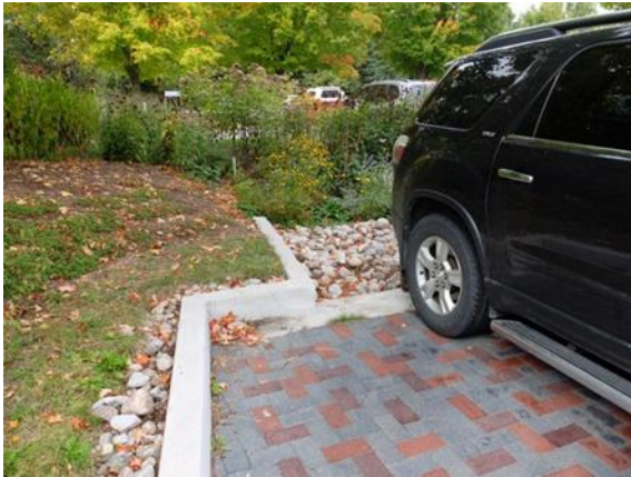
Figure 30: Rain gardens and permeable pavement, Kortright Centre, September 2015, OMC photo
