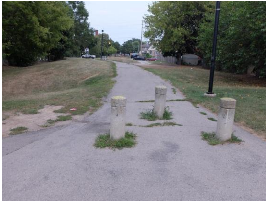
Figure 37: Paling Avenue, OMC photo
