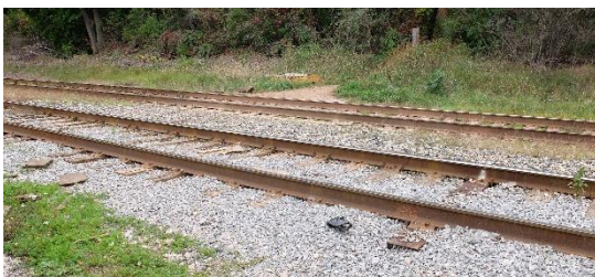
Figure 11: View toward rail crossing, across tracks, looking south, OMC photo
