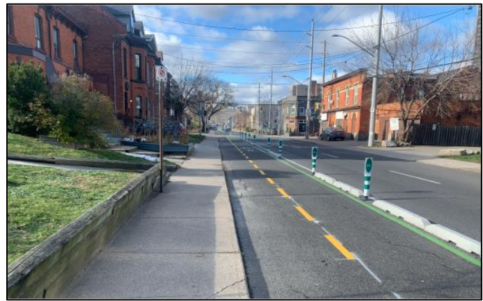
Hunter St, Hamilton Two-way cycle track with precast curbs and flexposts
