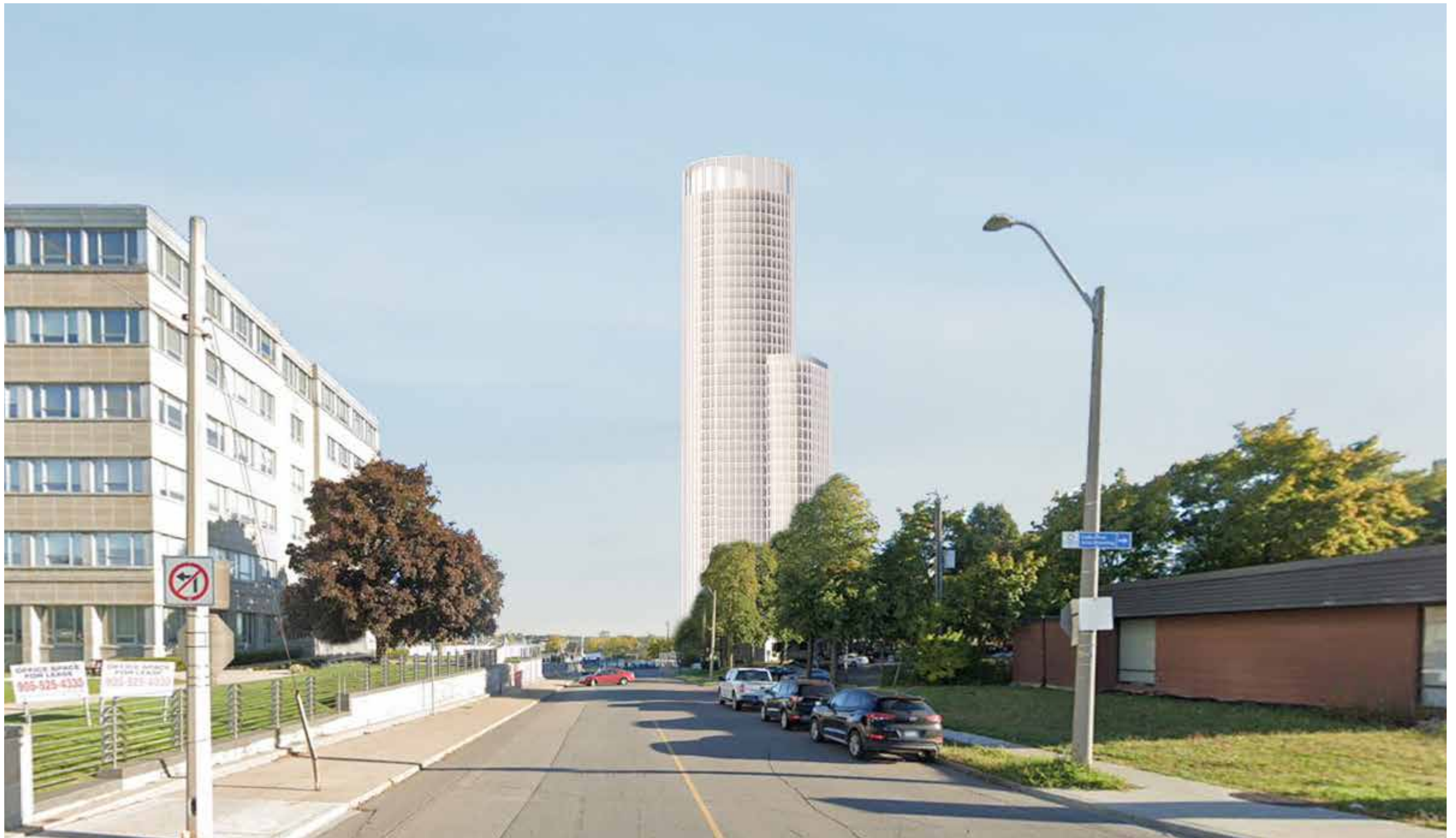
Option 1 Cylinder - View from James Street North and Burlington St. (Looking North)
