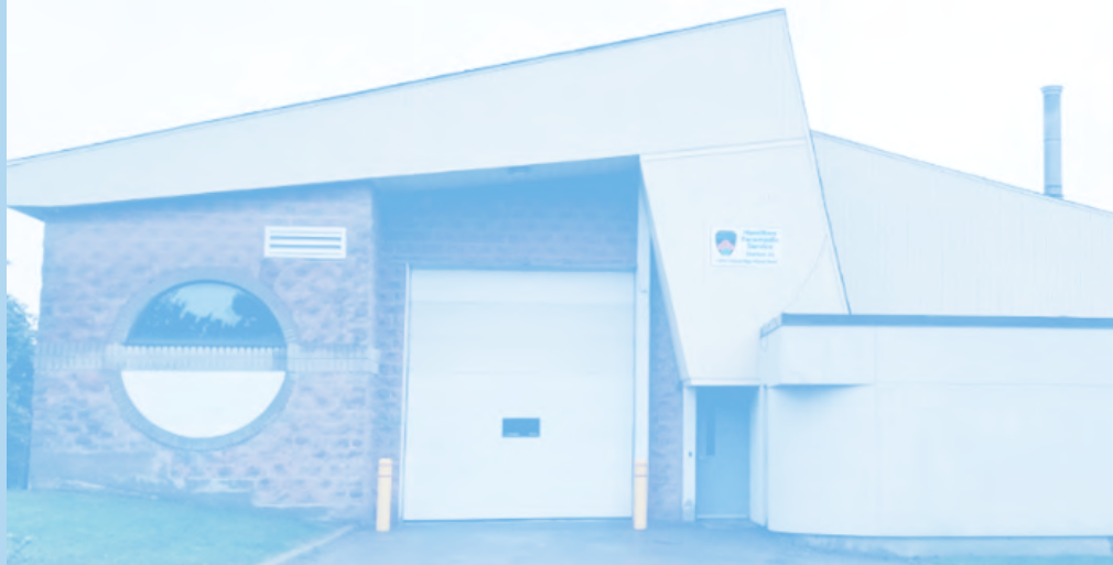
HPS Station 32, Limeridge Rd. E, Hamilton
