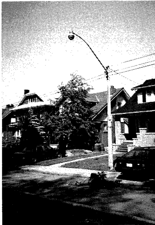
Present-day, City-wide lighting standard: concrete utility pole with an elliptical arm and tungsten luminaire.
