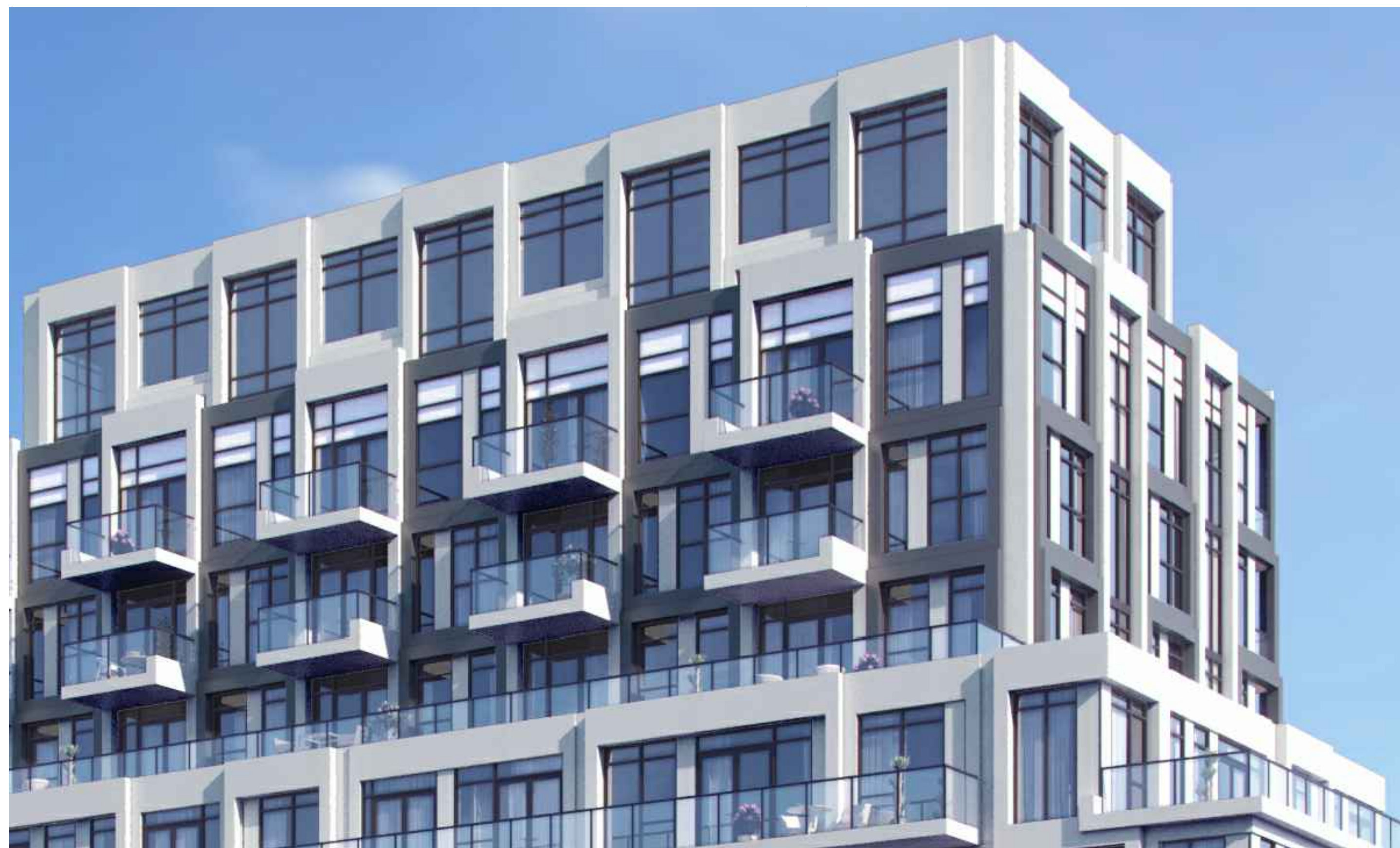
VIEW OF UPPER BUILDING FACADE DETAILS
