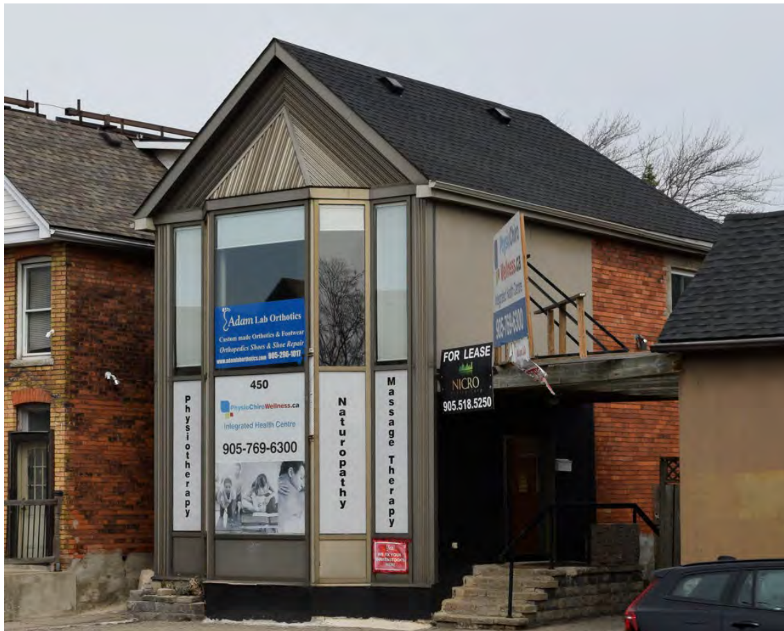
FIGURE 24: 450 MAIN STREET WEST, FACING NORTH FROM SOUTH SIDE OF MAIN STREET WEST
