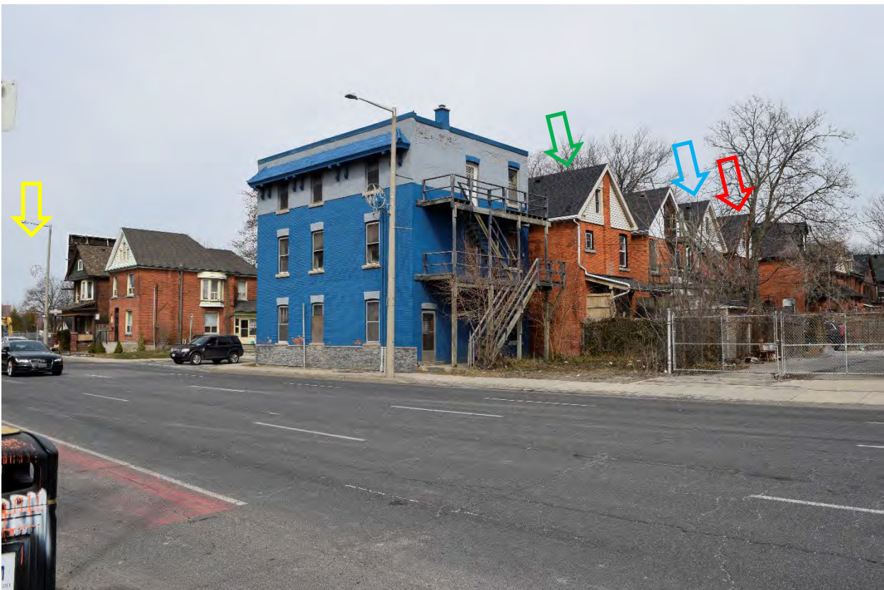
FIGURE 23: REAR EXPOSURE OF 59 (RED), 61 (BLUE) AND 65 (GREEN) STRATHCONA AVENUE SOUTH, FACING NORTHWEST FROM SOUTH SIDE OF MAIN STREET WEST, THE THREE STOREY BLUE STRUCTURE IS 67 STRATHCONA AVENUE SOUTH, ALSO AN INVENTORIED PROPERTY AS PER THE CITY OF HAMILTON HERITAGE MAPPING & RESOURCES, SUBJECT PROPERTY INDICATED BY YELLOW ARROW
