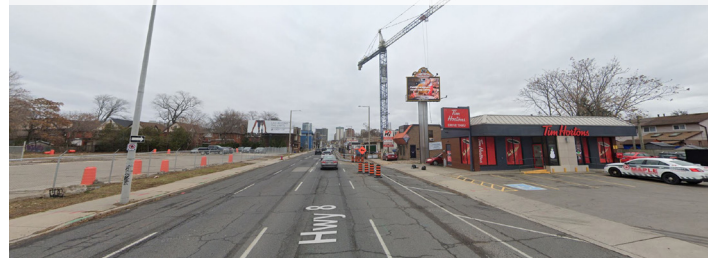
2. View towards North at New Street
