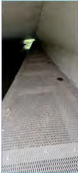
"Catwalk", Tremaine Road, Milton, Ontario
