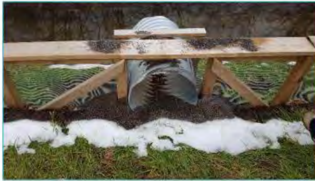
Jump-out / Escape Tunnel, Neyagawa Blvd, Oakville, Ontario
