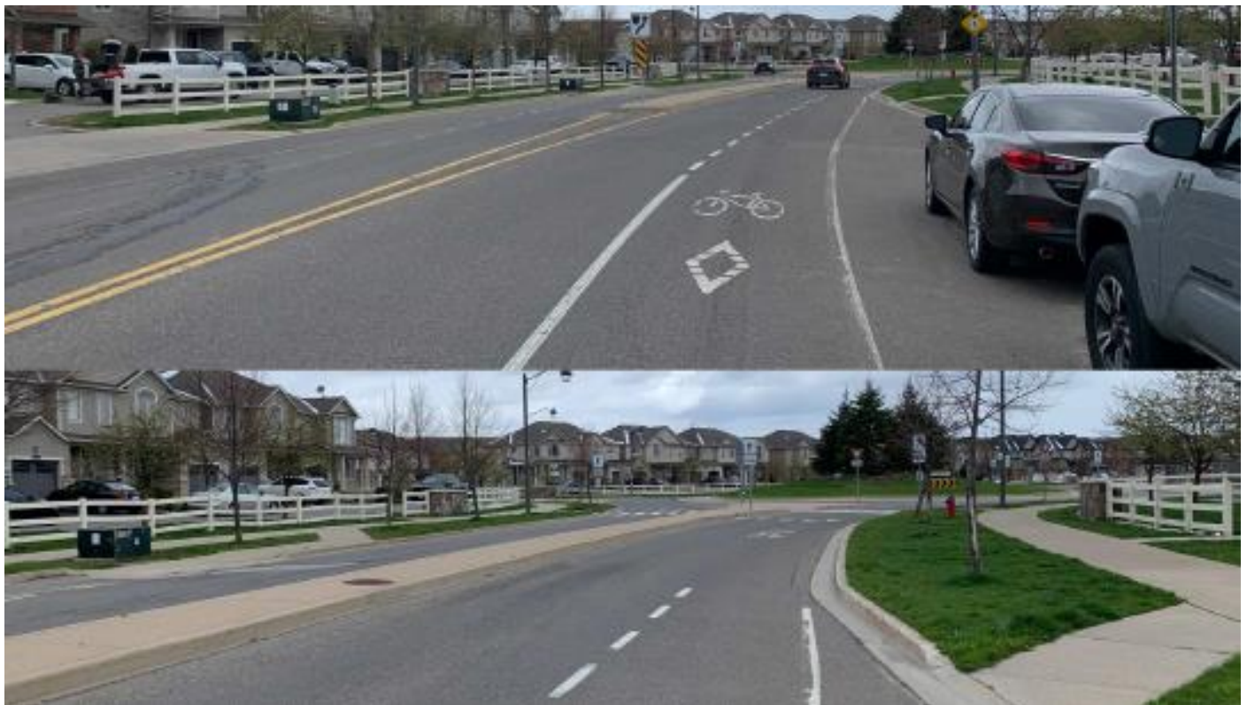
Fall Fair Way, Binbrook Bicycle lanes approaching a roundabout
