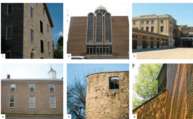
1. Ancaster Old Mill 2. Church of The Holy Spirit 3. Liuna Station 4. East Flamborough Township Hall 5. Raspberry Farm Silo 6. Goodwood Jones House
