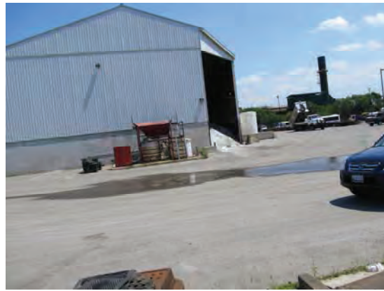
Plate 8: South-southeast view of current facility. Industrial buildings, paving, grading, and infrastructure. No potential.
