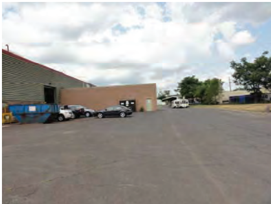
Plate 7: West-northwest view along PVT Road. Industrial buildings, ROW, and grading. No potential – all disturbed.
