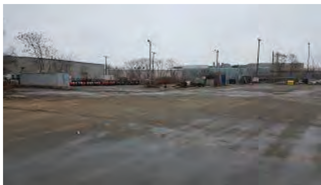
Photo 2 – View looking northwest at the northwest corner of the fleet yard at 330 Wentworth St N.
