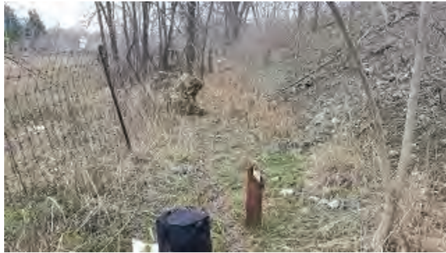
Photo 6 – View looking south at monitoring well BH32, which was installed on the east edge of the Site in 1996 for GSW Heating Products Company. On March 6, 2017, 0.86 m of LNAPL was measured in this well.
