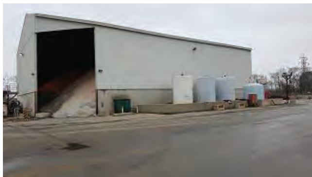
Photo 1 – View looking northwest at the salt storage structure and brine tanks located on-site in the fleet yard at 330 Wentworth St N.
