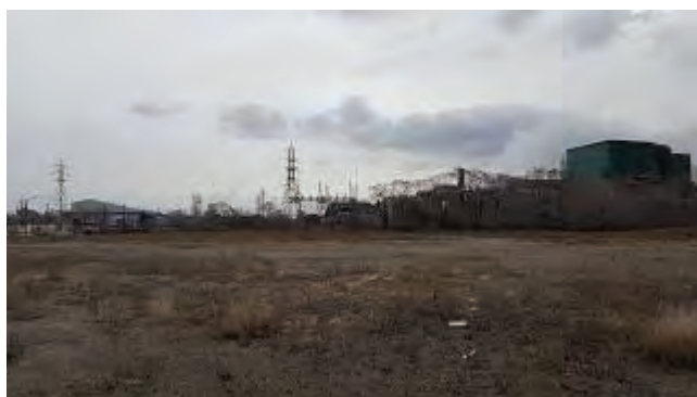
Photo 13 – View looking east across the Site from 80 Brant St. The Hamilton Specialty Bar steel plant and electrical transformer substation are visible on the adjacent property.
