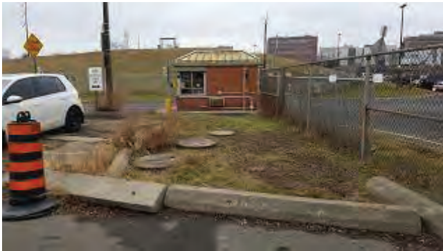
Photo 7 – View looking east across the south edge of the Site. The three manhole covers for the oil-water separator are visible in the grass area.
