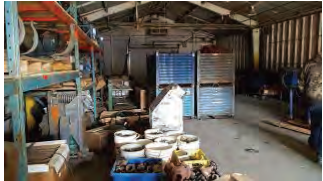
Photo 22 – View of the interior of the 2 Hillyard St building, now used for storage and workshop space by Duke Electric Ltd.
