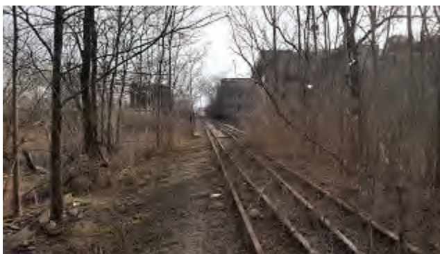
Photo 17 – View looking east along the on-Site railway tracks towards the bridge cross Birch Ave.
