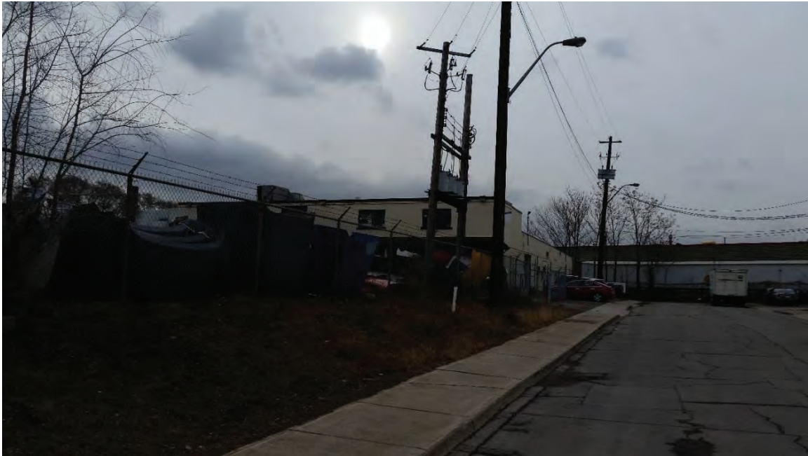
Figure 4-3 Photo of Overhead power supply and transformers
