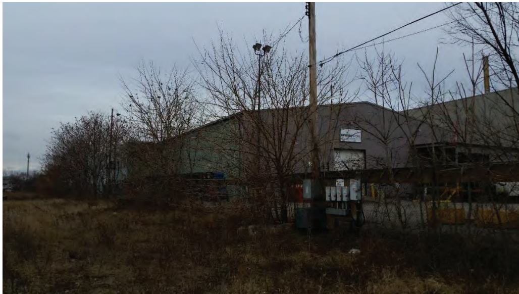
Figure 3-6 photo showing power supply and transformer cabinet
