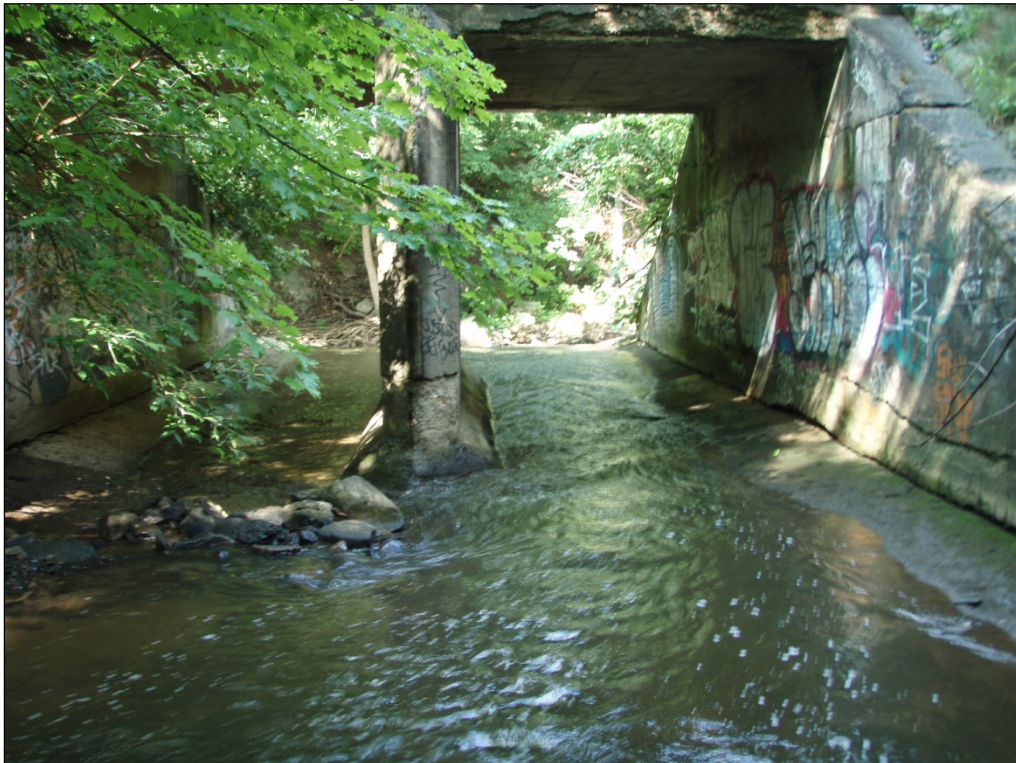
Photograph 6. July 30, 2014. Bridge beneath railway tracks, approximately 140 m downstream of Bridge 451.
