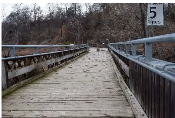
Plate 11: Wood decking, wood barriers, and steel tube railing, looking west
