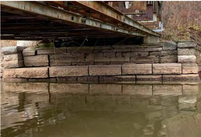
Photo 3: Upstream side of the Valley Inn Bridge; west abutment.
