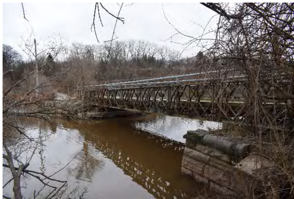
Plate 15: Truss superstructure and abutments, looking southeast
