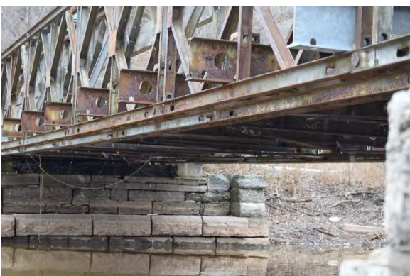
Plate 12: Stringers, I-beams, and cross bracing supporting decking, looking northwest
