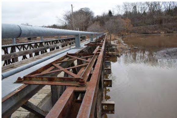
Plate 16: Horizontal cross bracing, looking east
