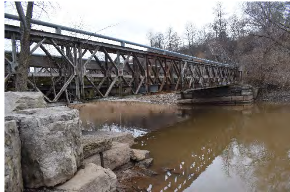
Plate 21: Stone abutment on east side of bridge, looking southwest
