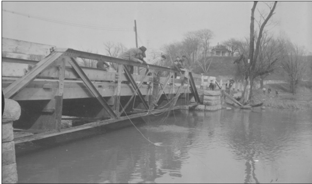
Plate 7: Valley Inn Bridge looking northeast 1960 (Hamilton Public Library, Local History & Archives)
