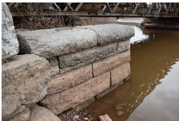
Plate 19: Stone abutment on west side of bridge, looking northeast
