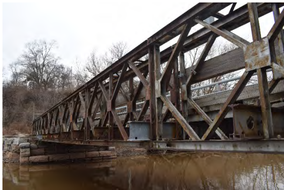
Plate 14: Truss superstructure, looking northwest
