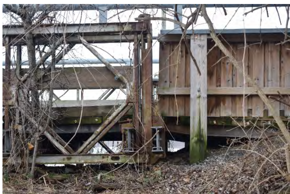
Plate 18: Original southwest end post, looking southeast
