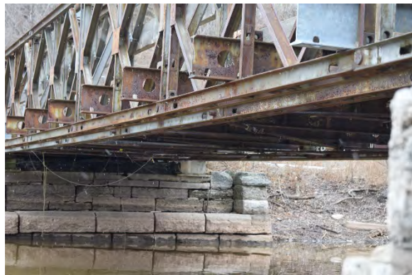
Plate 18: Stringers, I-beams, and cross bracing supporting decking, looking northwest
