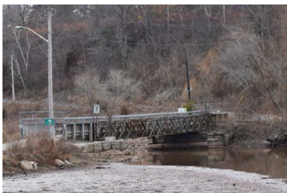
Plate 9: Valley Inn Bridge, looking southwest
