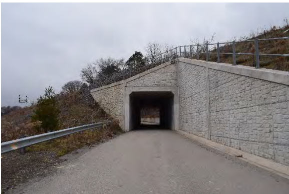
Plate 12: Railway overpass, looking southwest
