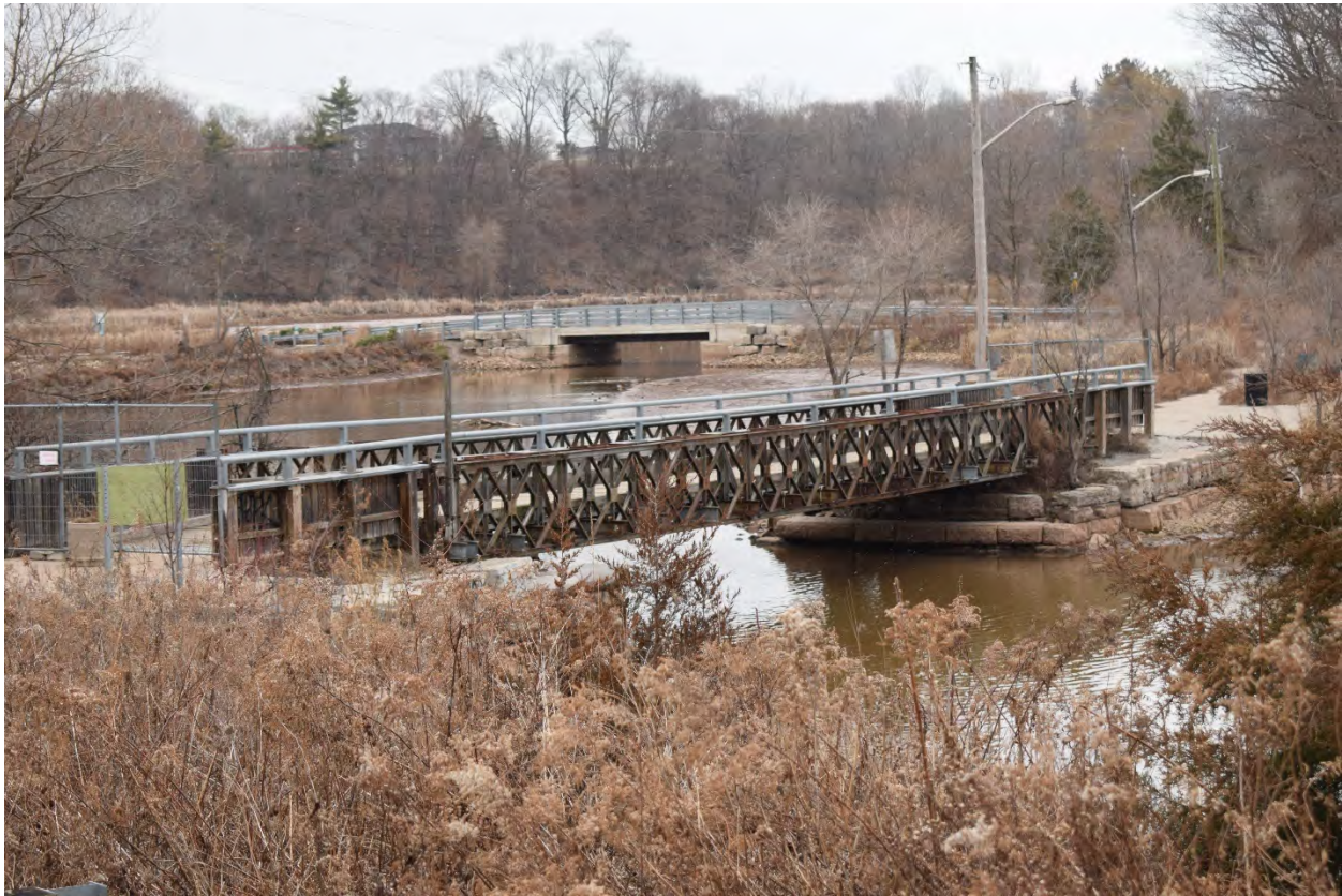
Plate 16: Valley Inn Bridge, looking northeast
