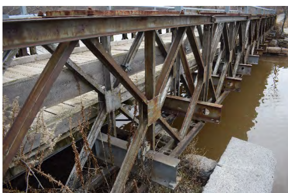
Plate 13: Stringers, I-beams, and cross bracing supporting decking, looking northeast
