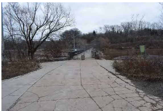
Plate 7: Concrete paving just west of bridge, looking east
