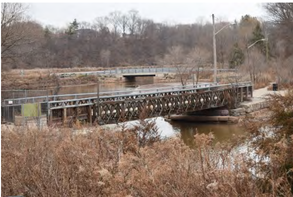
Plate 8: Valley Inn Bridge, looking northeast
