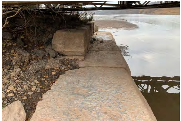
Photo 4: East bridge abutment, facing downstream (south) towards Carroll's Bay
