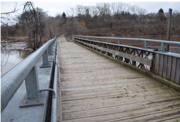
Plate 17: Wood decking, wood barriers, and steel tube railing, looking east
