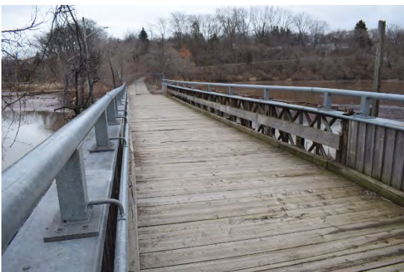
Plate 10: Wood decking, wood barriers, and steel tube railing, looking east
