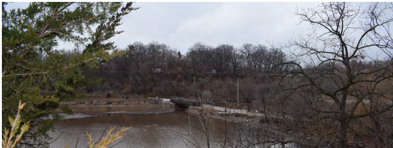
Plate 9: Looking northwest from Spring Gardens Road to the Valley Inn Bridge and the confluence of Lake Ontario and Grindstone Creek
