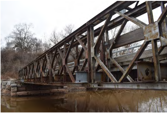
Plate 19: Truss superstructure, looking northwest
