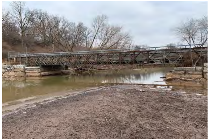
Photo 6: Downstream (south) of the Valley Inn Bridge, facing upstream (north).
