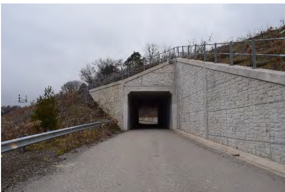
Plate 4: Railway overpass, looking southwest
