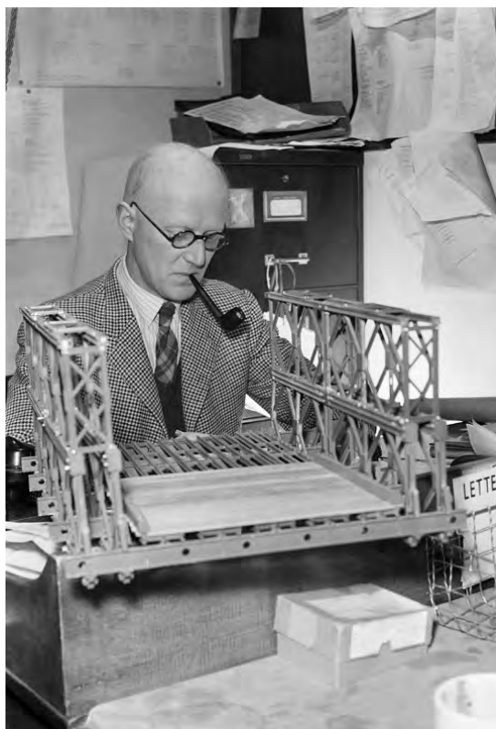
Plate 30: Donald Bailey with a model of the Bailey Truss Bridge in 1944 (Imperial War Museum 1944)
