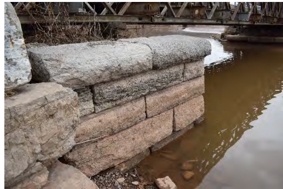
Plate 22: Stone abutment on west side of bridge, looking northeast
