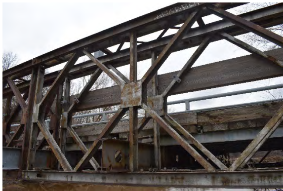
Plate 17: Bracing details, looking northwest
