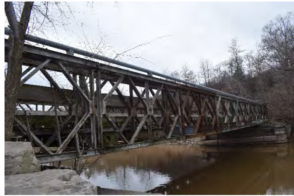
Plate 20: Truss superstructure, looking southeast
