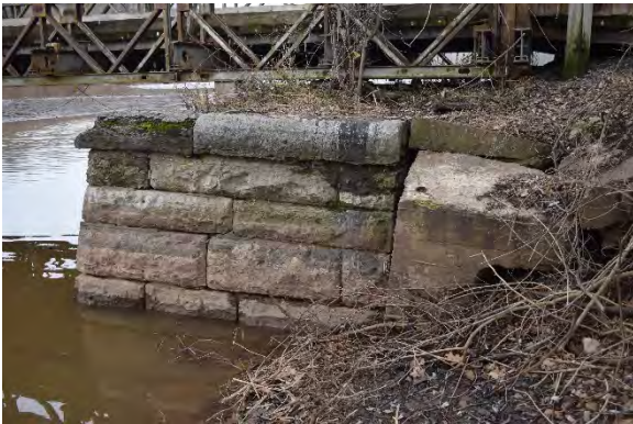
Plate 20: Stone abutment on west side of bridge, looking southeast
