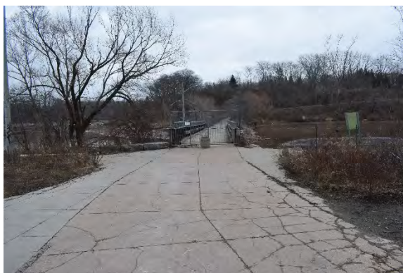
Plate 15: Concrete paving just west of bridge, looking east
