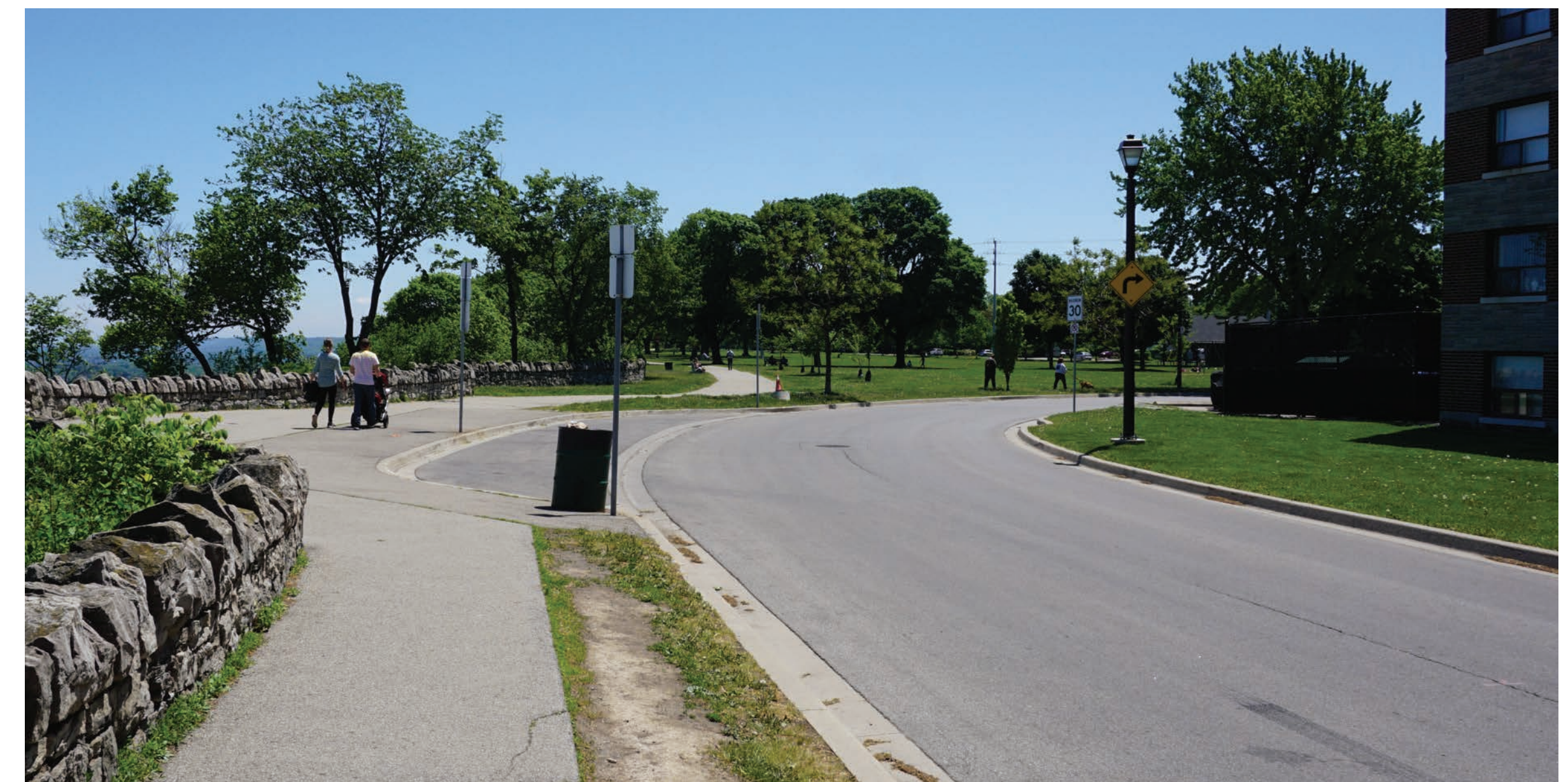
Existing Streetscape Conditions
