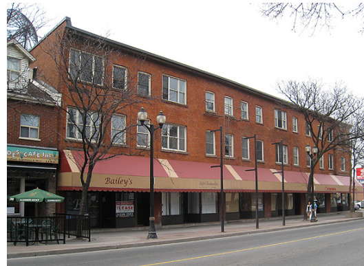
4. Hamilton Brass Manufacturing Co. Building - 1873
