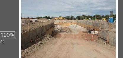
To date, excavation of the Tertiary Facility foundation has completed, with concrete forming/pouring underway. Demolition of the first stage of the south aeration and secondary clarifier works is mostly complete, with excavation and site works underway. Work began in the Red Hill Creek which is expected to finish this year.
