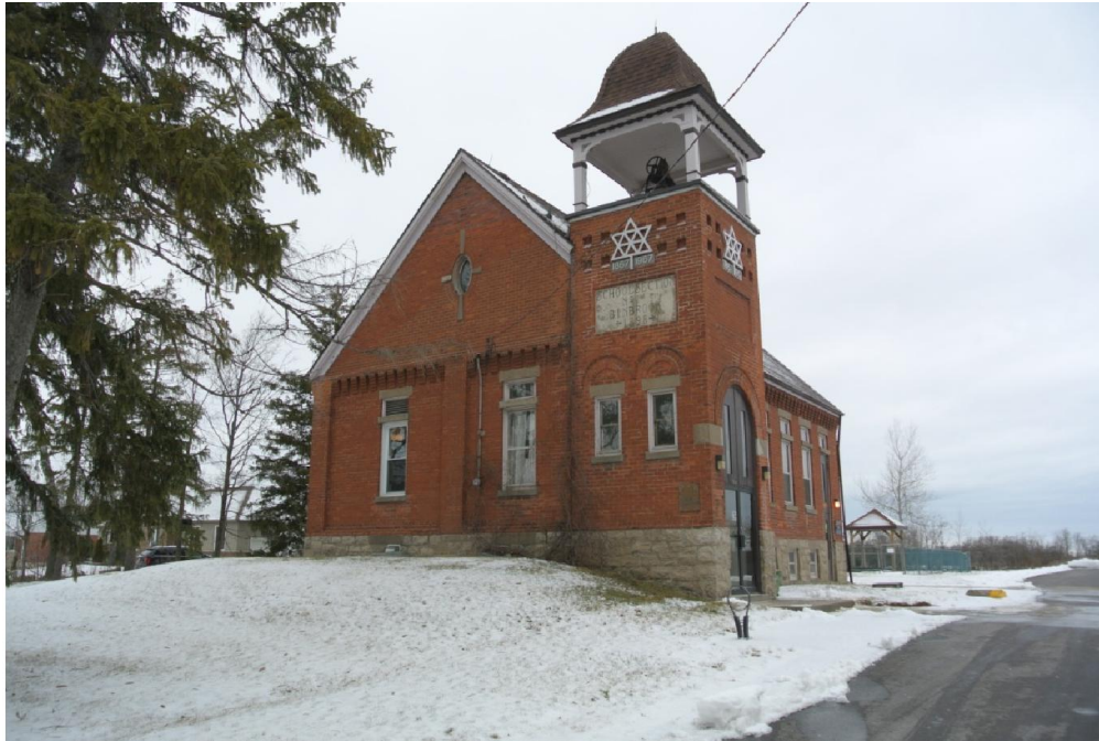
Plate 1: South (front) elevation of the subject resource.
