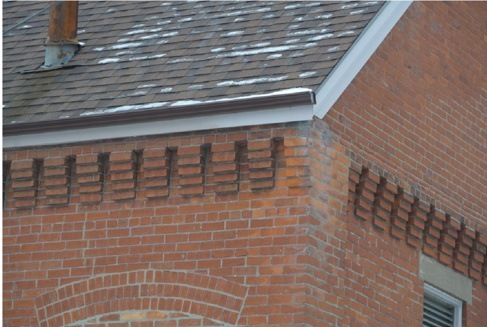
Plate 5: Detail of brick corbel trim along the roof line.
