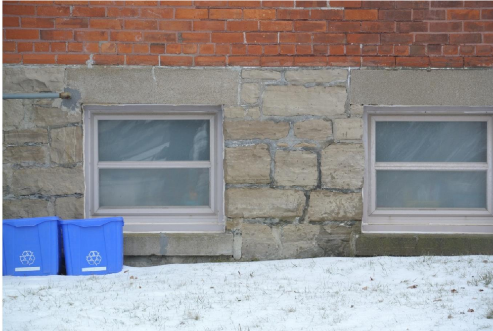
Plate 13: Detail of the basement fenestration.
