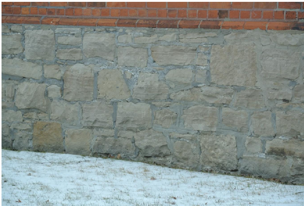
Plate 6: Detail of the cut stone foundation.
