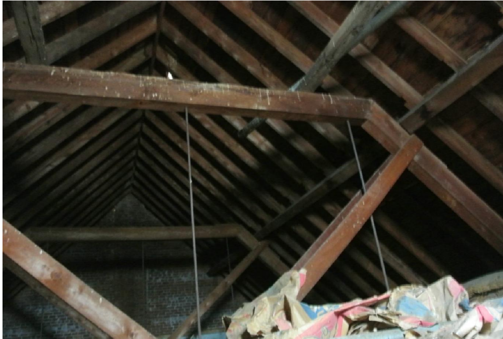
Plate 23: View of the attic.
