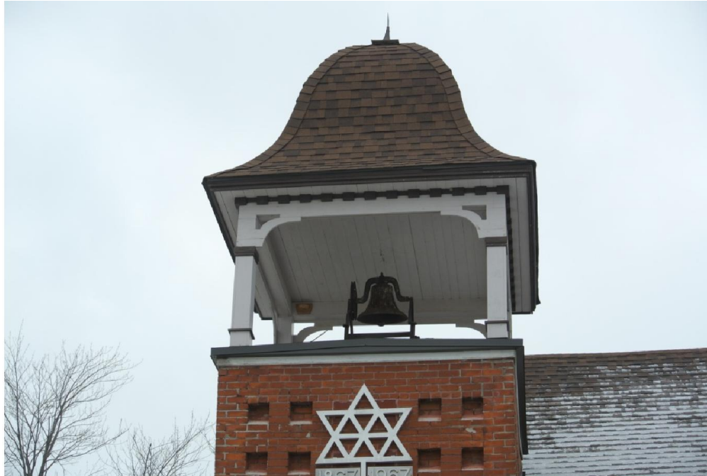
Plate 7: Detail of the bell-shaped roof supported by wooden posts of the bell tower.
