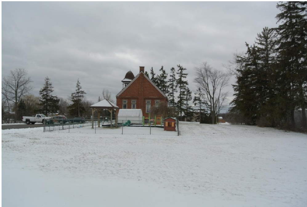
Plate 28: Looking south across the lawn toward the playground and the north elevation of the subject resource.
