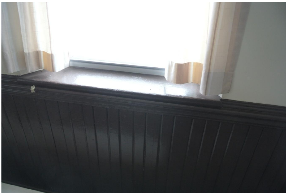
Plate 20: Detail of the wainscoting and window sill on the main floor.
