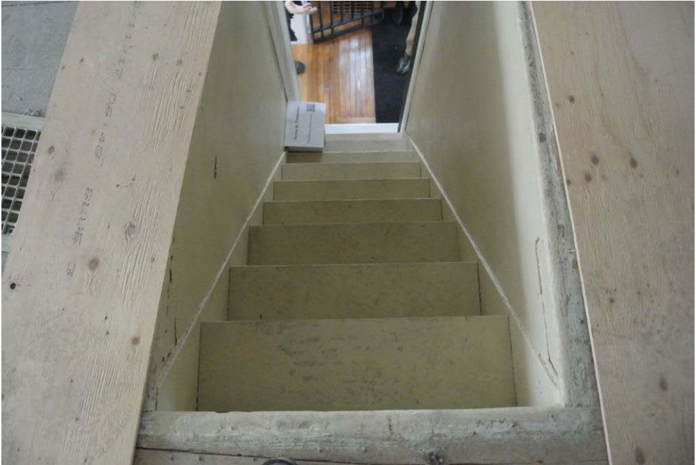
Plate 22: View down the stairwell from the half-storey.
