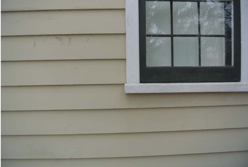
Plate 9: Detail of the clapboard siding.
