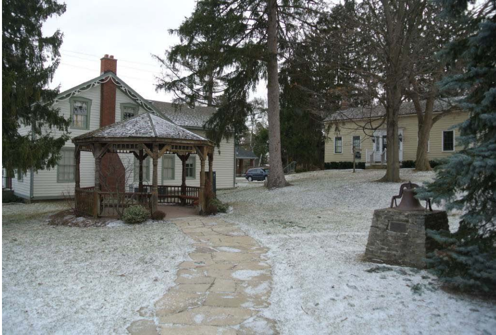
Plate 25: View of generally north from Wilson Street East. Note the relationship between the Tisdale House (right), the Hammill House (left), and the modern Gazebo (foreground).
