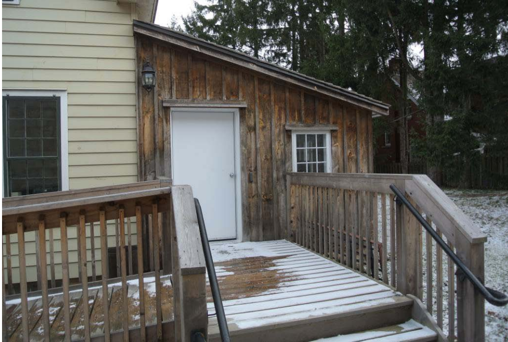
Plate 13: View toward the modern addition at the rear of the building.
