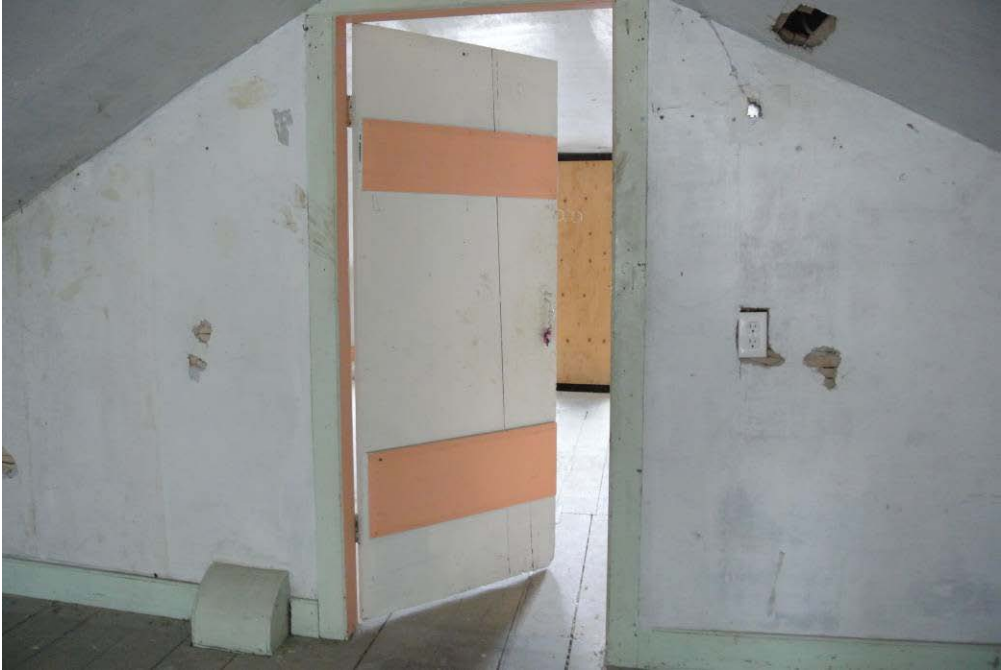
Plate 23: View of the interior of the half-storey.
