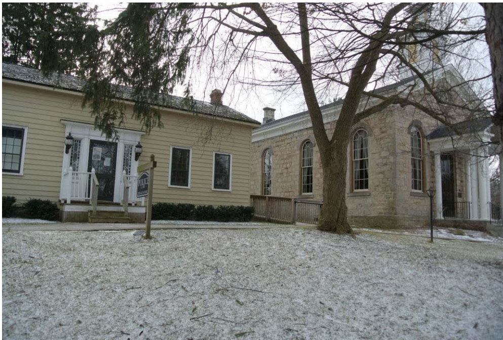
Plate 26: Looking generally east from the interior of the property at 314 Wilson Street East. Note the relationship between the Tisdale House and the former Ancaster Town Hall.
