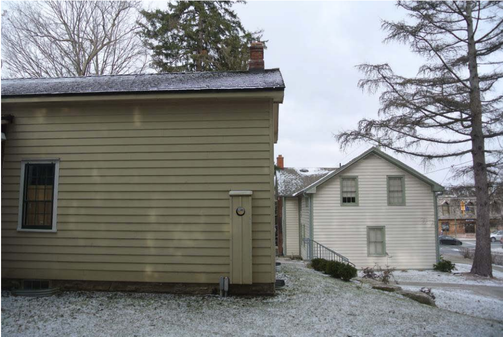
Plate 8: View west toward the Hammill House from the west elevation of the Tisdale House.
