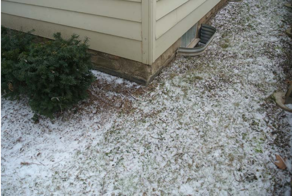
Plate 5: Detail of the stone cladding covering the concrete foundations.
