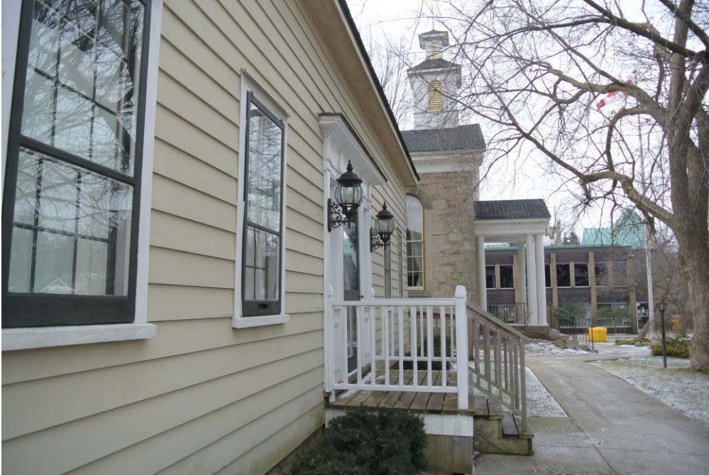
Plate 7: Oblique view of the west elevation.
