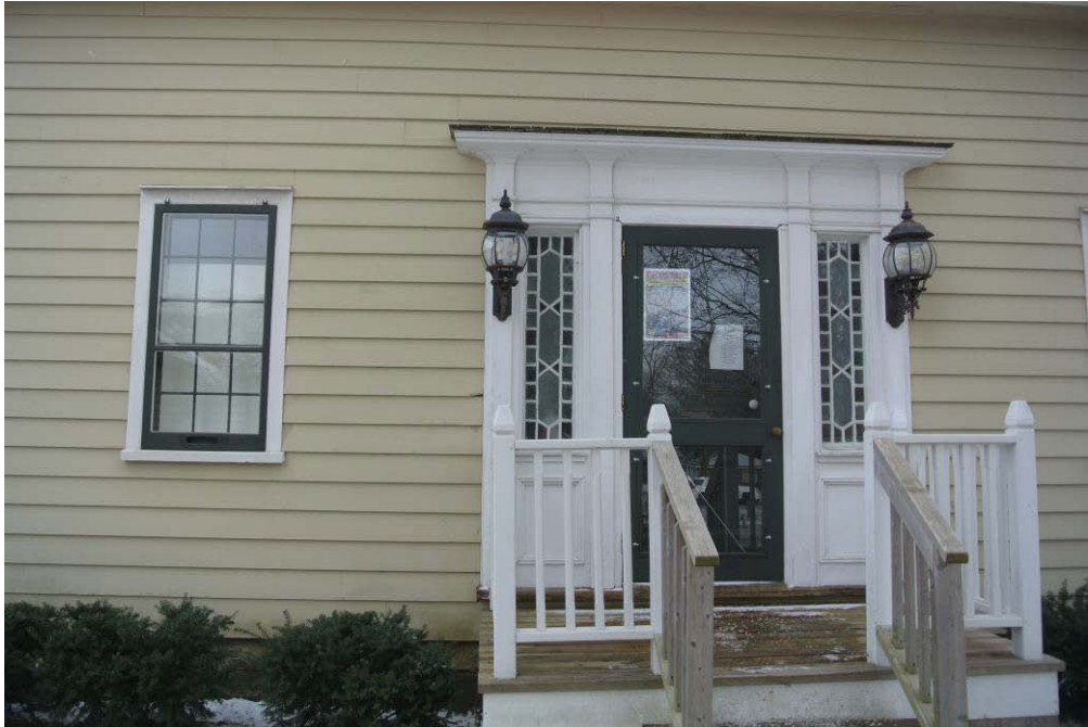
Plate 6: View toward the entryway on the west elevation.
