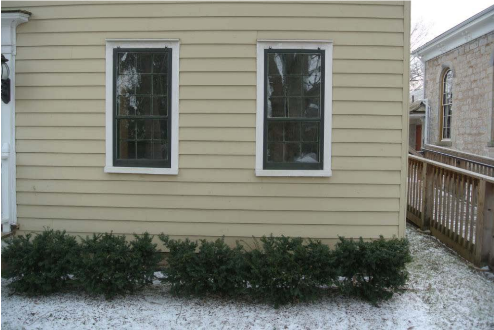
Plate 12: Detail of the fenestration on the east elevation.
