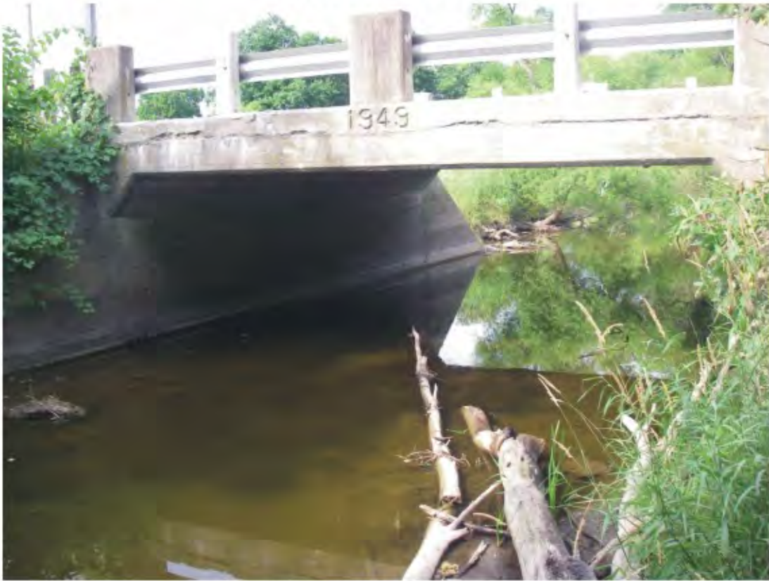
Westover Road - Upstream side
