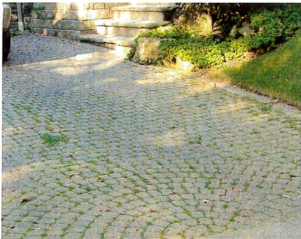
Porous (permeable) driveway
