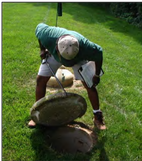
Inspection of Septic Tank (Source CJ Septic)
