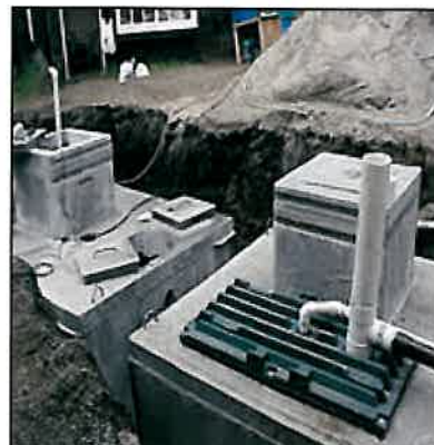
Septic Tank Replacement (Source US EPA)
