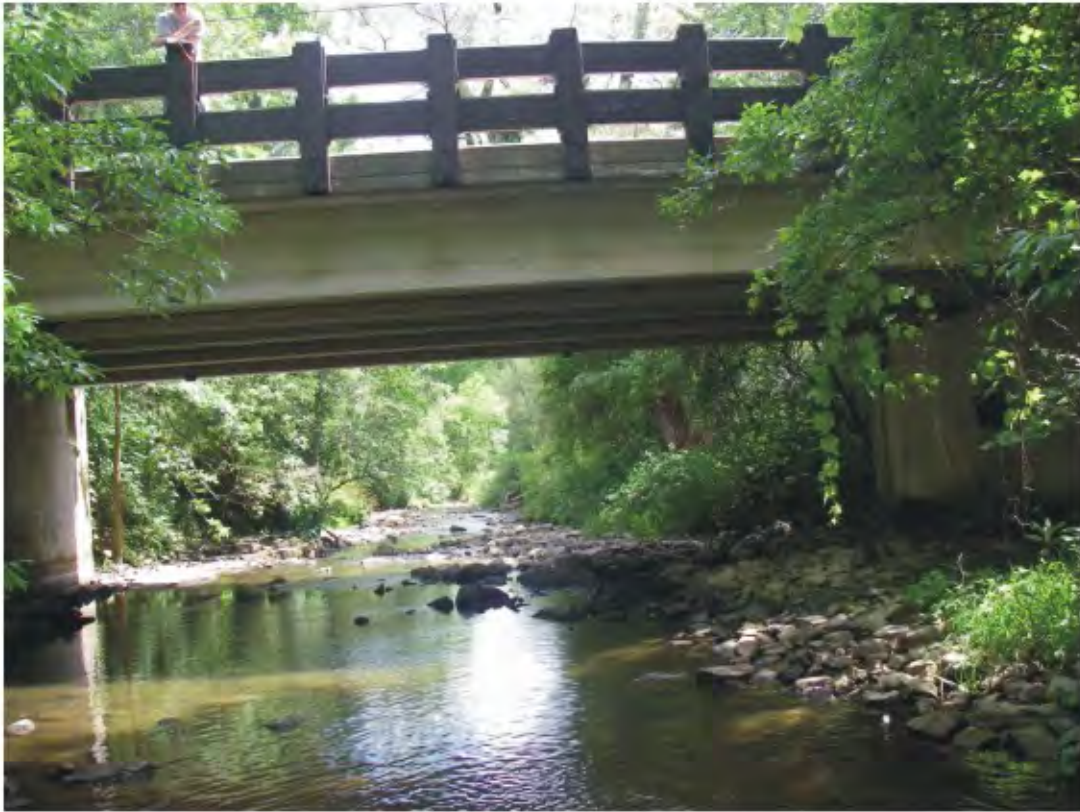
Crooks Hollow - Upstream side
