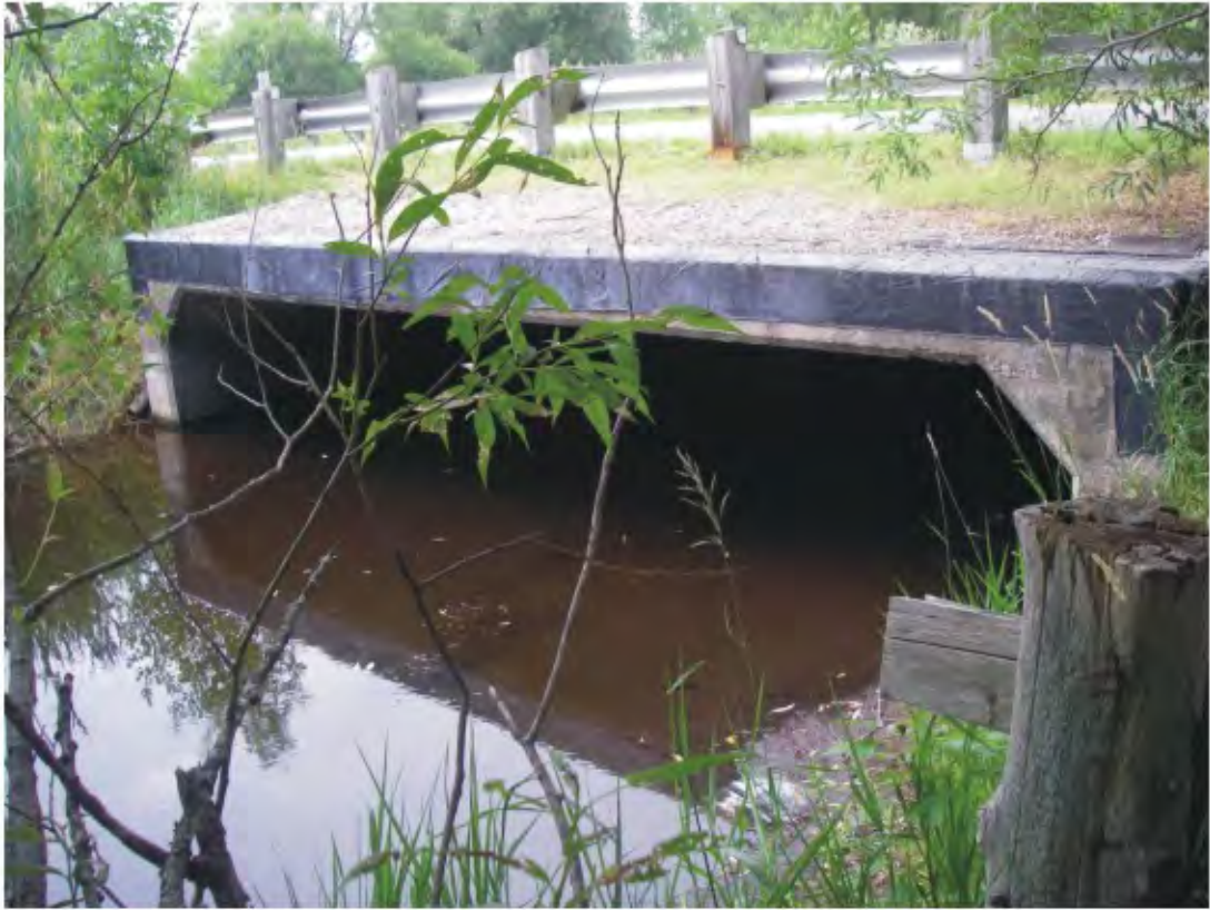
Concession 5 - Downstream side
