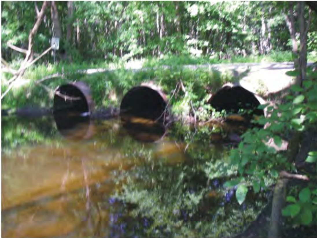
Middletown Road - Upstream side
