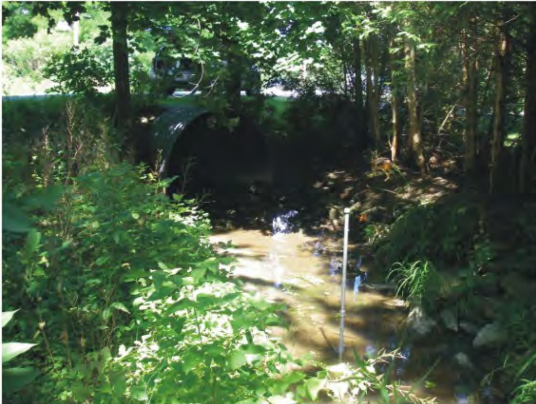
Park Avenue - Downstream side
