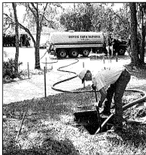
Pumping of Septic Tank (Source US EPA)
