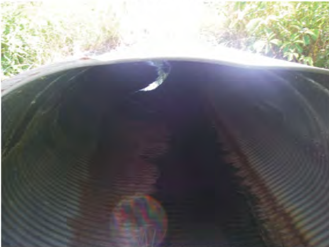
Mountain View Road - Upstream side
