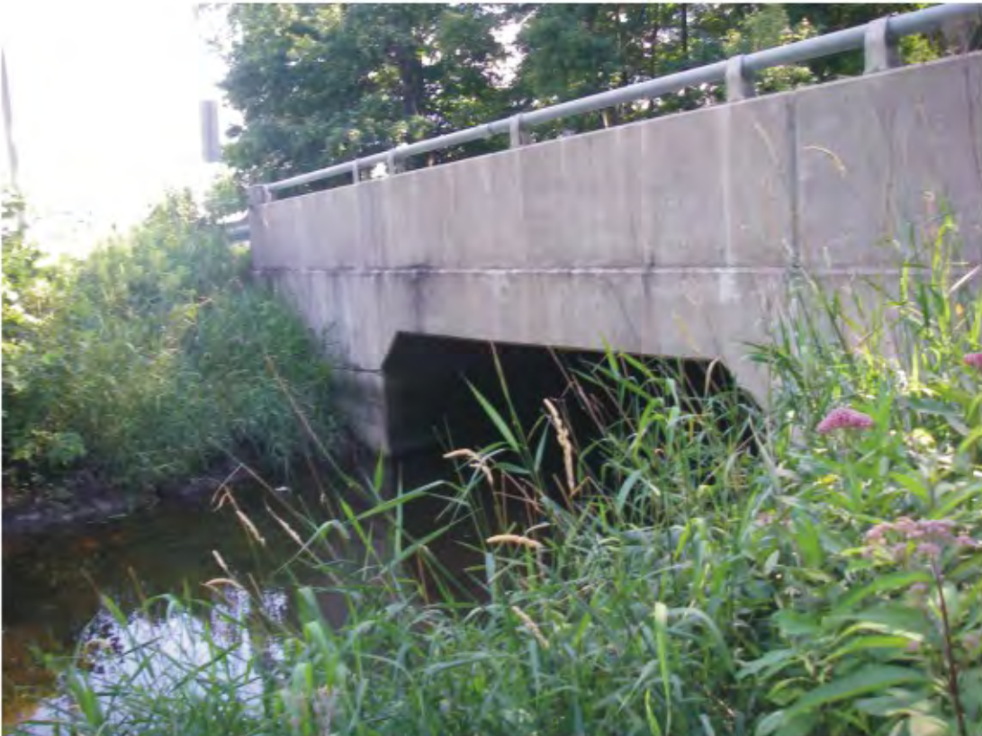
Middletown Road - Downstream side
