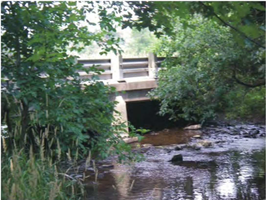
Concession 4 - Downstream side
