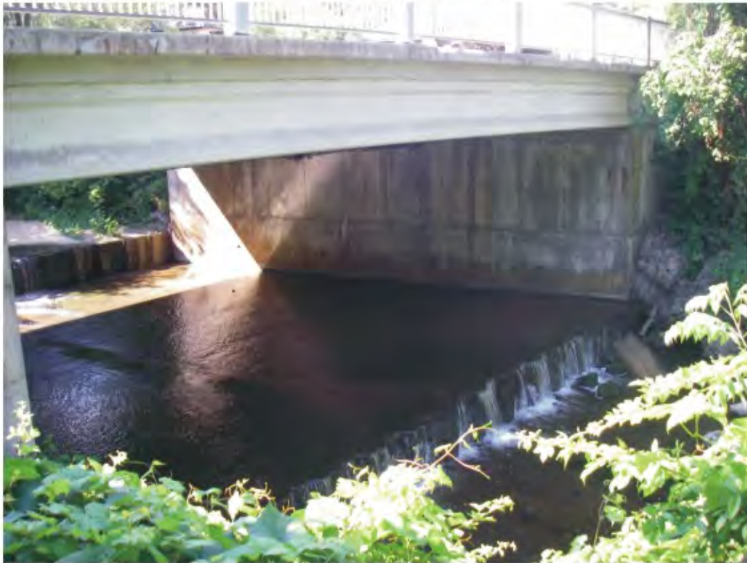
Market Street - Downstream side
