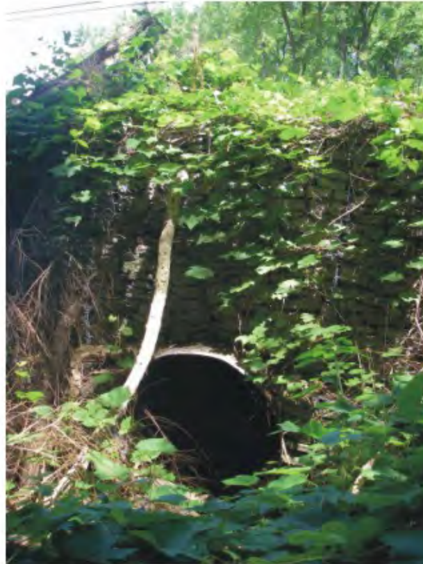
Highway 8 - Upstream side
