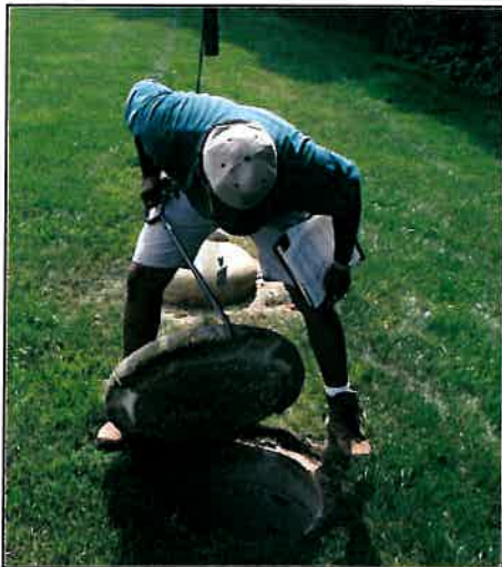
Inspection of Septic Tank (Source CJ Septic)
