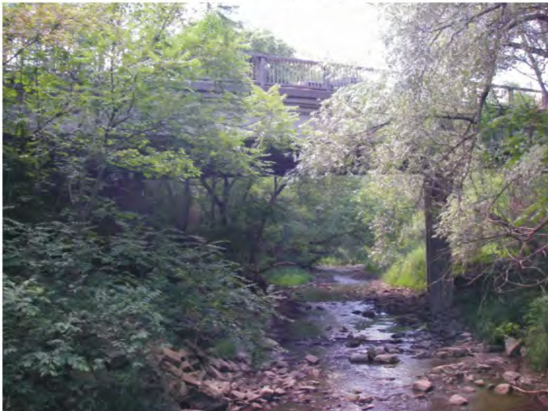
Brock Road - Downstream side
