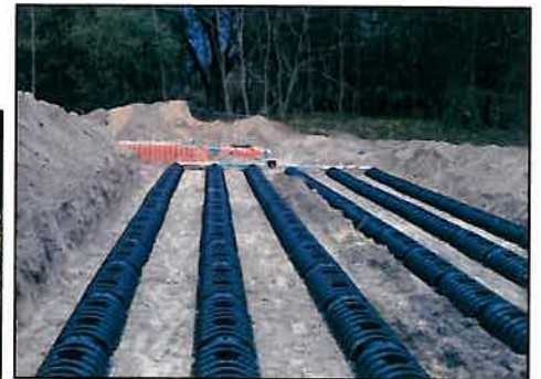
Septic Bed Replacement (Source SW Soil)
