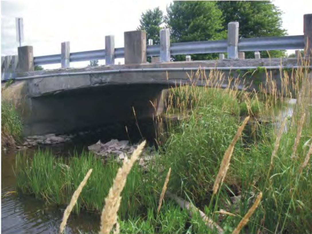
Westover Road - Upstream side
