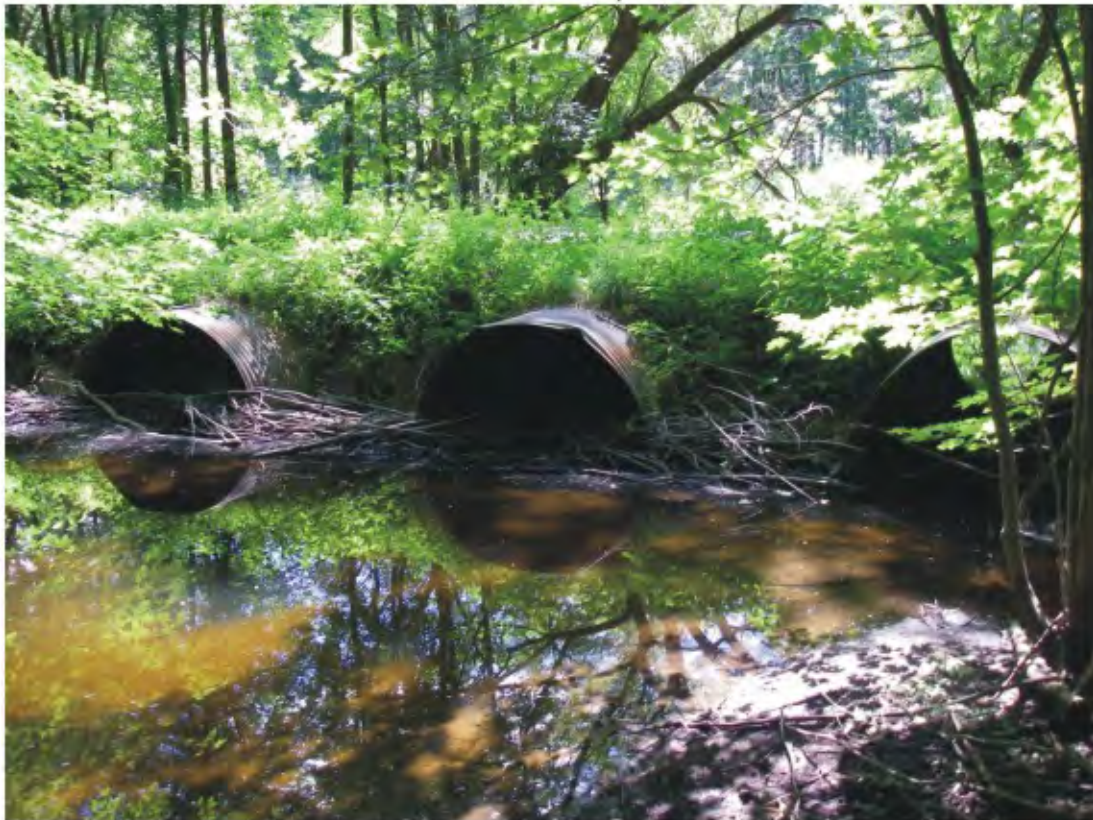
Middletown Road - Downstream side
