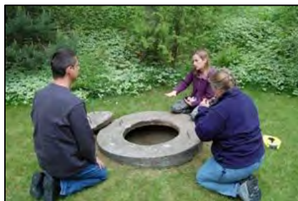
Ground around your wellhead should be graded away to ensure surface runoff does not flow in. The area should be maintained with low-growing grass . (Source WellAware.ca)
