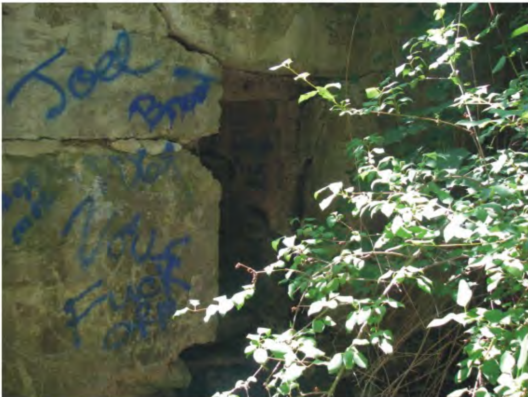
Highway 8 - Downstream side
