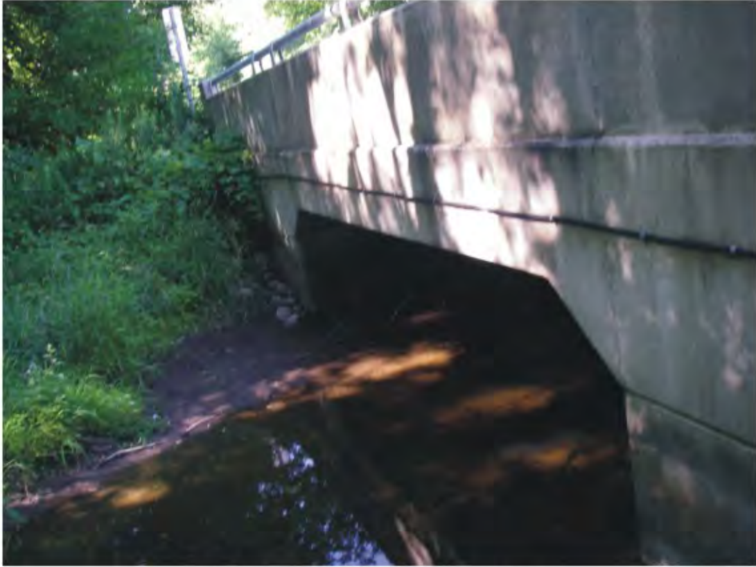
Middletown Road - Upstream side
