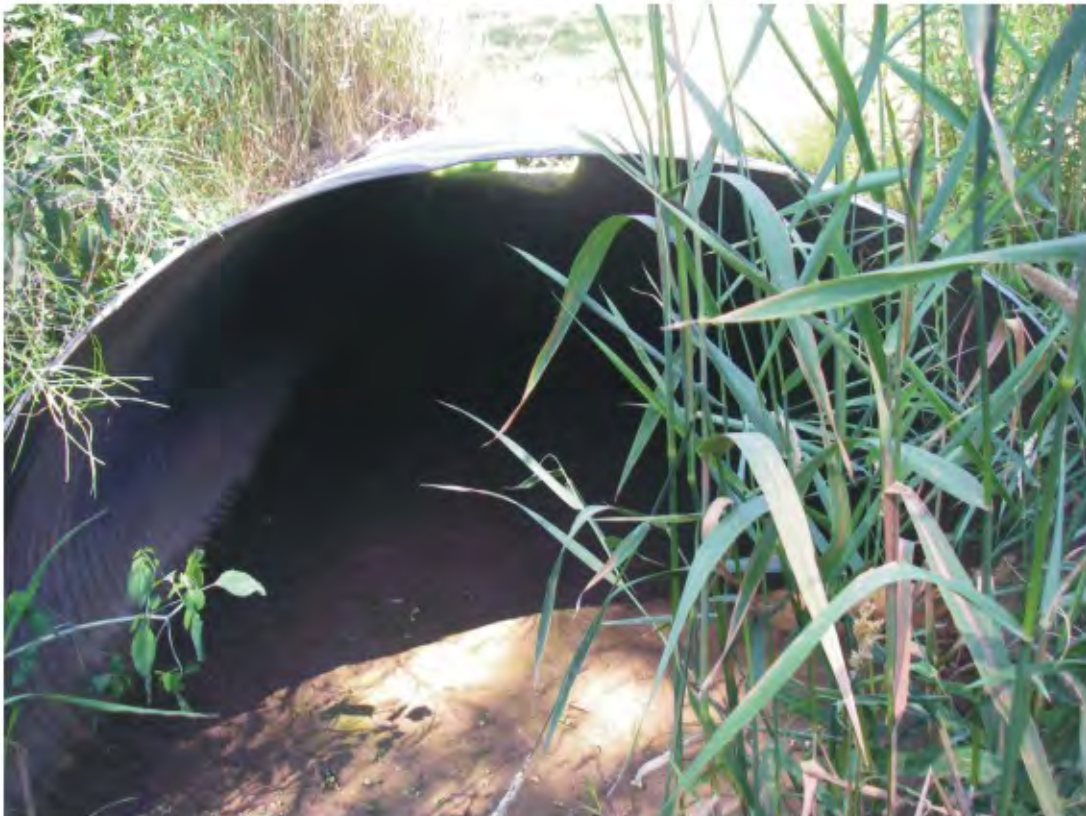
Parkway off Oak Avenue - Downstream side
