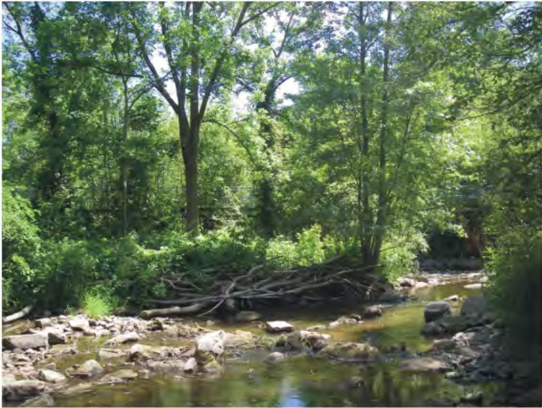
Pedestrian Bridge - Upstream side
