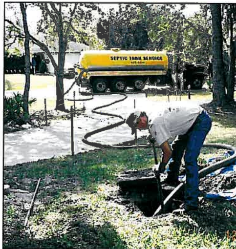
Pumping of Septic Tank (Source US EPA)
