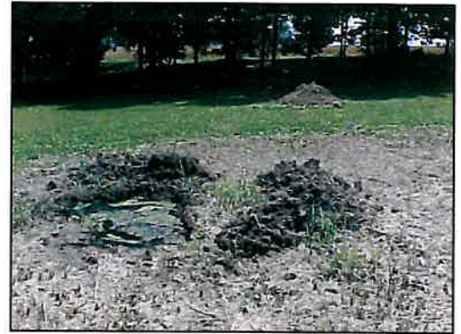
Failed Septic System (Source ORWC)
