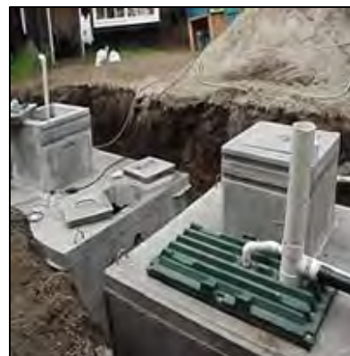
Septic Tank Replacement (Source US EPA)
