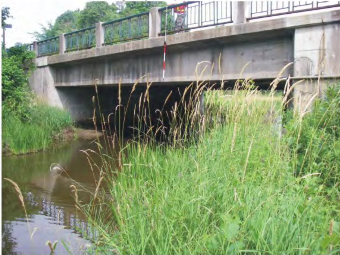
Highway 5 - Downstream side
