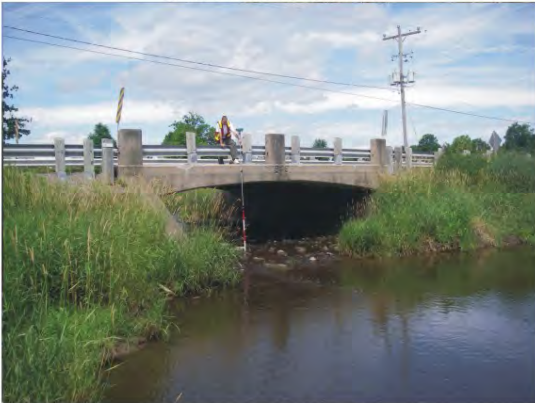
Westover Road - Downstream side
