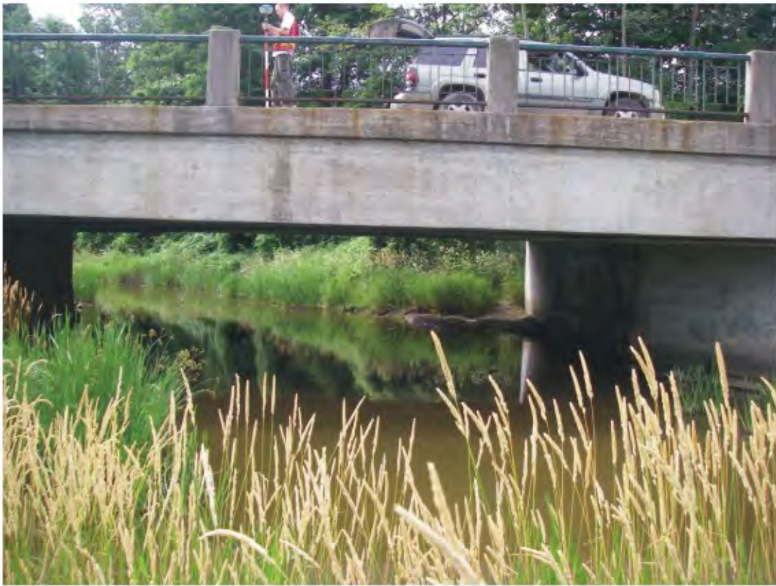
Highway 5 - Upstream side
