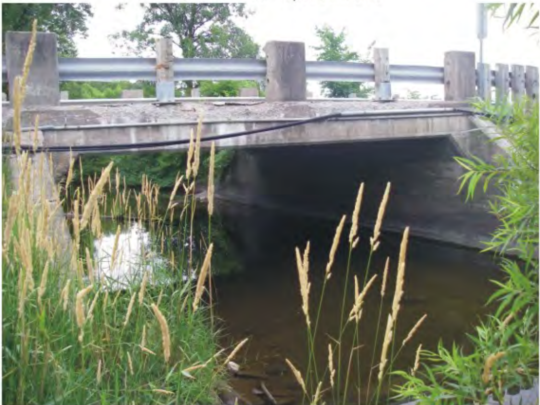
Westover Road - Downstream side
