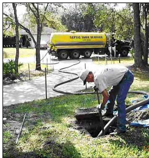
Pumping of Septic Tank (Source US EPA)
