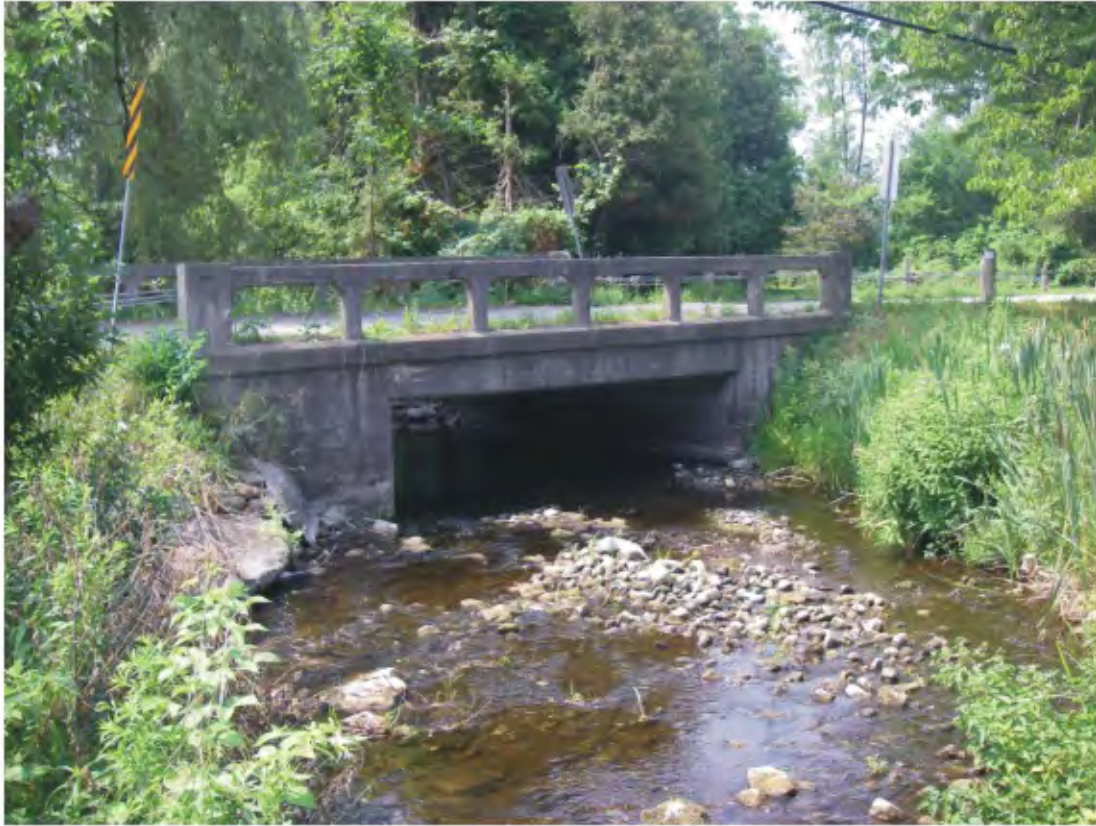
Concession 6 - Upstream side
