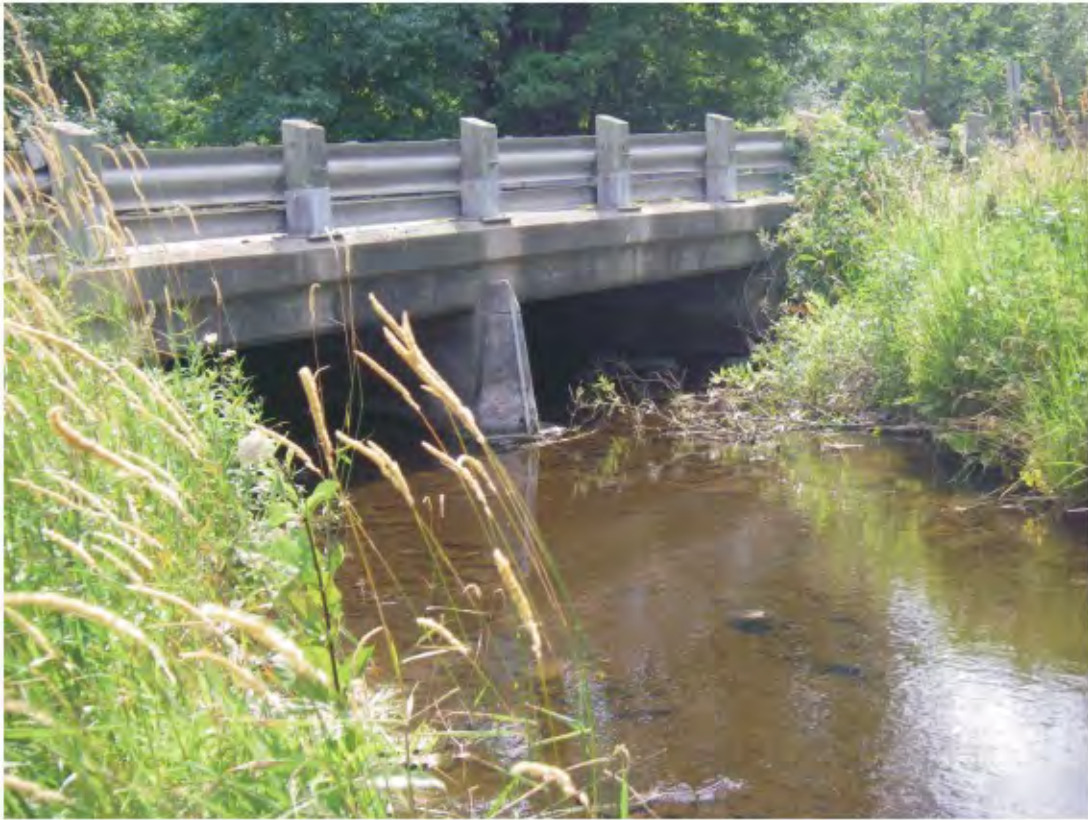
Concession 4 - Upstream side
