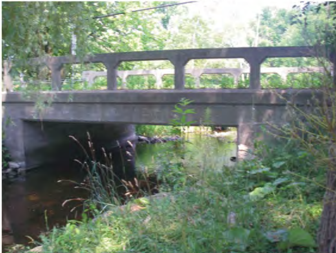
Concession 6 - Downstream side
