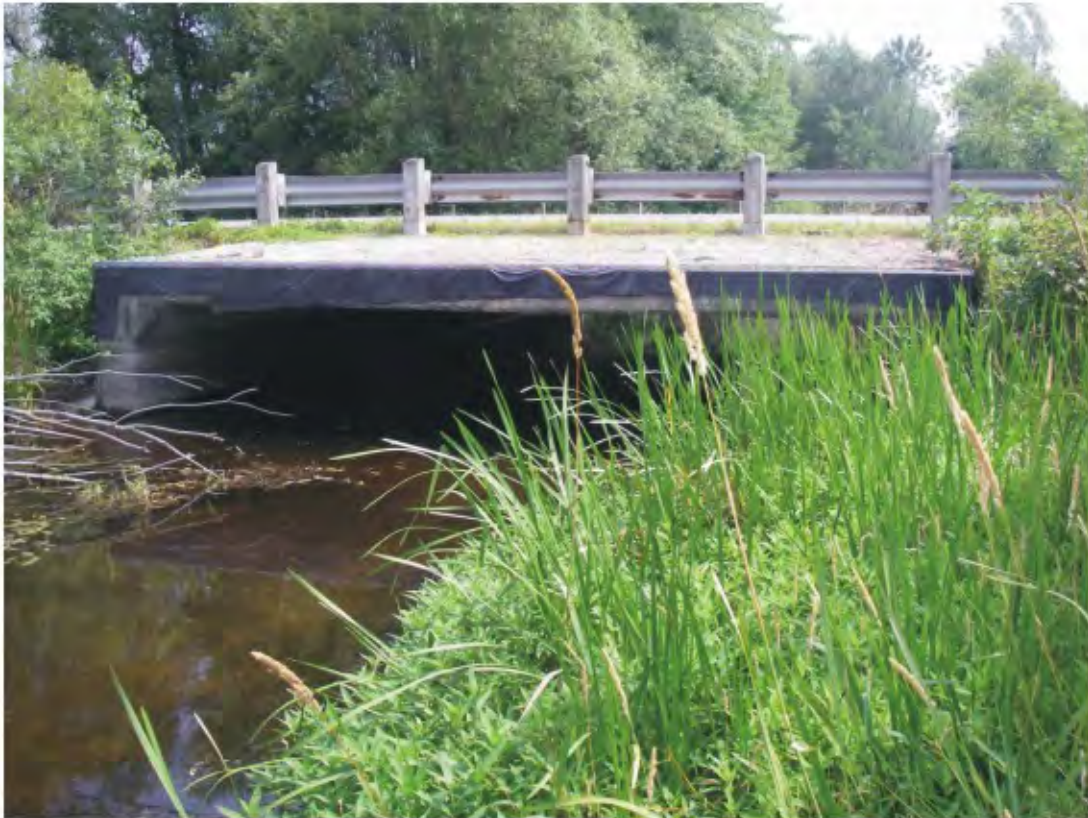
Concession 5 - Upstream side
