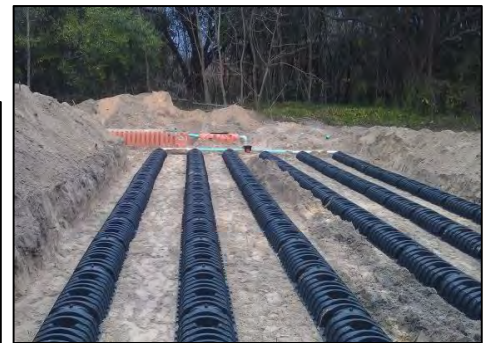
Septic Bed Replacement (Source SW Soil)
