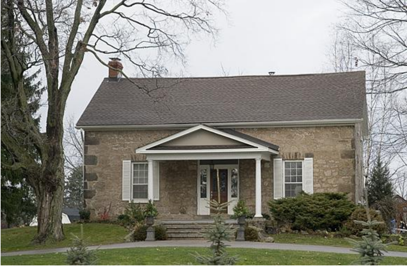
Figure 3: A closer image of the subject property. Note the location of the westerly chimney (the easterly chimney was removed sometime after 1982). The prominent, pedimented modern portico was modeled after a previous portico which was replaced sometime after 1982 (Paul Dolanjski, 2009).
