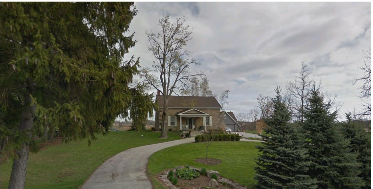
Figure 2: View of the subject property, facing northeast. Note the curvilinear driveway pattern which has been in place for many years (Google Streetview, 2017).
