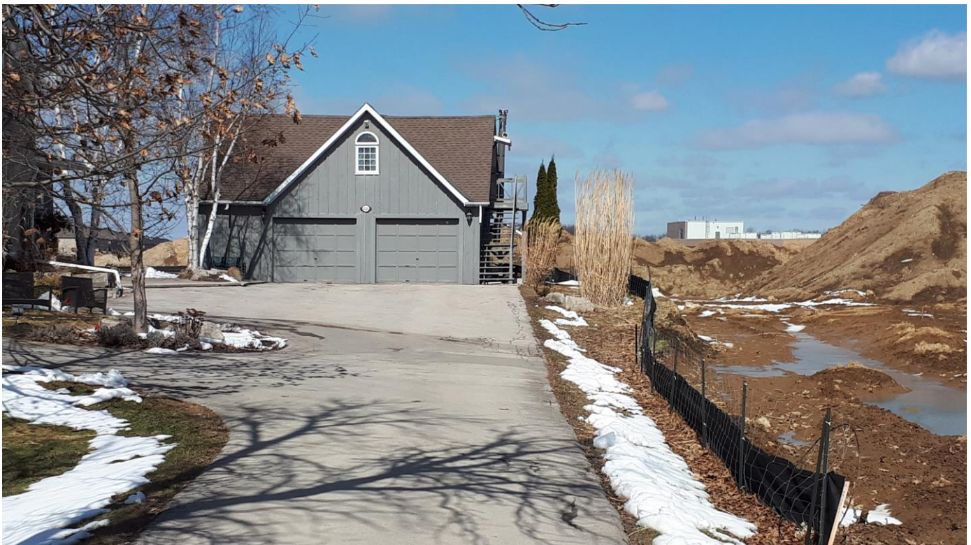
Figure 6: The modern cross-gabled two-car garage northeast of the existing dwelling (Parsons, 2018).
