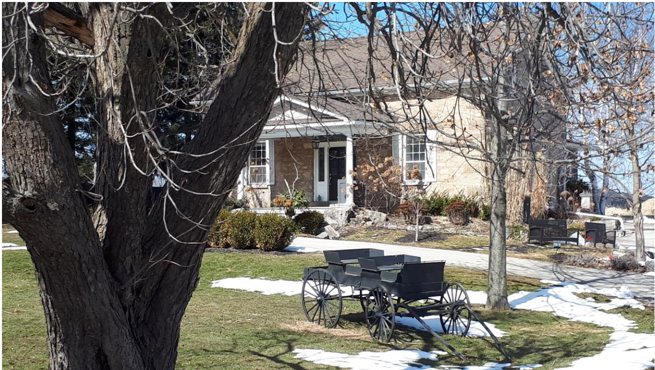
Figure 4: North-facing image of the subject property (Parsons, 2018).
