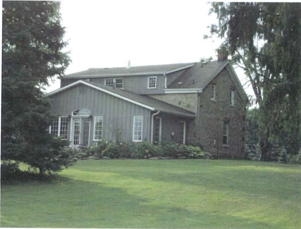
3. North elevation (direct shot obscured by trees)
