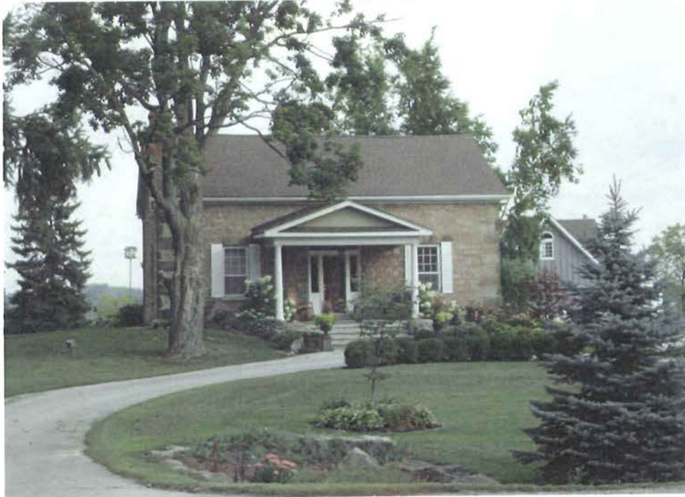
1. Lampman House south elevation
