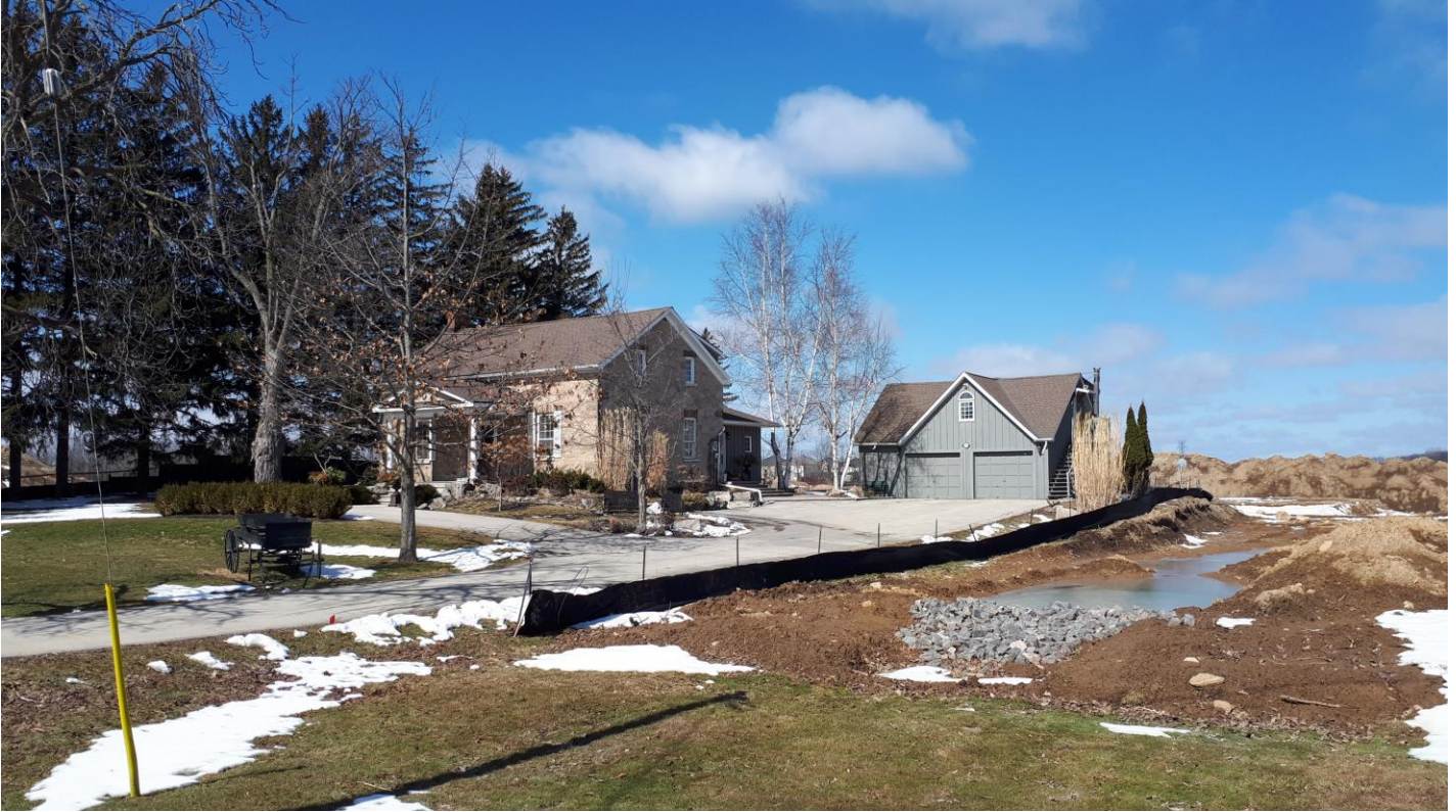
Figure 1: View of the subject property, facing northwest, from Garner Road East. Note the small parcel size and the soil disturbance on adjacent lands as part of ongoing construction activities (Parsons, 2018).
