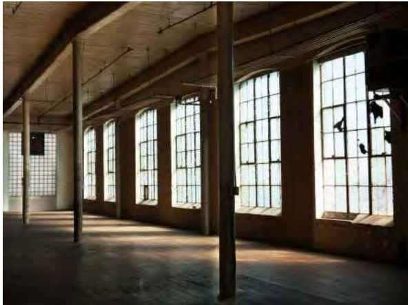
Figure 4.18 - Level 3: Large windows with 6 over 6 window panels, others with glass block infills
