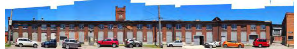
Figure 4.25 South Elevation Photo stitch
