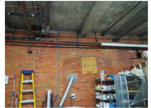
1948 addition wall, filled in window with brick
