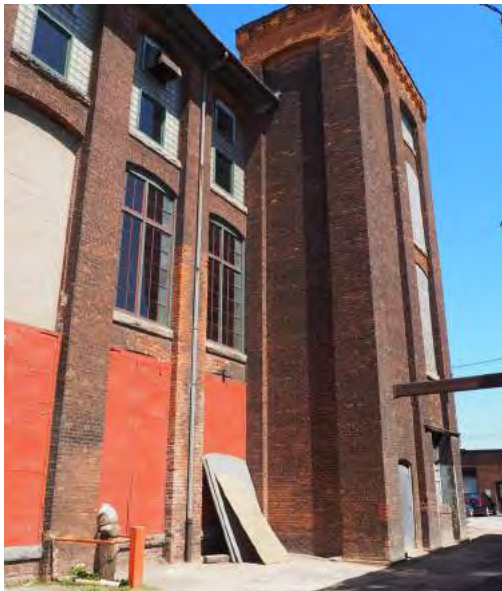
Figure 4.8 South East All original openings with ranging enclosure from plywood, glass block, and wood replacement windows.
