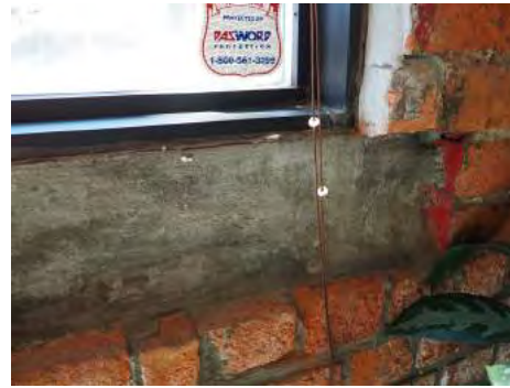
Stone lintel visible from interior window ledge
