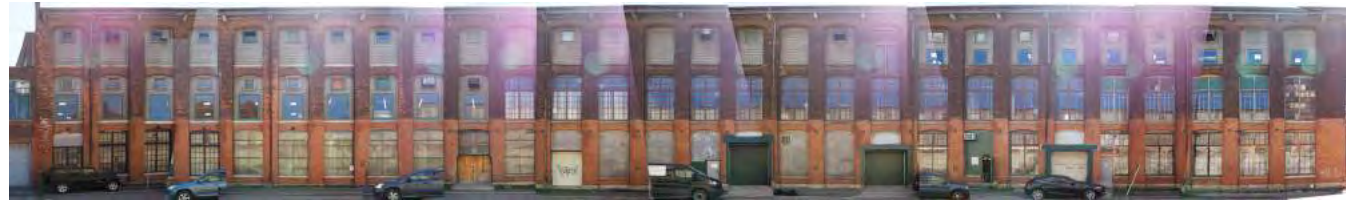
Figure 4.5 North Elevation on Biggar Avenue
