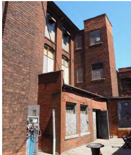
Figure 4.9 Courtyard View to south elevation from courtyard. All original openings with plywood and glass block infill with aluminum picture windows.
