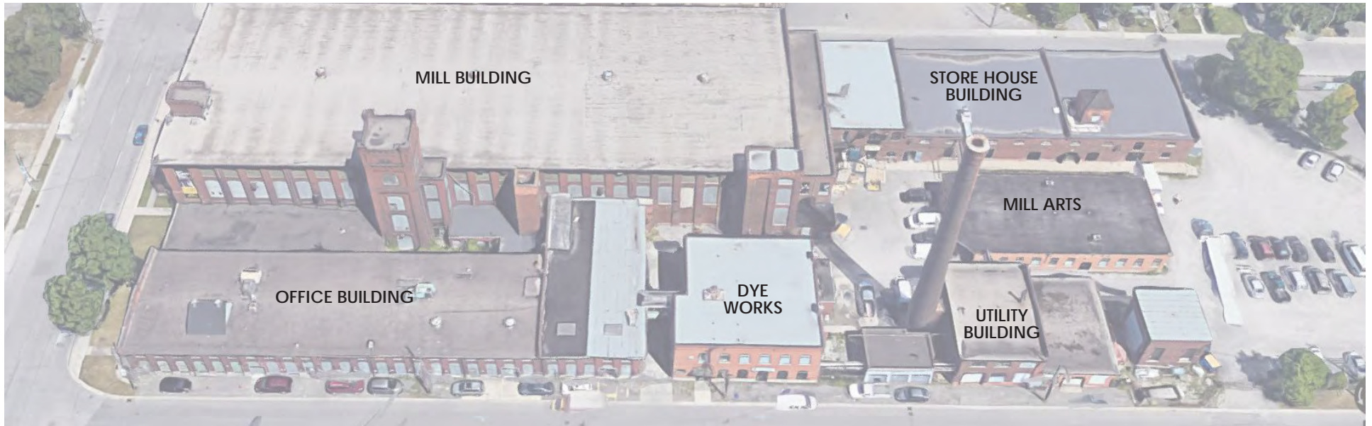
Figure 6.1 - (source: Google Maps) 270 Sherman Complex South View
