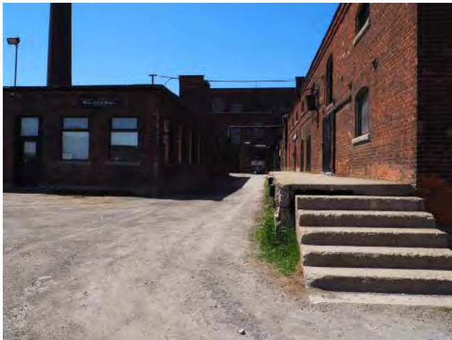
Figure 5.7 - (source: mcCallumSather) The TH&B Railway came directly into the site. The high platform indicated that the Storage Warehouse operated directly adjacent to the rail.
