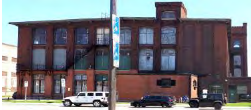
Figure 4.4 West Elevation on Sherman Avenue North
