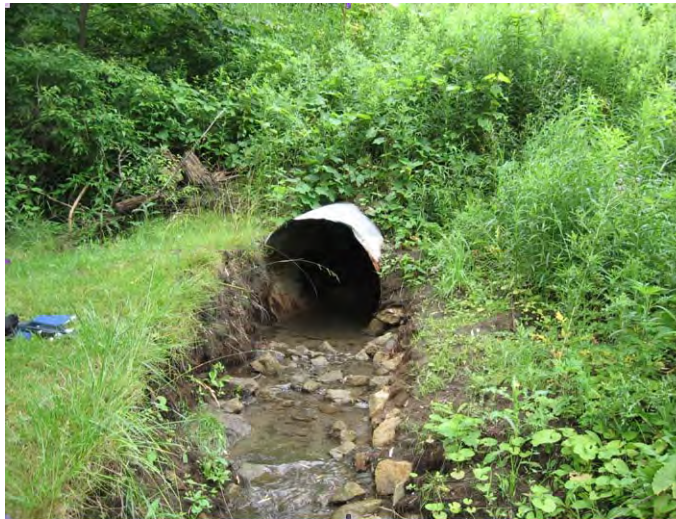
Crossing 11 – Downstream exit from the culvert
