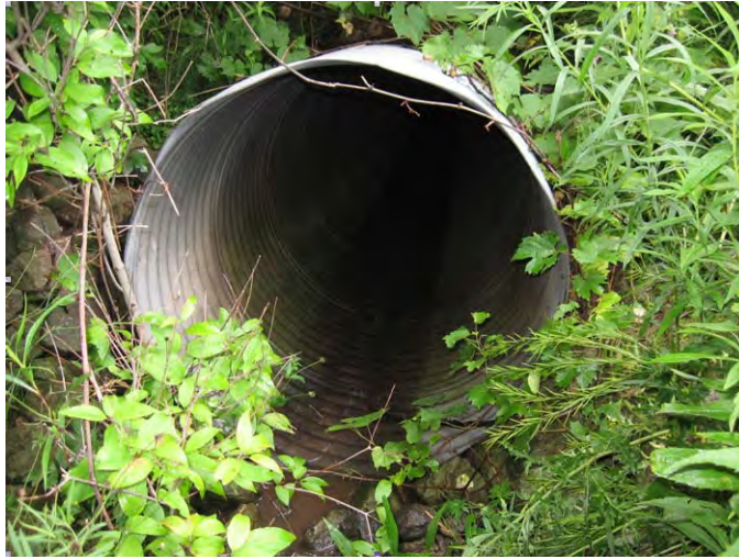
Crossing 11 – Upstream entrance to the culvert
