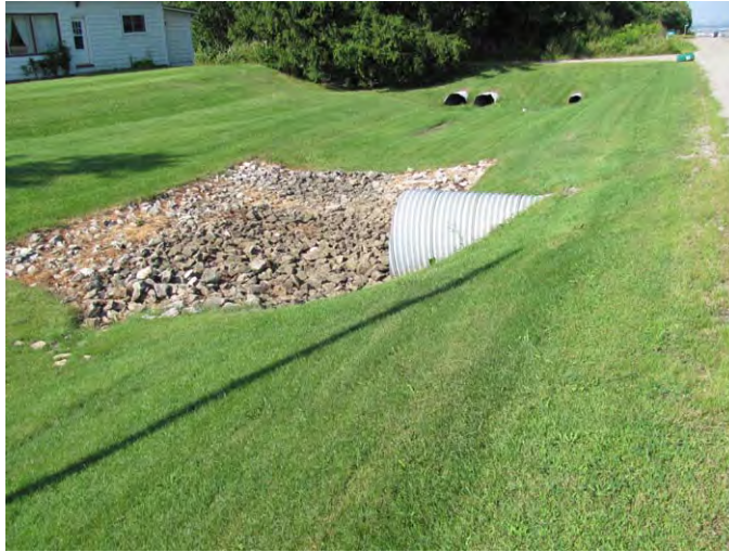
Crossing 10 – Upstream entrance to the culvert
