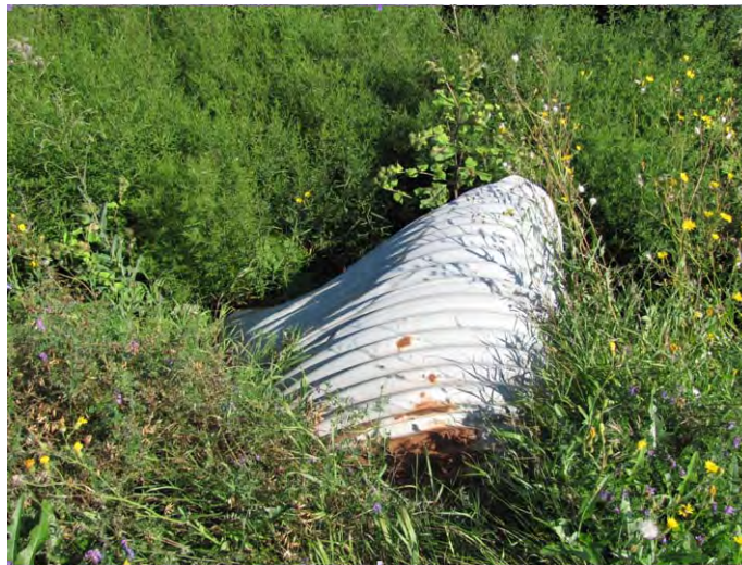
Crossing 10 – Downstream exit from the culvert
