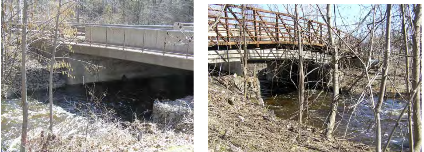
Figure 7 Existing Bridge at Parkside Dr (Left: upstream face; Right: downstream face)
