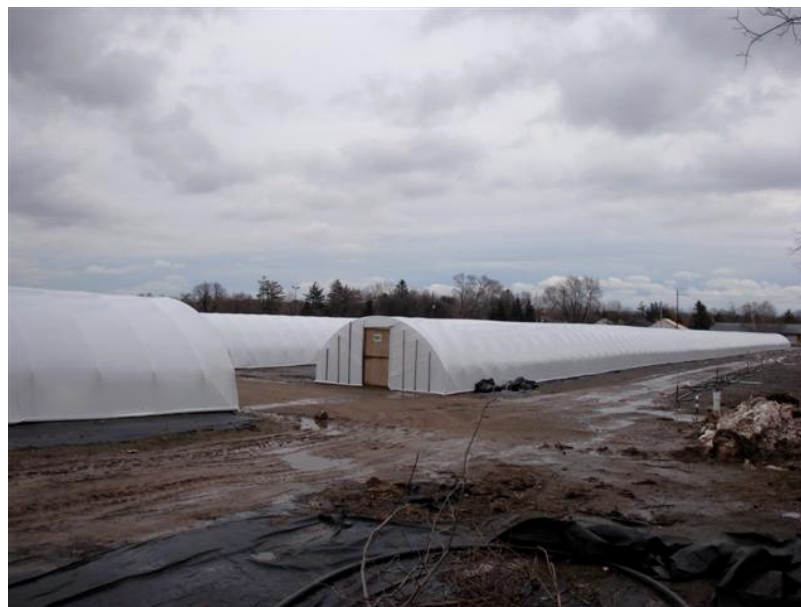
Photograph 2 – View looking southeast at typical Site conditions at the Connon Nursery property located at 383 Parkside Drive.
