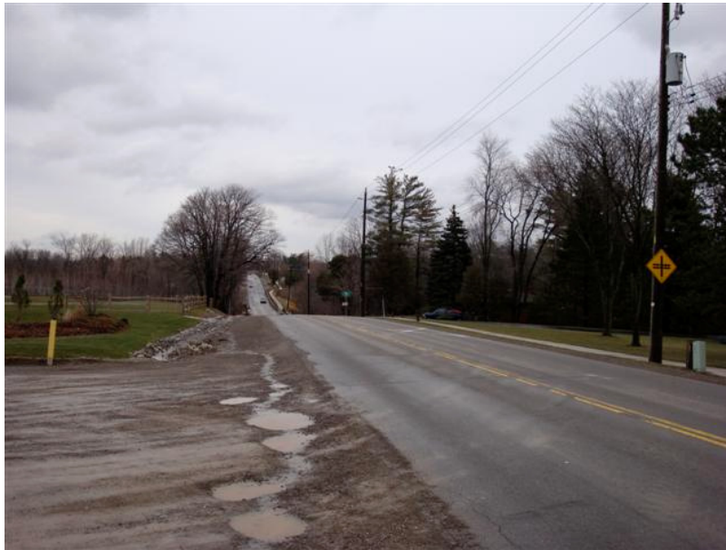
Photograph 3 – View looking west along Parkside Drive including the Grindstone Creek valley.
