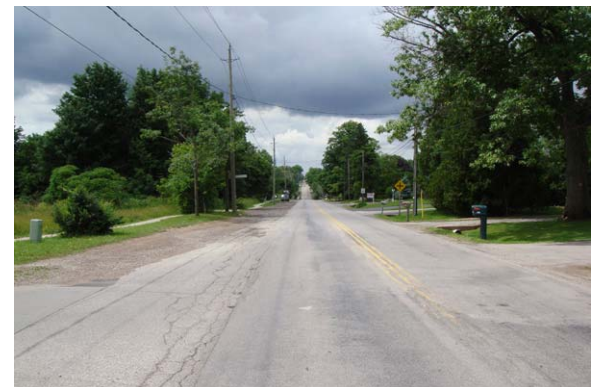
Exhibit 5-4: Parkside Drive East of Grindstone Creek Looking East (Section N4)
