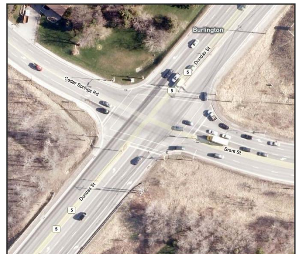
Exhibit 4-15: Existing signalized intersection at Dundas Street and Brant Street
