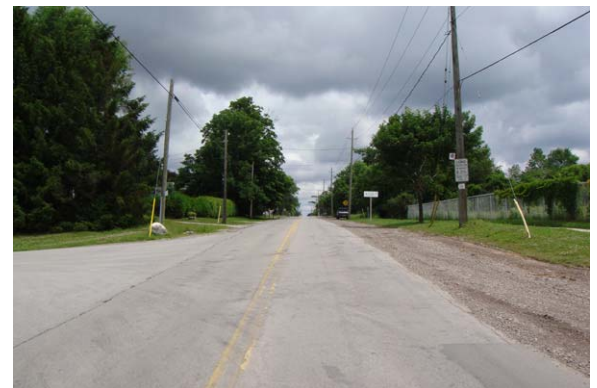
Parkside Drive East of the Grindstone Creek Looking East
