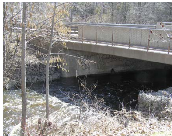
Exhibit 6-4: Existing Grindstone Creek at Parkside Drive (Upstream Face)
