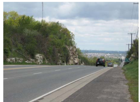
Dundas Street Escarpment Cut Area
