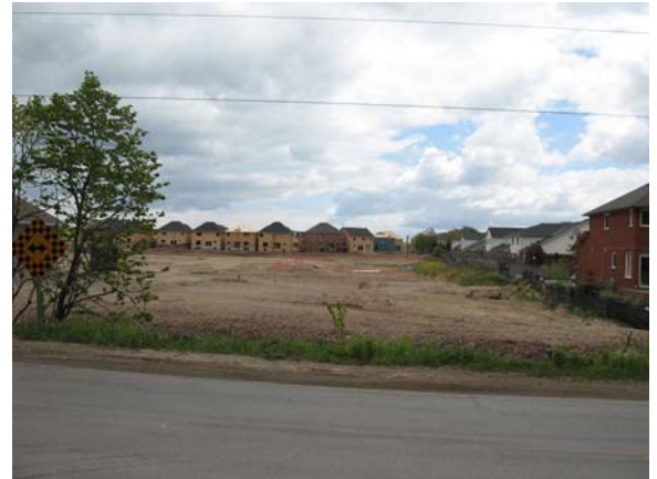
Exhibit 5-5: Initial Construction in Upcountry Development Area (Section N5)
