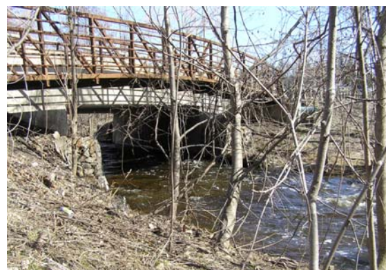
Exhibit 6-5: Existing Grindstone Creek at Parkside Drive (Downstream Face)
