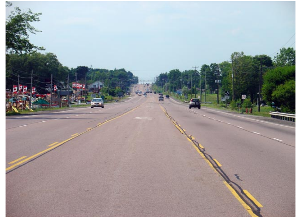
Exhibit 5-11: Highway 6 Looking North from Parkside Drive
