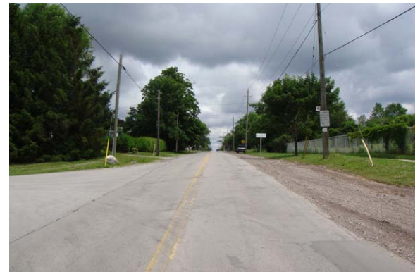
Exhibit 1-5: Parkside Drive East of the Grindstone Creek (Looking East)
