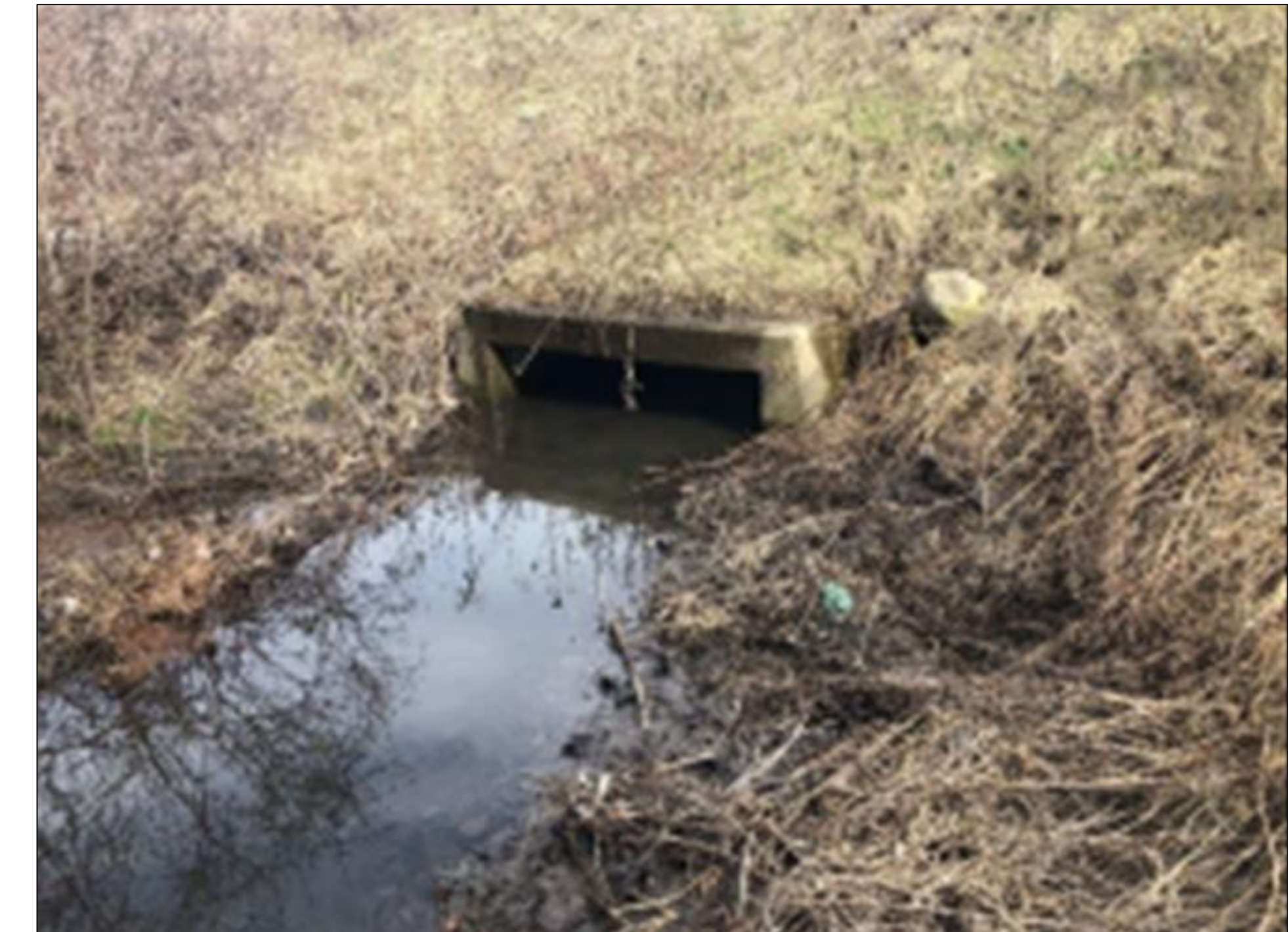
Culvert D, Ancaster Creek East Tributary, Downstream of Highway 403 (northwest)
