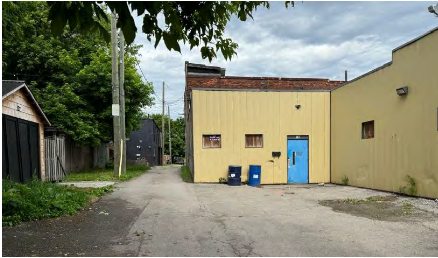
View of the alleyway from Ashley Street
