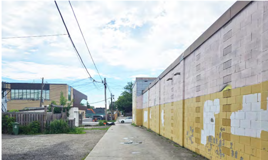
View from the alleyway looking east towards Ashley Street
