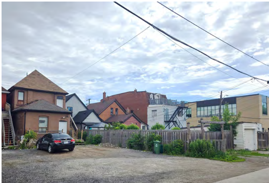
View from the alleyway looking north
