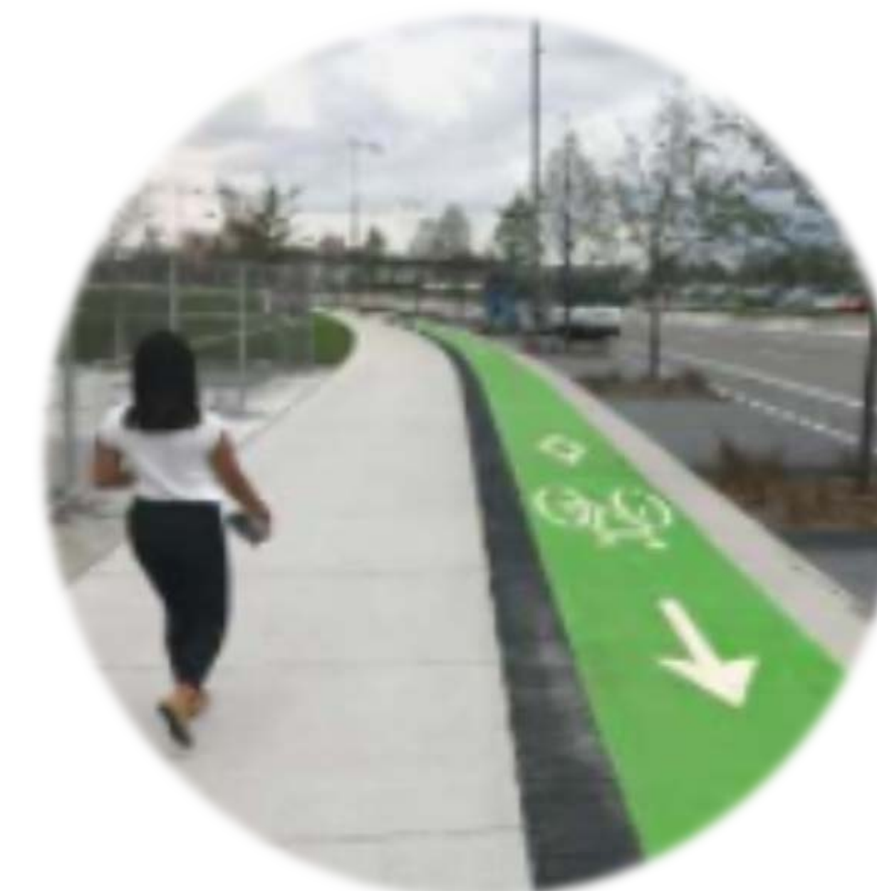
2.0m Sidewalk and 2.0m Cycle Track on Both Sides of the Road (+0.6m Buffer)
