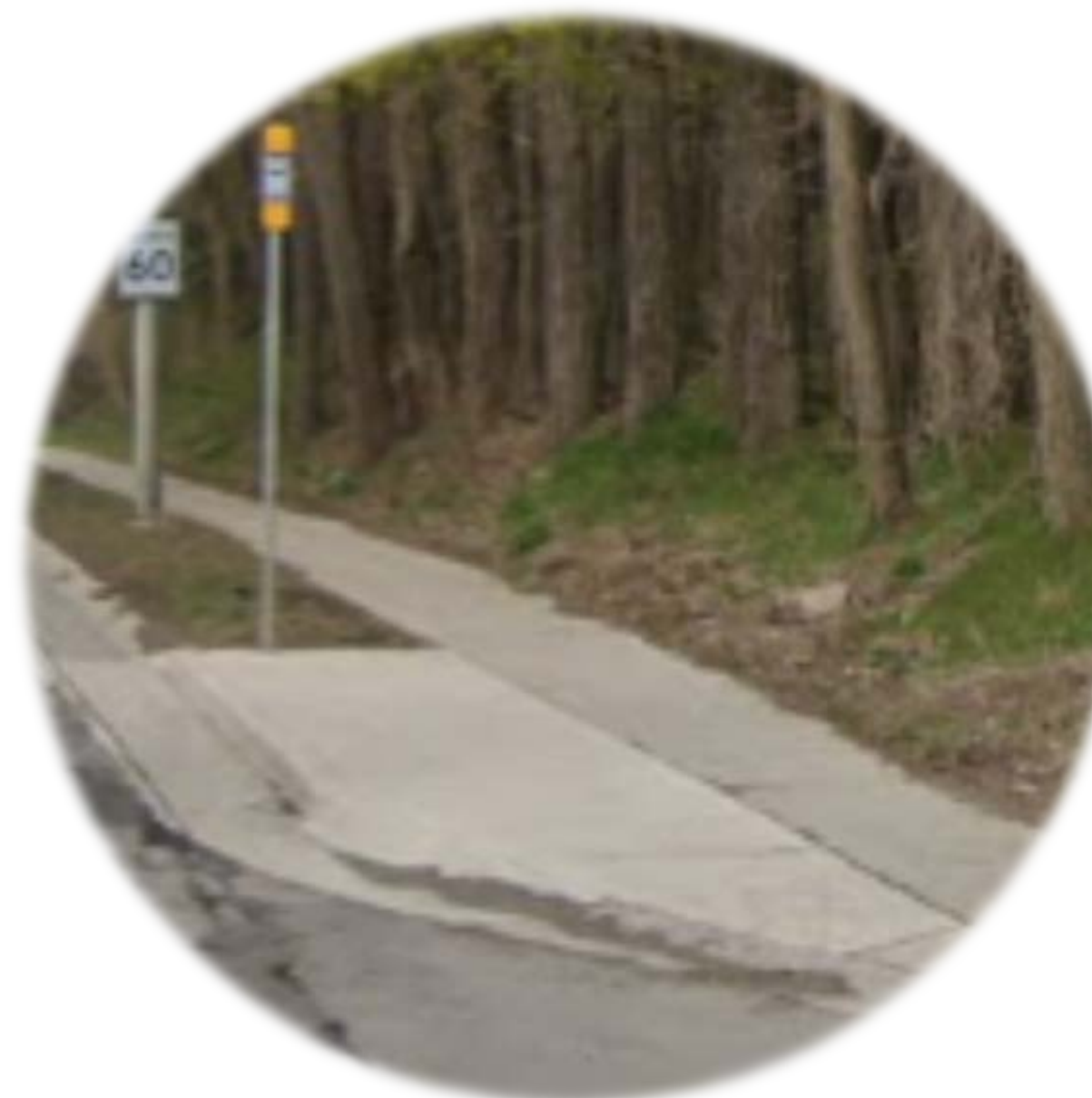
3.5m Multi-Use Pathway on North Side and 2.0m Sidewalk on South Side
