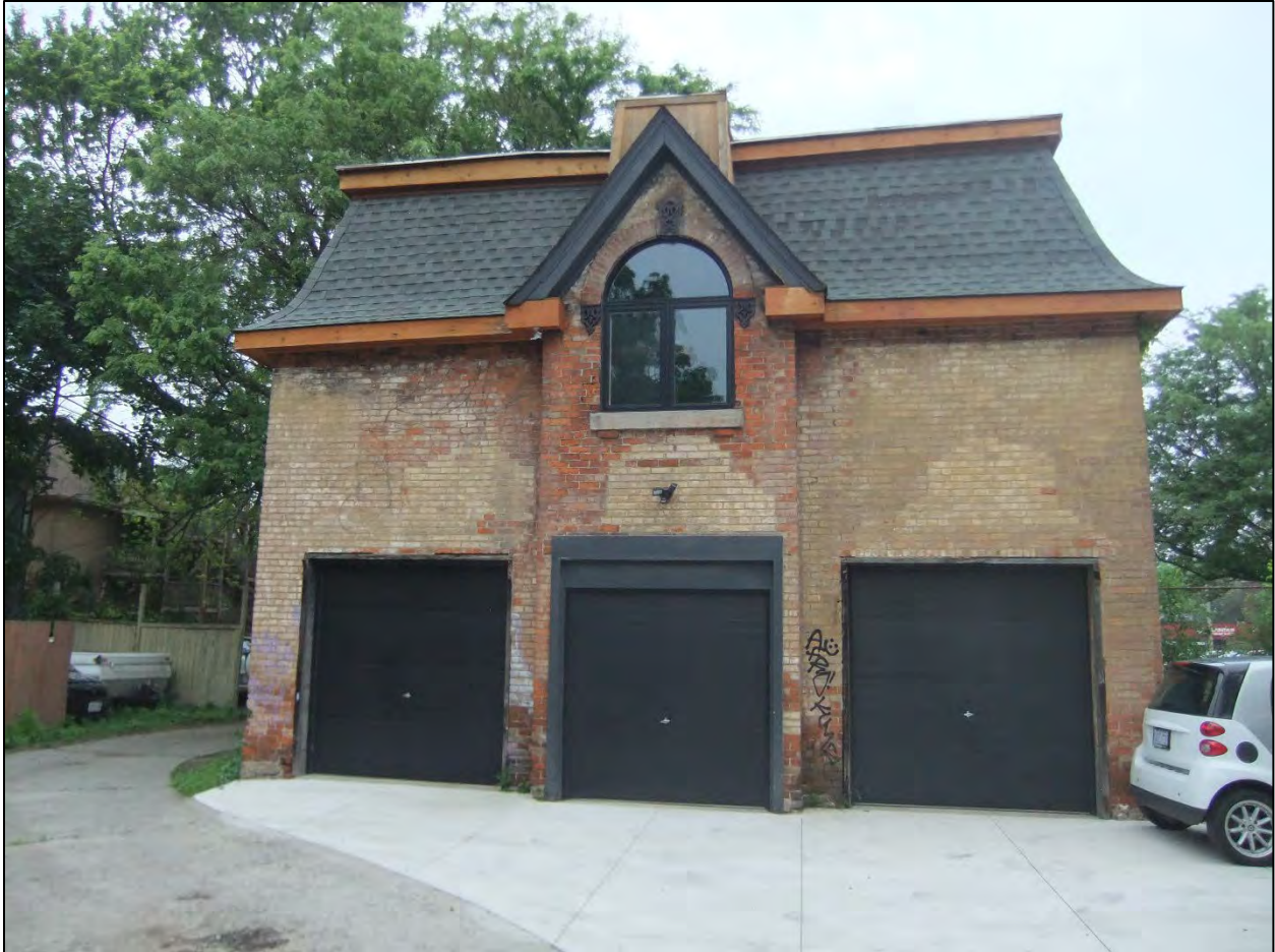
Image 4: Southern elevation looking north from the public alley. Note the varying brick colours.
