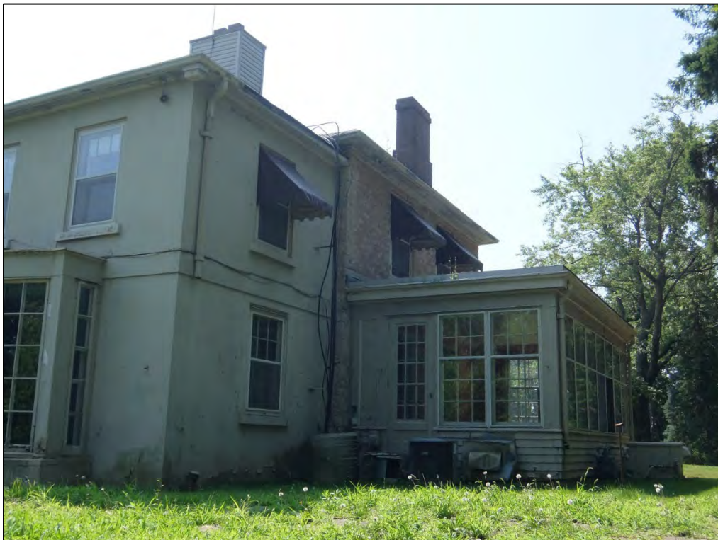
Figure 4: View of northeastern corner of property.
