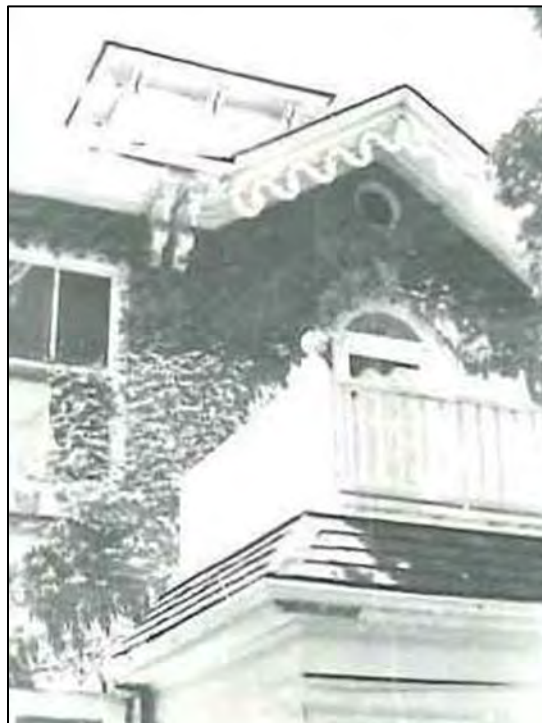
Image 24: Detail of balcony, front (east) elevation circa 1977 (Ancaster LACAC).
