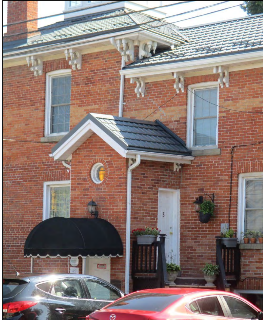
Image 15: Detail of side entrance on the north elevation.
