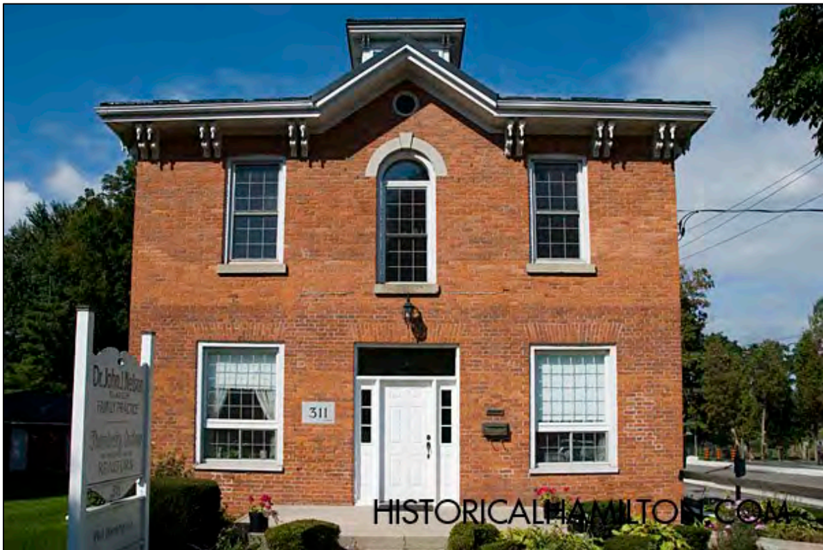
Image 18: East Elevation, c.2014 (Historical Hamilton, Retrieved September 6, 2023. https://historicalhamilton.com/area/ancaster/dr-henry-orton-house/ )
