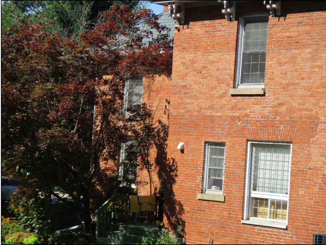
Image 13: Detail of contrasting brick masonry on side (south) elevation.
