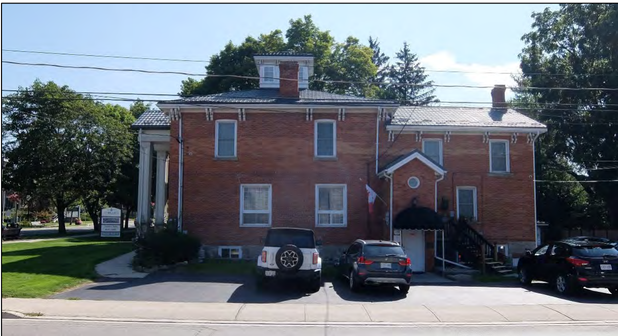
Image 4: Side (north) elevation fronting onto Sulphur Springs Road.
