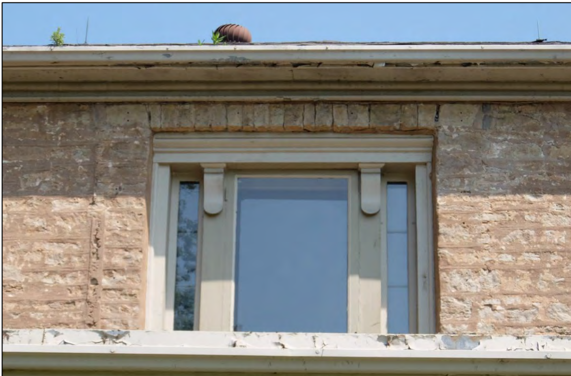
Figure 12: Detail view of Venetian window in the second storey of the south (front) elevation.
