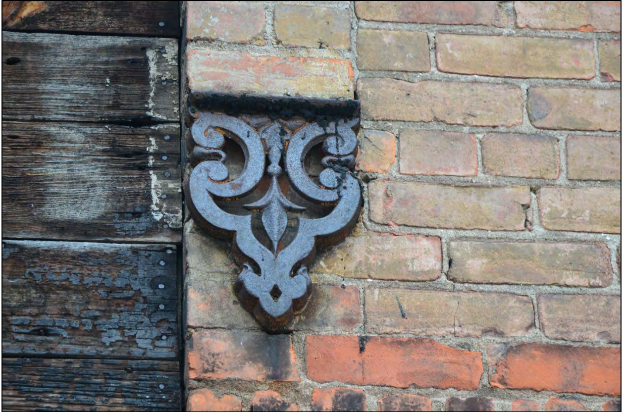
Image 9: Close-up of the cast-iron ornaments at the extremities of opening arch details. Image by Graham Carrol and Ann Gillespie, 2019.
