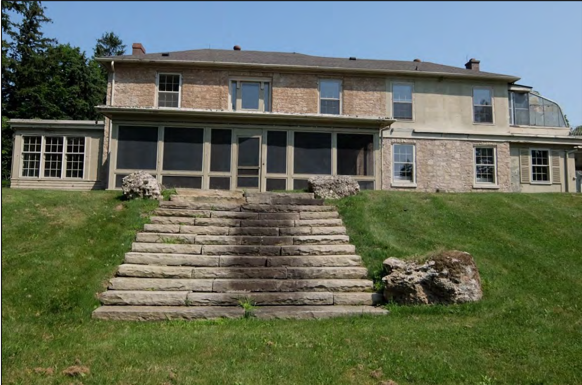
Figure 1: Front (south) elevation showing the central three-bay circa 1846 stone Neoclassical dwelling (middle), eastern stone addition (right) and one-storey western sunroom addition (left).
