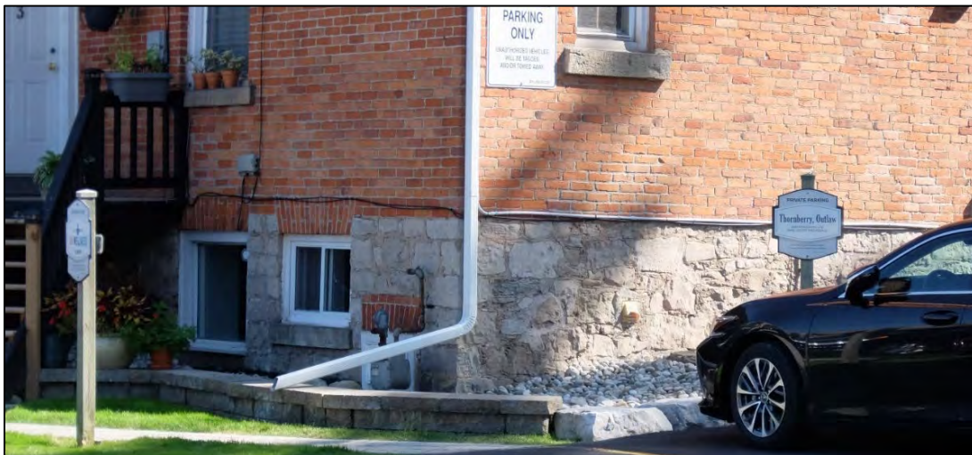
Image 16: Detail of stone foundation on the rear wing northwest corner.
