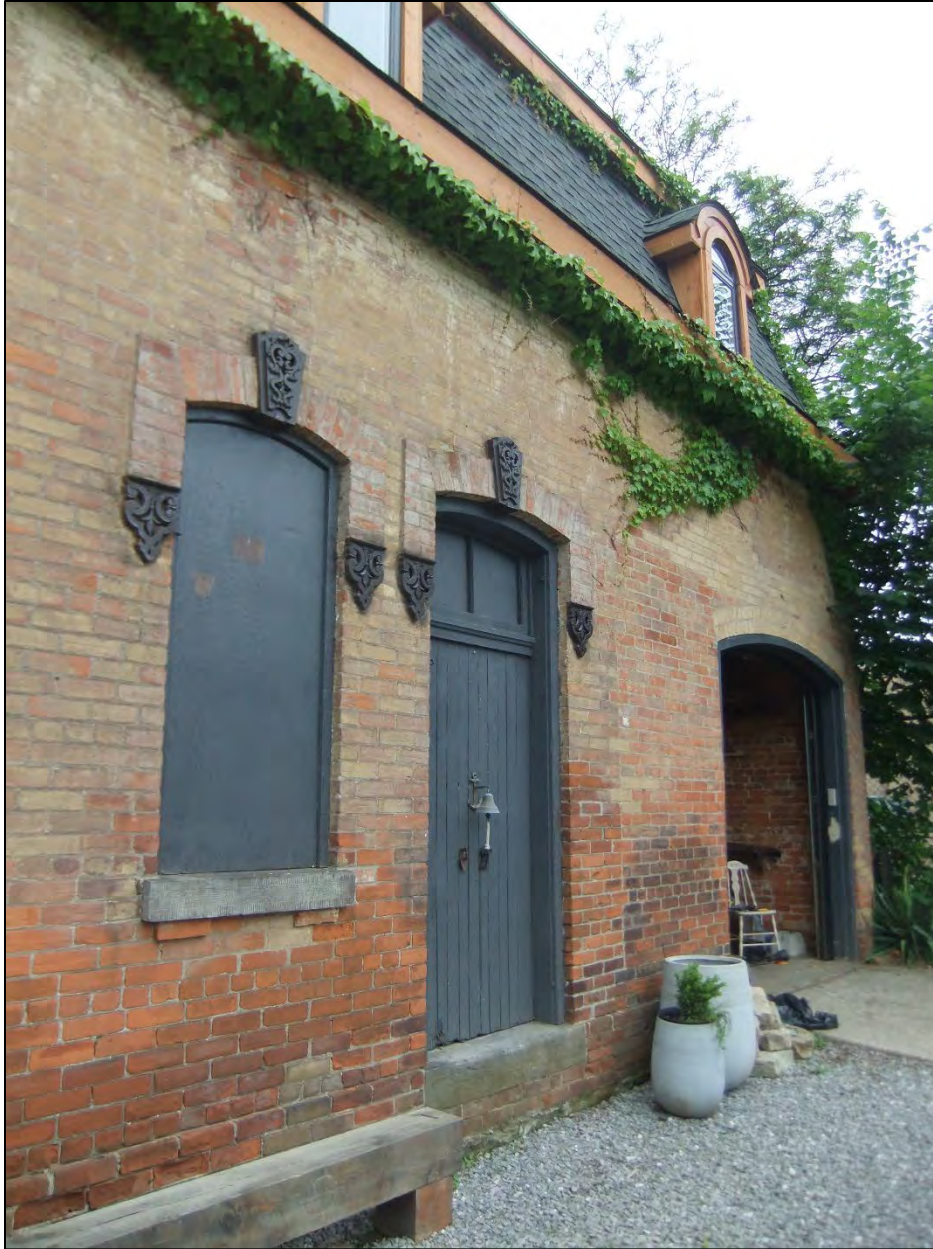
Image 2: Close-up of the eastern elevation, showing the openings and brick in greater detail.
