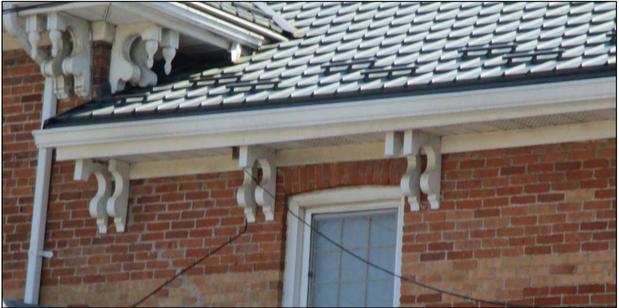
Image 9: Detail of brackets on the north elevation at the intersection of the main building and the rear wing.
