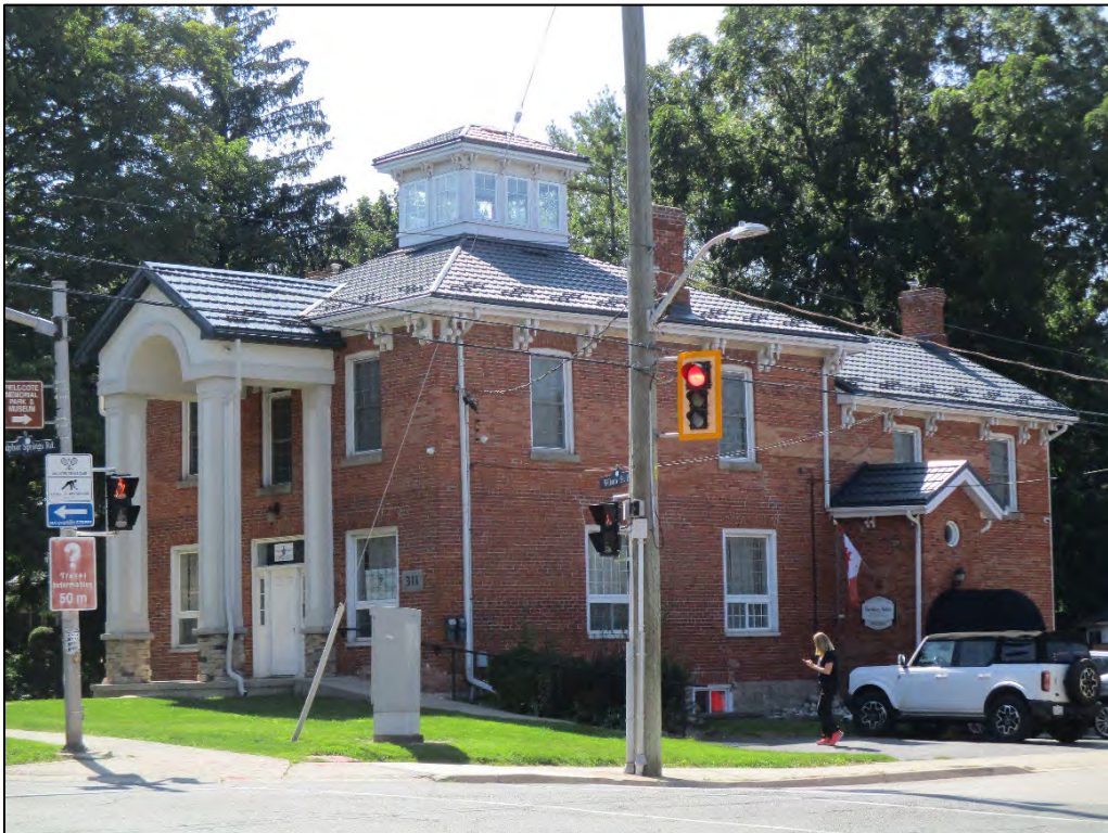
Image 2: Orton House, looking southwest from the intersection of Wilson Street East and Sulphur Springs Road.
