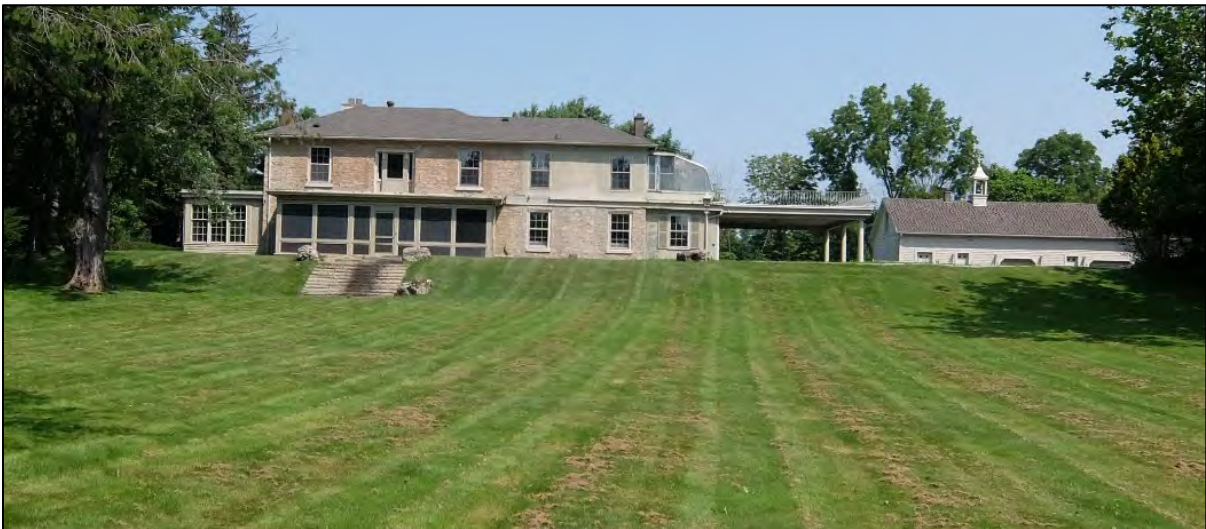
Figure 2: View of south (front) elevation of the building, showing the original circa 1846 Neoclassical residential building to the left, side additions with covered drive and detached accessory building.
