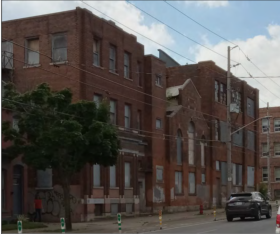
Figure 11: North elevation of the property looking west along Cannon Street East, including 136 Cannon Street East (Structure 5, left), eastern portion of 140-146 Mary Street (Structure 4, middle) and the western portion of 140-146 Mary Street (Structure 4, right).
