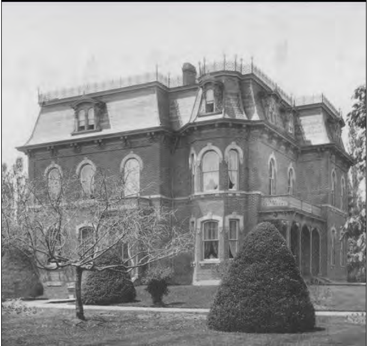
Image 15: Historic image of the original Eastcourt Estate residence. Note the cast iron ornaments around the first storey window openings which match those of the surviving Carriage House.
