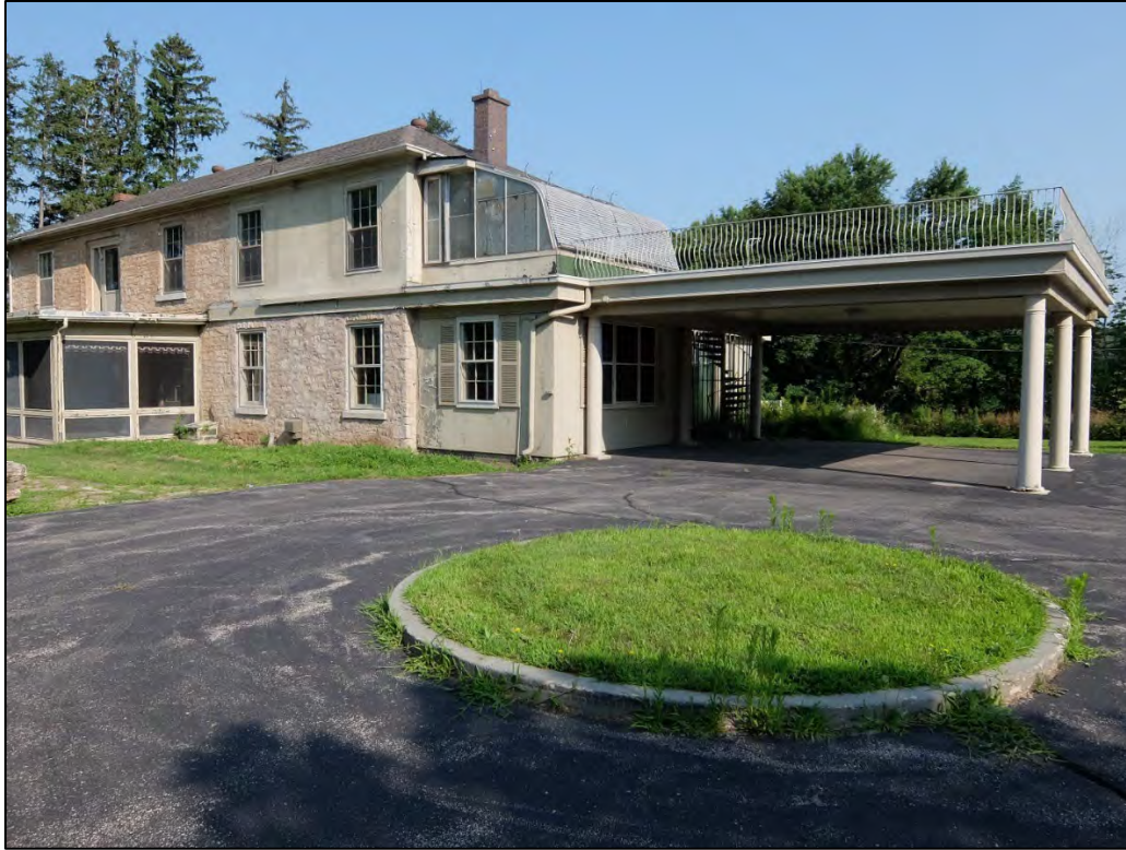
Figure 7: View of southwestern elevation showing side additions.
