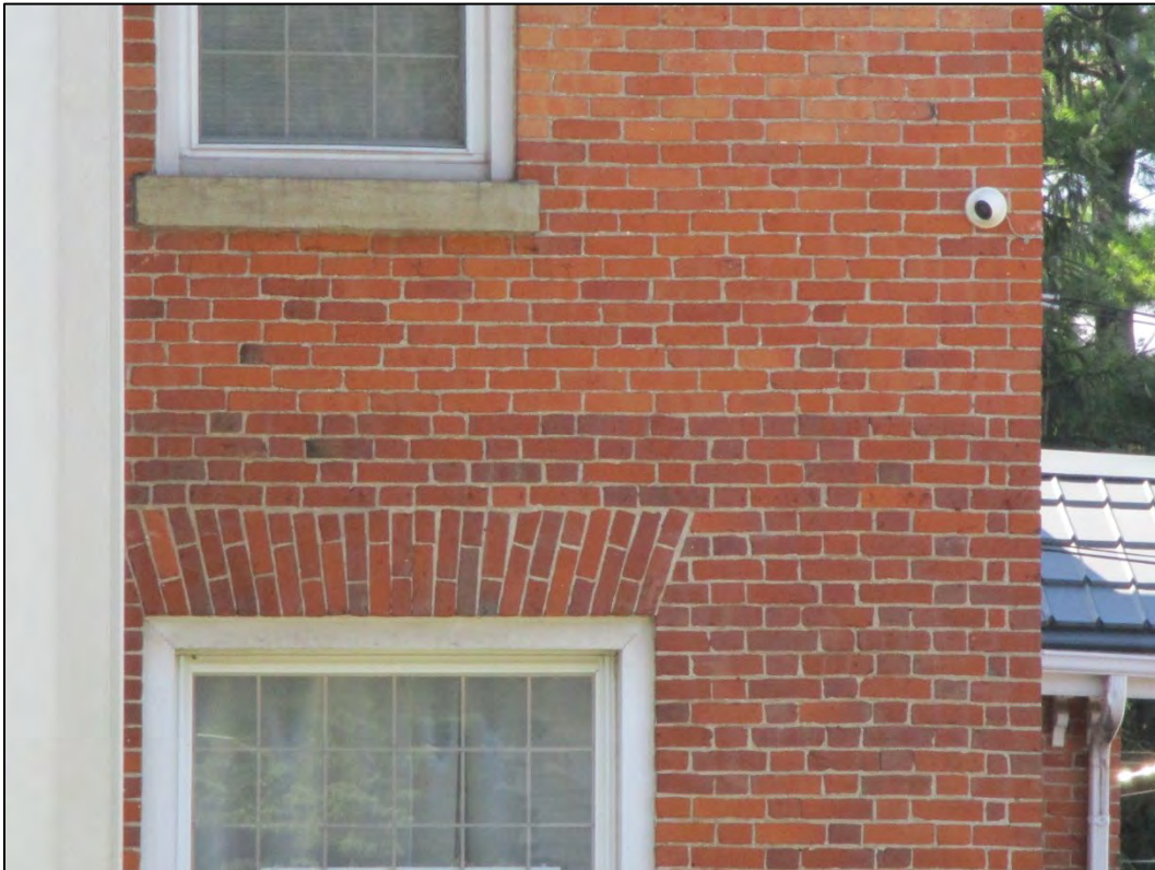
Image 12: Detail of contrasting brick masonry on front (east) elevation.
