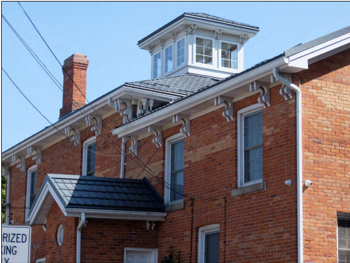
Image 6: Detail of roofline on side (north) elevation, showing brackets and belvedere.
