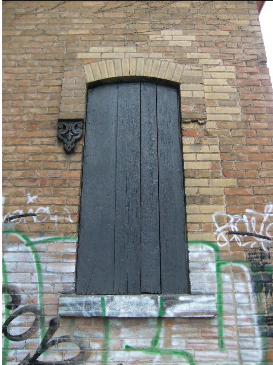
Image 7: Close-up of a window opening on the western elevation. Note the different colour bricks and missing cast-iron elements, indicating that the opening was repaired in the past.
