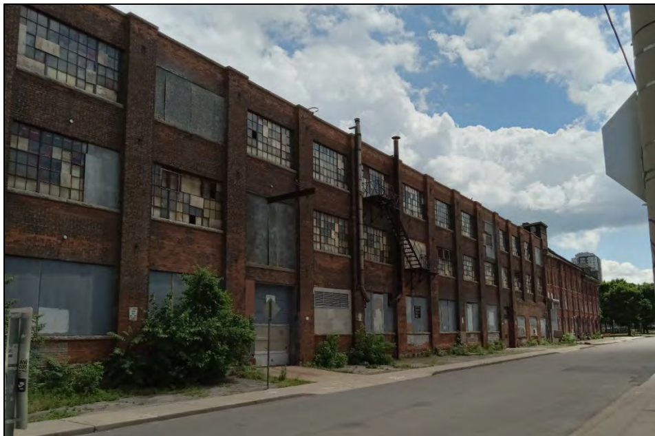
Figure 12: West elevation of the property looking south along Mary Street, including 140-146 Mary Street (Structure 4, left), 130 Mary Street (Structure 1, middle right) and 122 Mary Street (Structure 2, far right).
