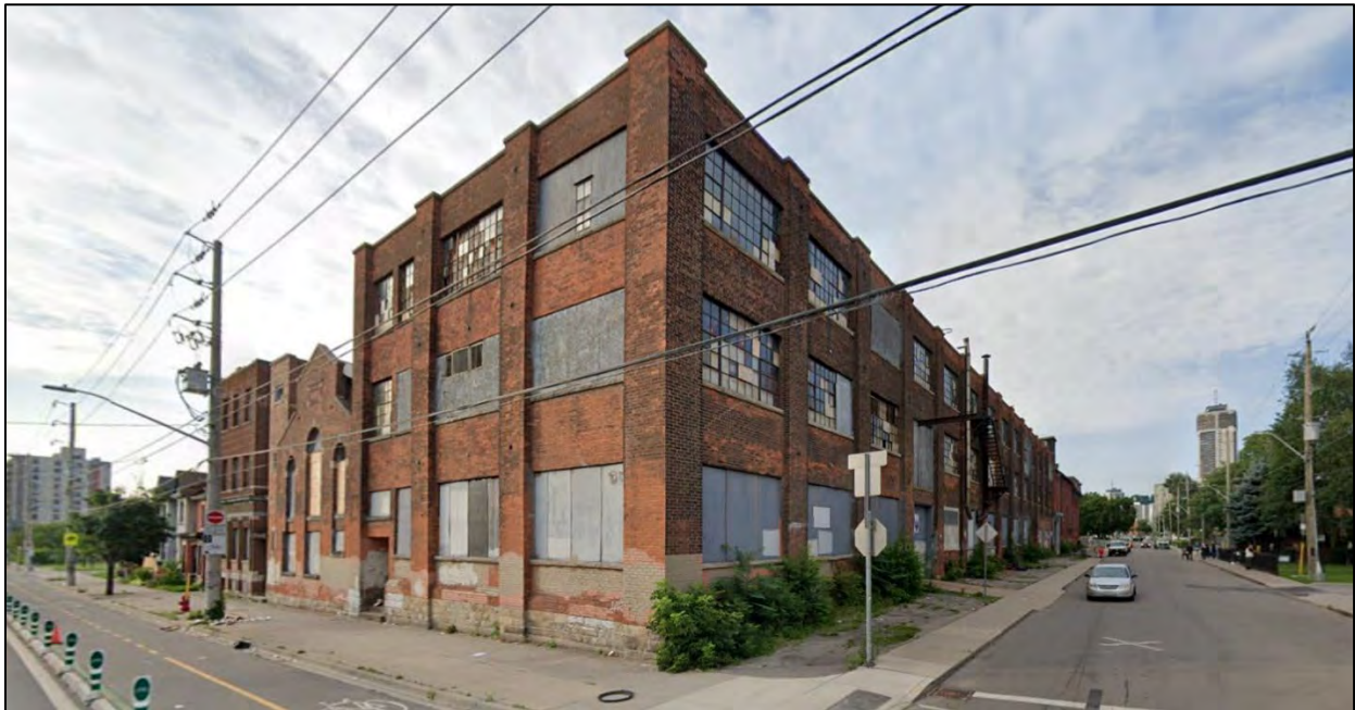
Figure 10: Northwestern corner of the property at the intersection of Cannon Street East and Mary Street. (Google Maps)
