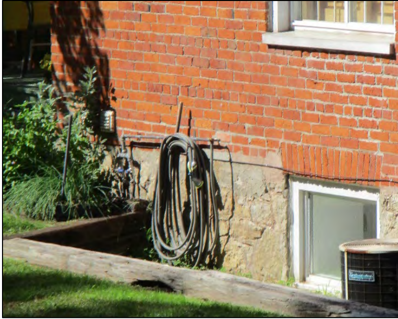
Image 17: Detail of stone foundation on south elevation.
