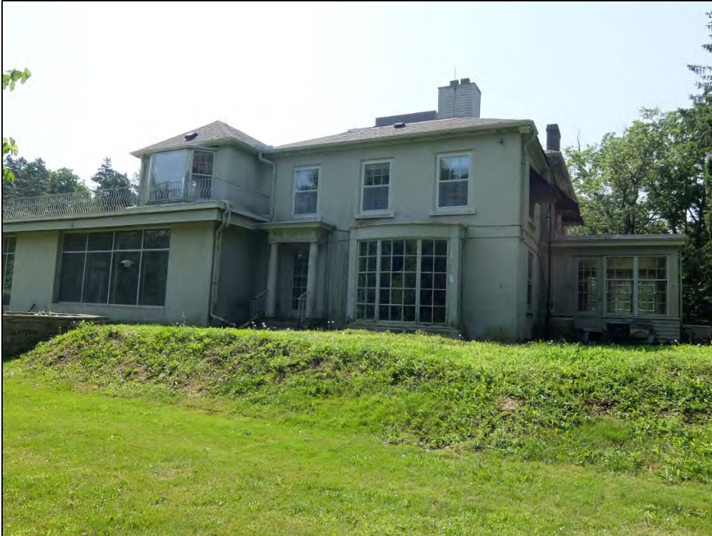
Figure 5: View of northern (rear) elevation.
