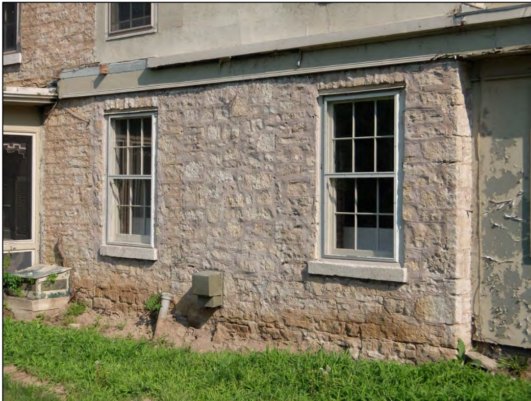
Figure 10: Detail view of the first storey of the circa 1860 eastern side addition.
