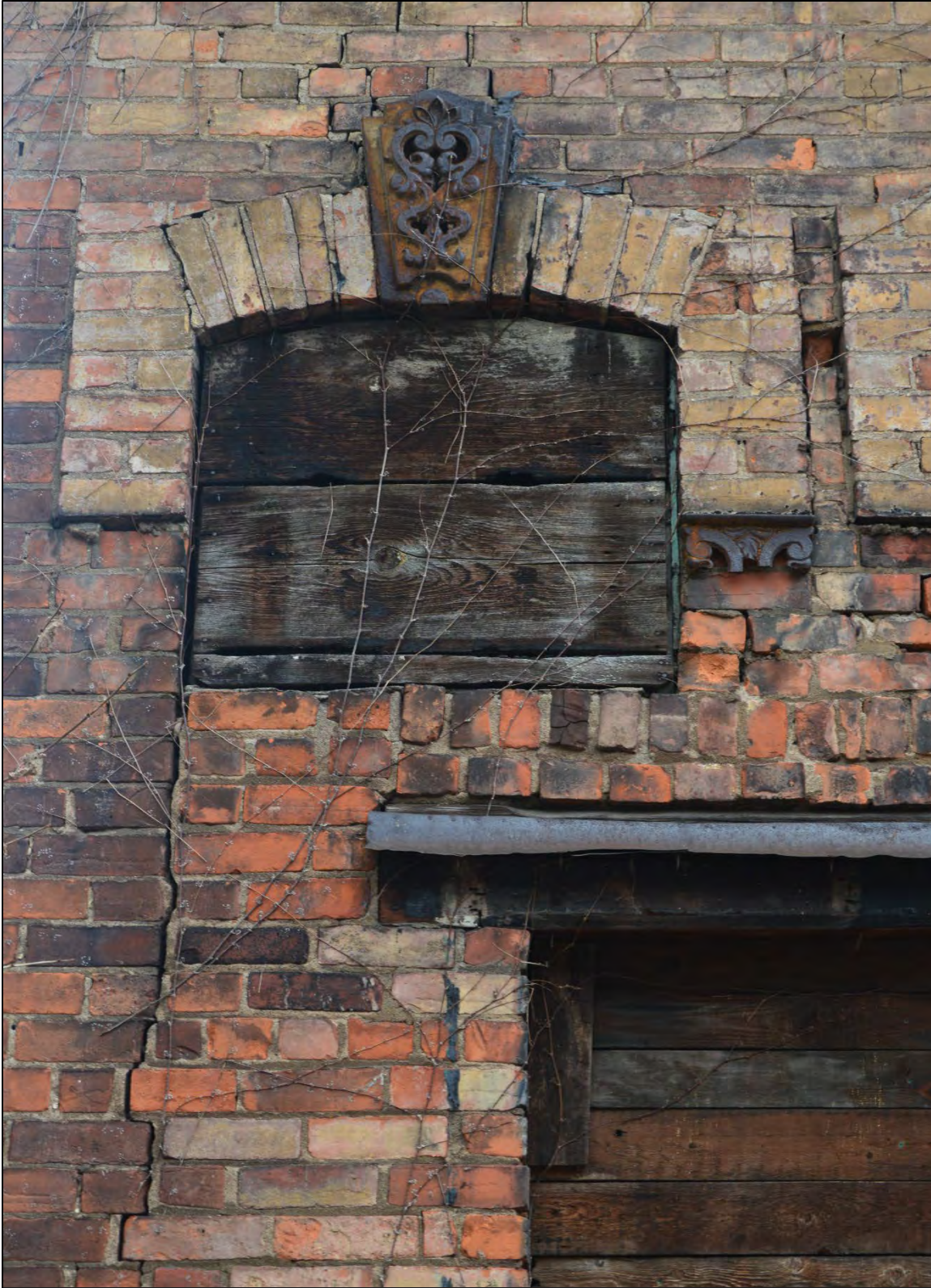
Image 10: Close-up of the truncated original openings on the western elevation. Image by Graham Carrol and Ann Gillespie, 2019.
