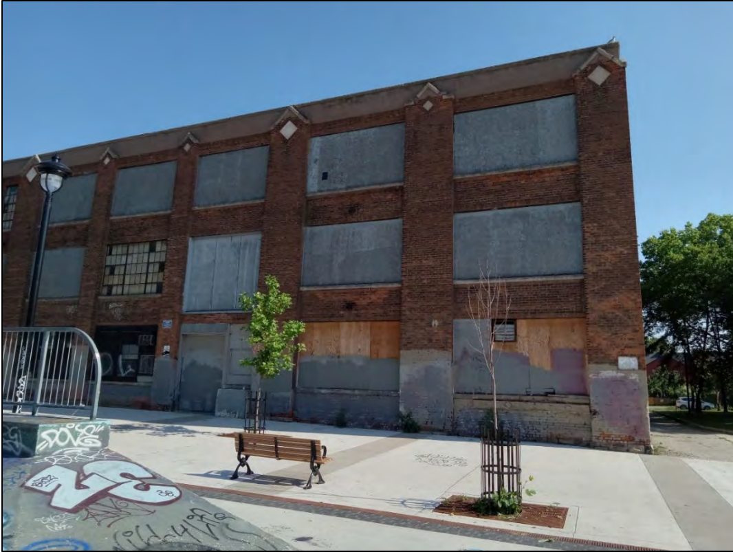
Figure 5: View of the south façade of 11 Kelly Street (Structure 3), built circa 1910.
