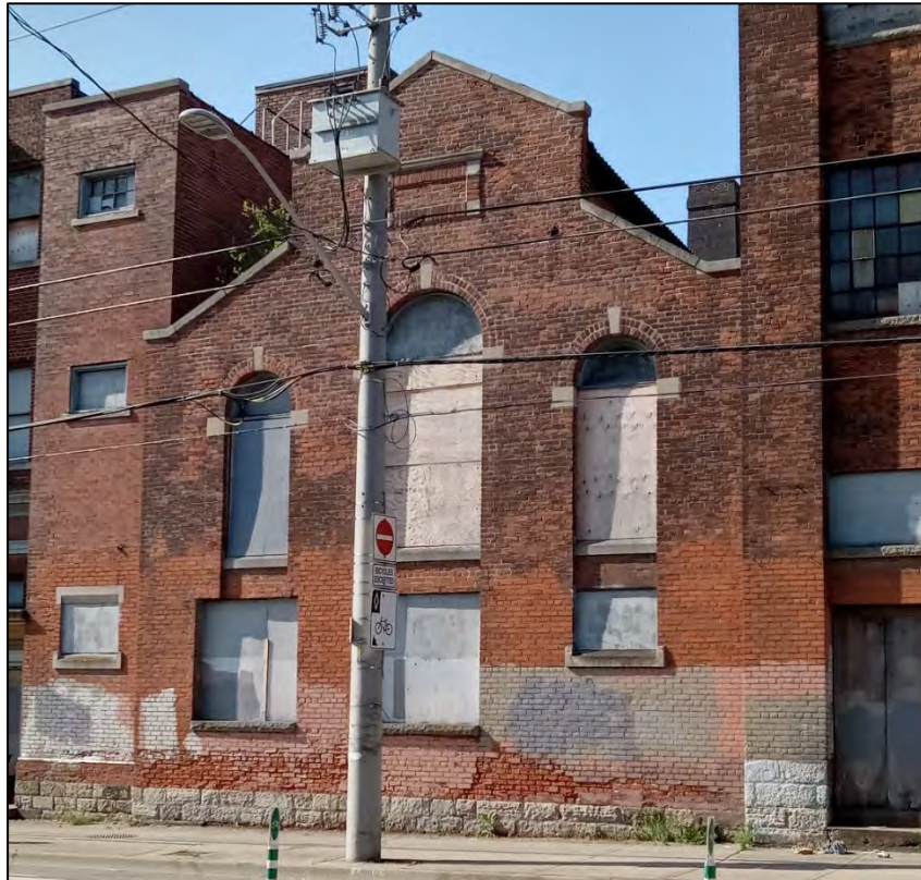
Figure 8: View of the north façade of the eastern portion of 140-146 Mary Street (Structure 4) facing onto Cannon Street East, built circa 1927.
